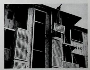
Detail of the light-weight concrete components which were used to make the latticework of the balconies of the Cité de la Muette, both for the tower blocks and the comb-layout buildings.
