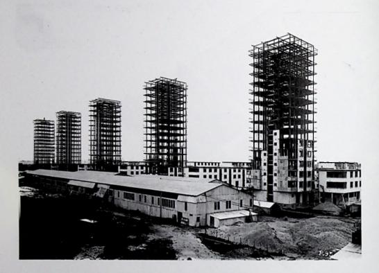
The layout of the buildings on the plot allowed for the concrete panels to be made on-site, taking advantage of the empty spaces between the blocks and meaning no transportation was required. The manufacturing facilities were set up on the north-west angle and the components were moved on rails. The buildings were erected following an order from west to east.
