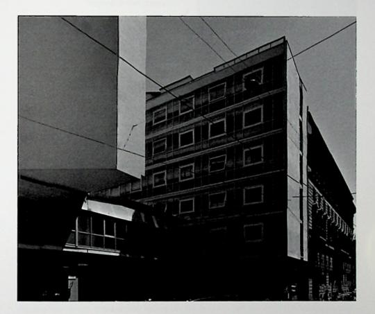
The whole north facade of Block D is glazed and its layout contains fixed and opening elements, tilting sashes with a horizontal axis at the centre. The entire facade is unprotected glazing as it faces north. This material breaks with the massiveness of the facades in the historic centre and it is only the balance in the layout of the openings which preserves the rhythm of the surrounding buildings.
