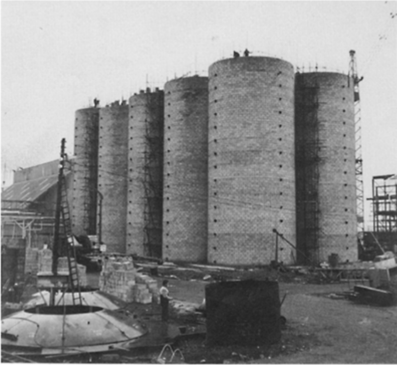
Figure 21 20000 ton prestressed concrete rock phosphate silo (before steelwork and cladding fixed)
