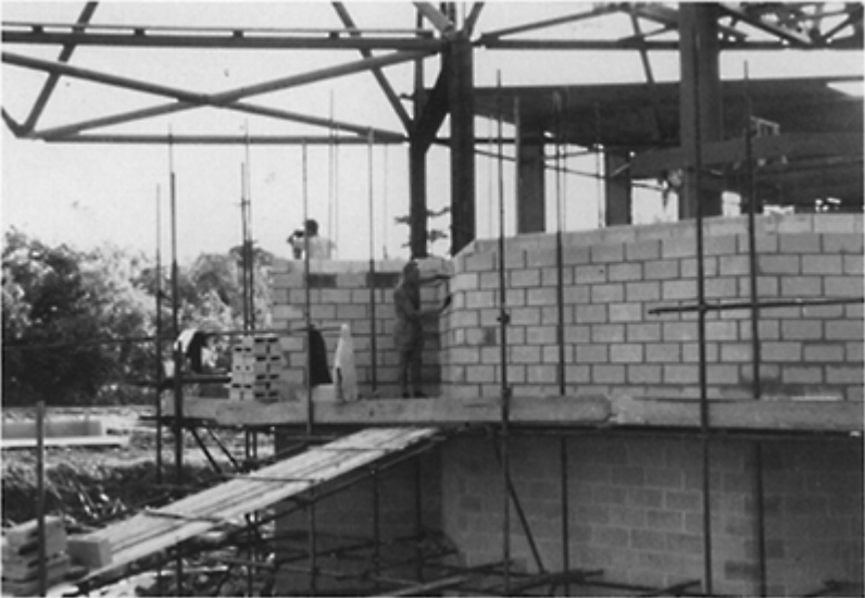
Figure 10 Reinforced chevron walls of Beaulieu Motor Museum
