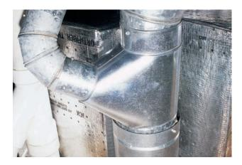
Transition piece used in the heating and cooling system of a building
