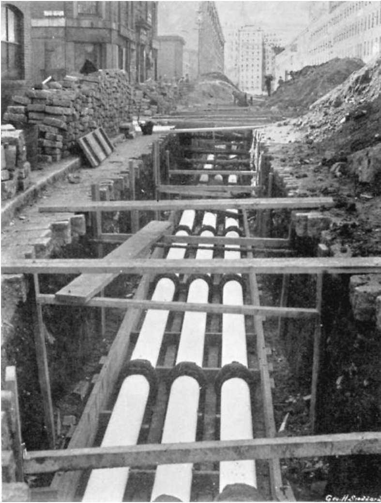
FIGURE 2.9. The brine conduit being laid underground in the market district. "Boston's Cold Corner," Ice and Refrigeration 9:6 (December 1895): 386–87.
