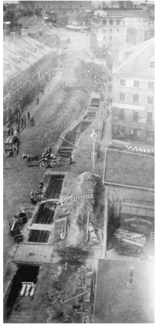
FIGURE 2.9. The brine conduit being laid underground in the market district. "Boston's Cold Corner," Ice and Refrigeration 9:6 (December 1895): 386–87.
