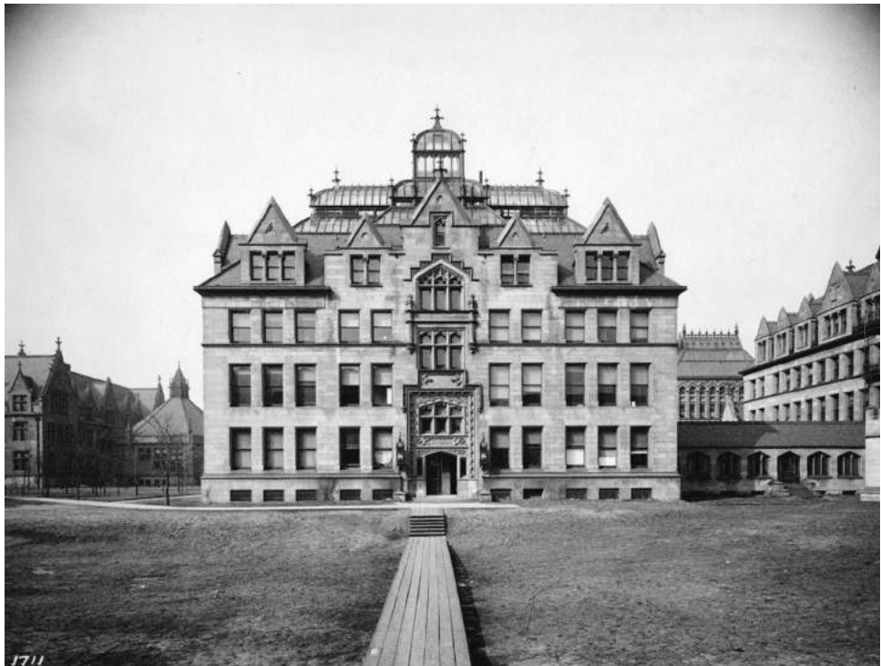
FIGURE 31. The east face of the Botany Building, Hull Biological Laboratories, University of Chicago, Chicago, Illinois. The greenhouse was ornamented with neo-Gothic forms in keeping with the rest of the campus architecture. American Environmental Photographs Collection, [APF2-01053], Special Collections Research Center, University of Chicago Library.
