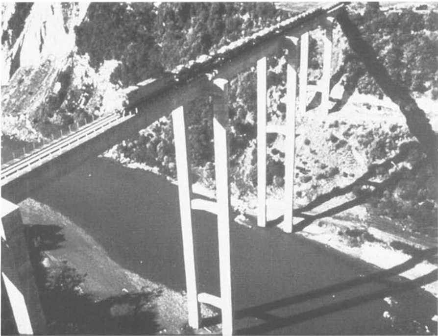
Fig. 3.11 South Rangitikei River Bridge.
