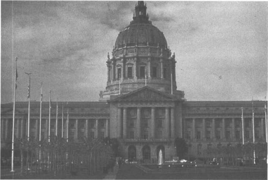
Fig. 1.10 San Francisco City Hall, San Francisco, California.
