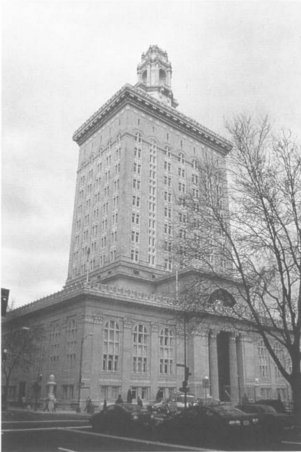
Fig. 1.9 Oakland City Hall, Oakland, California. (Photo courtesy of SIE, Inc.)
