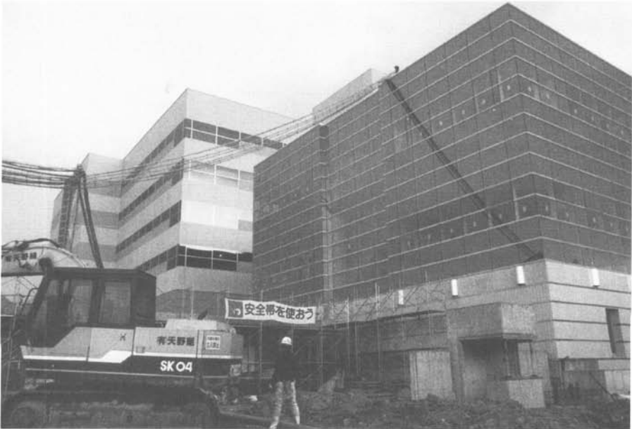
Fig. 1.17 Matsumura-Gumi Technical Research Institute.
