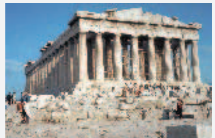
The Parthenon in Athens, Greece, was completed in 438 B.C. and is an example of early column and beam masonry construction.
