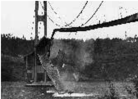
Figure 1.8 Failure of the Tacoma Narrows bridge in Tacoma, Washington, in 1940, due to severe vibrations produced by a 42 mph wind.
