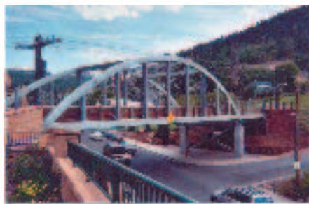
Figure 6.3 While most truss structures are composed entirely of straight members, this truss uses a curved upper chord.
