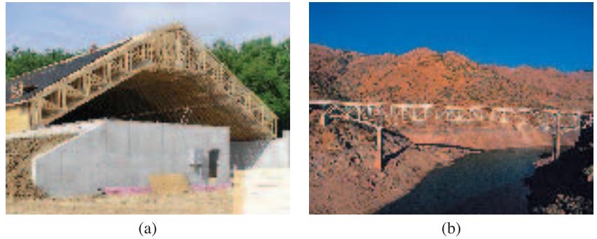
Figure 6.1. Examples of truss structures. (a) The roof of this highway maintenance building under construction uses 124 identical wooden roof trusses with 16 in. spacing. (b) Mores Creek bridge over Lucky Peak Reservoir near Boise, Idaho.
