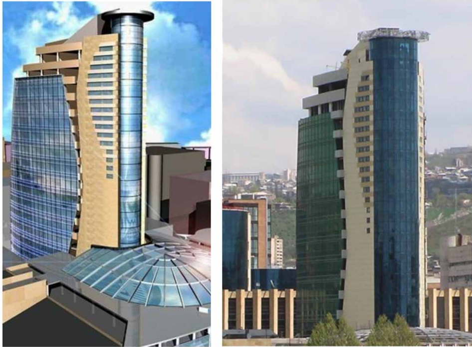
Figure 12. Architectural design view of the 20-story base isolated building of the “Elite Plaza” business center and its current view
