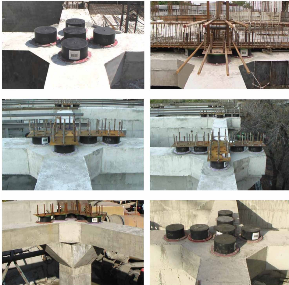
Figure 7. Examples on installation of clusters with different numbers of rubber bearings
