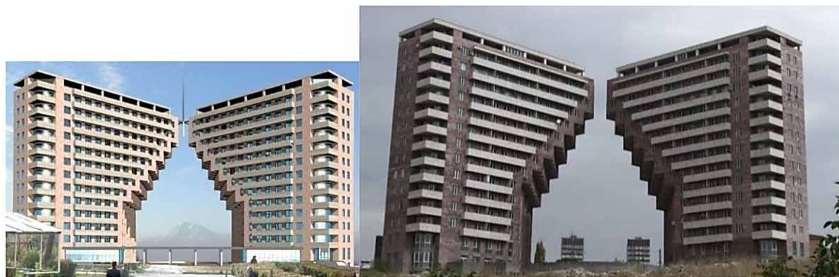
Figure 16. Architectural design view of the 18-story base isolated buildings/twins of the multifunctional residential complex “Northern Ray” from the Northern side (left) and the current view of the constructed base isolated buildings/twins from the Southern side (right)
