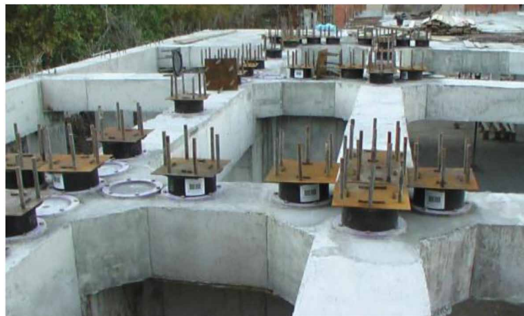
Figure 6. Construction process on installation of small size rubber bearings clusters
