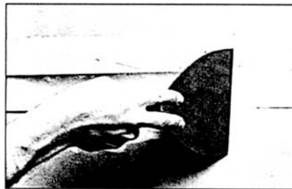
1. Fill Joint And Bed Tape Simultaneously
