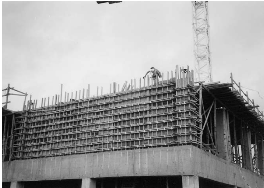
FIGURE 8.5 Plyform system for wall and column construction.
