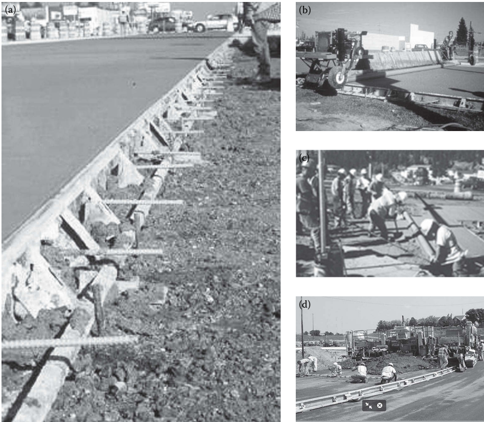
FIGURE 17.9 Typical fixed form construction operations. (ACPA)
