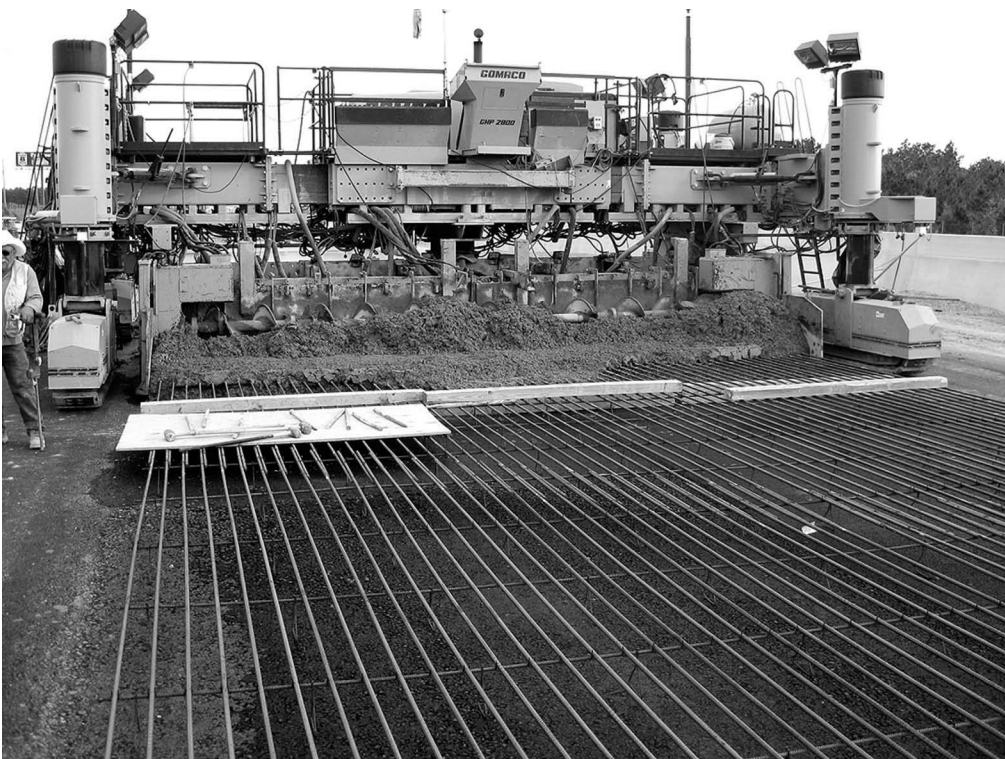
FIGURE 16.28 CRCP under construction.
