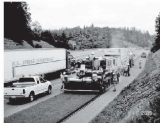
Recycling with traffic in adjacent lane
