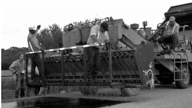
FIGURE 20.6 Chip seal. (Courtesy of Maureen Kestler, USDA Forest Services, Washington, DC.)
