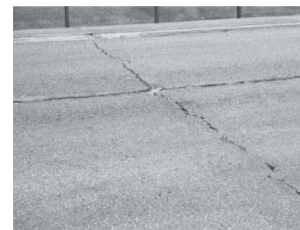
Reflective cracking
