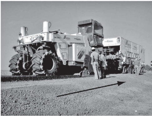
FDR using WR 2500S recycler and WM 100 cement slurry equipment
