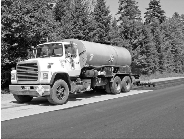
FIGURE 13.12 Application of tack coat. (Courtesy of Carolina Carbo, Road Recycling Council.)
