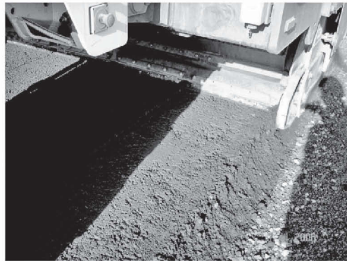
300 mm FDR with cement slurry with 5.8% cement
