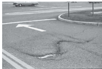
Slippage crack
