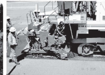
WR 4200 fitted with integral voguele AB500 tamping and vibrating paving screed
