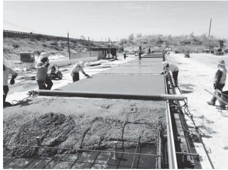
Pretensioning process
