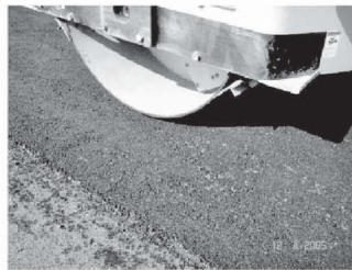
Compaction with steel drum roller
