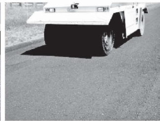
Finish rolling with rubber tired roller
