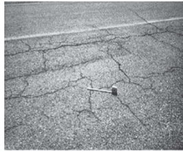
Block cracking
