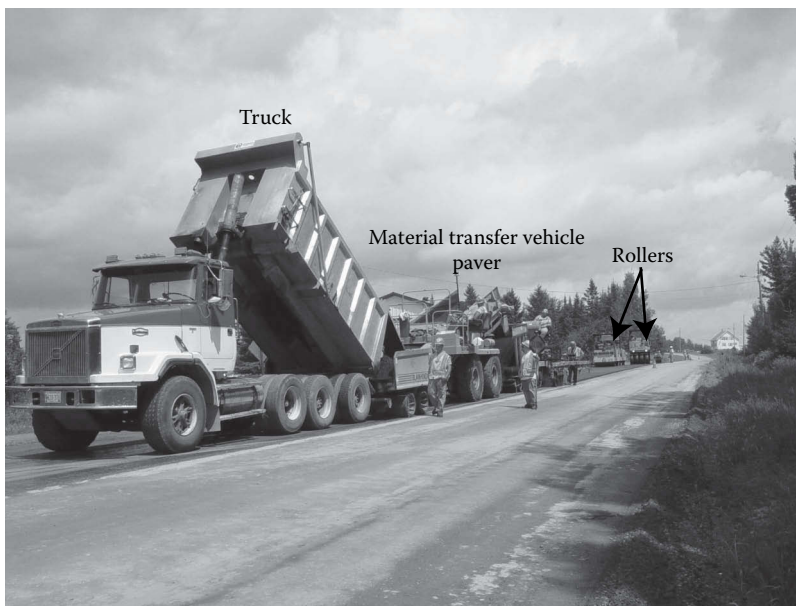
FIGURE 13.13 Different equipment used in hot mix asphalt paving. (Courtesy of Carolina Carbo, Road Recycling Council.)
