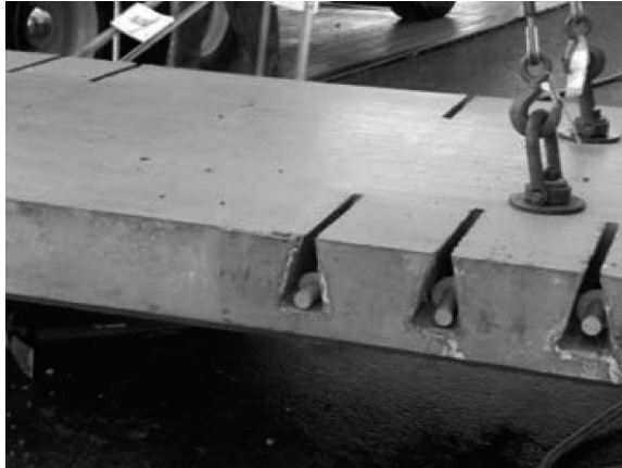
FIGURE 18.7 SHRP2-developed surface slot system, standard version. (Photo Courtesy of Shiraz Tayabji, Applied research associates, Inc.)
