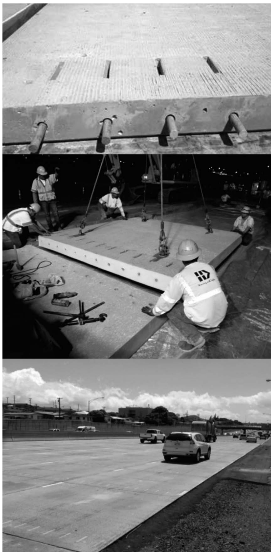
FIGURE 18.8 Rapid roadway system's Barra Glide load transfer feature showing the dowel inserted through partially open narrow slots at the surface of the precast panel and the finished gouted panels in service. (Courtesy of Shiraz Tayebji, Applied research associates Inc.)
