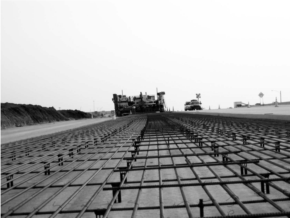
FIGURE 16.27 CRCP under construction.
