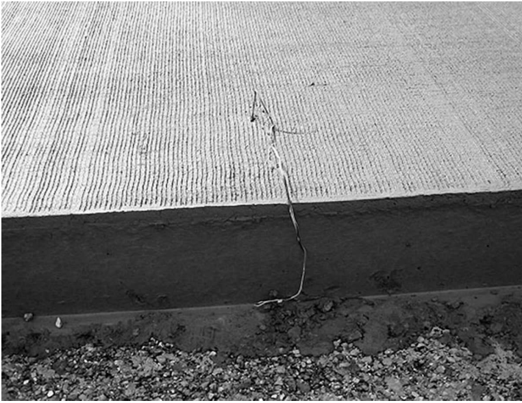
FIGURE 17.23 Field testing of concrete temperature for using the maturity test. (Courtesy of wouter gulden, aca-se chapter, duluth, ga.)
