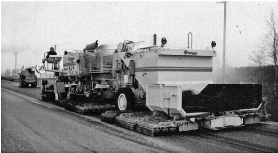
FIGURE 20.8 Hot in-place recycling.
