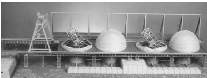
Fig. 11.5. Early VLT concept for open-air operation. Enclosures made of fabric were to protect each telescope during the day and be retracted at night. A windscreen made of tiltable louvers was to protect the telescopes from prevailing winds [5, 6, 7]. This approach was not implemented because telescope and mirror wind shake was determined to be excessive [8].
