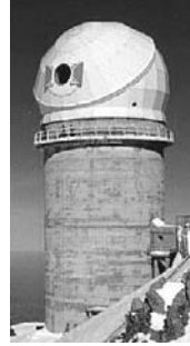
Fig. 11.9. Isolating the telescope from the inside of the enclosure and from the outside eliminates enclosure seeing in principle, but this requires a large glass plate to close off the top of the telescope tube. This solution was only partially implemented for the Pic-du-Midi 2-meter telescope shown on the right, as the glass plate was never installed. (Photo by Robert Futaully, courtesy of Observatoire Midi-Pyrénées.)
