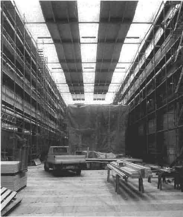
FIGURE 11.50 The laboratory hall with the glazed roof during retrofit work.
