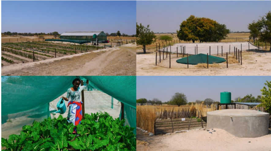
Fig. 3.3 CuveWaters rainwater harvesting pilot plants (from top left clockwise: communal approach with greenhouse and outside garden, communal approach ground catchment with underground tank, household approach ferrocement tank with garden, spinach inside household greenhouse) (Liehr et al. 2015)
