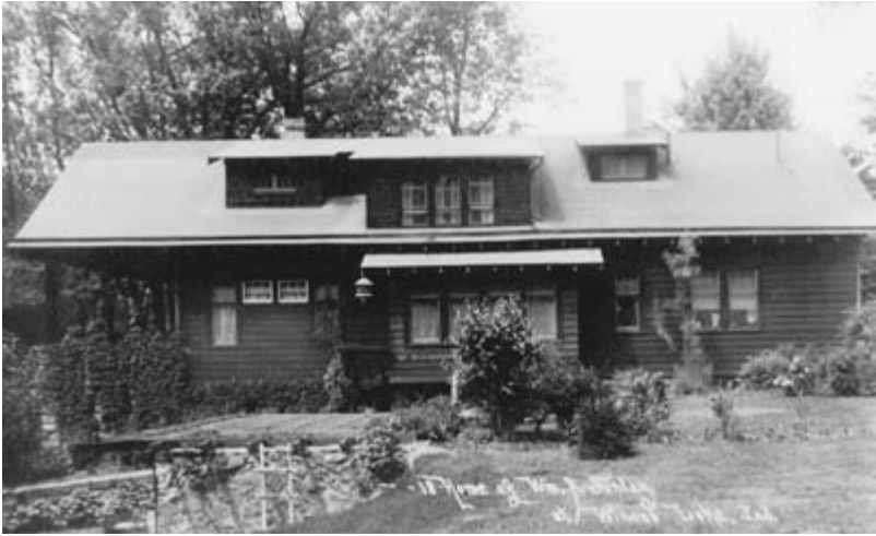
FIGURE 40. South facade of Mount Hood bungalow showing details of shed dormer construction, exposed rafter tails, banded window design, and landscape improvements circa 1925. Image courtesy of the Reneker Museum of Winona History, Grace College, Winona Lake, Indiana.
