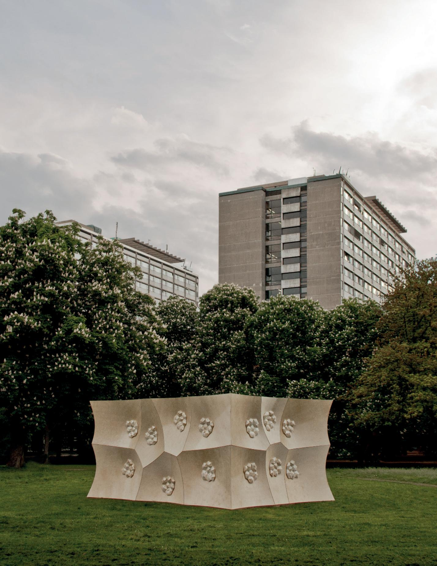
through a repetitive and parametrically adaptive production process. In this context the geometry of a standard conical surface was of particular interest. Developable surfaces like the cone offer the opportunity to construct a geometrically stiff module from initially flat and elastic sheets.
