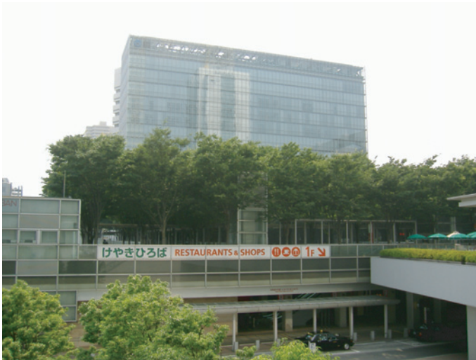
Fig. 15.6. External view of Keyaki Hiroba (Zelkova Tree Plaza) with rooftop vegetation, built in 2001 in Saitama City, Saitama Prefecture, Japan.
