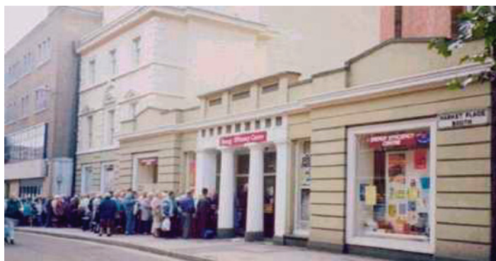
Fig. 21.1. Leicester Energy Efficiency Centre.
