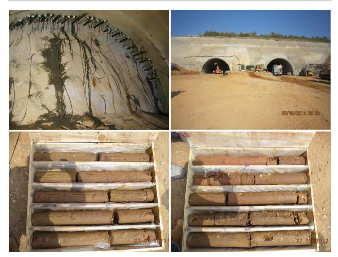
Fig. 55.1 View on borehole core samples, tunnel tubes and forepoles as a face protection
