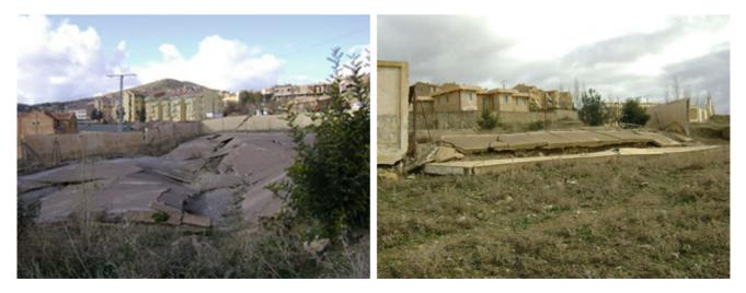
Fig. 191.2 Landslide causing disorders to the stadium and surrounding wall
