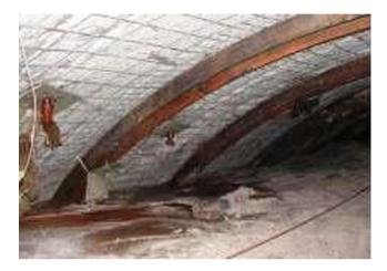
Fig. 172.3 Heavy discharge with slush in Parbati HRT
