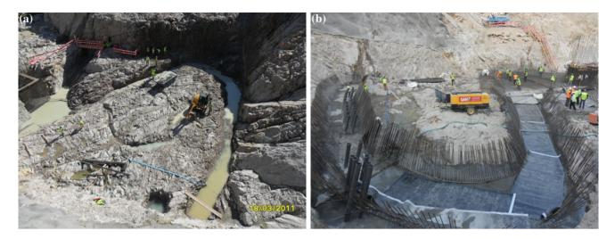
Fig. 10.6 a River bed faults excavations (*facing downstream*). b Placed reinforced concrete and PVC molds for posterior cement grout injection (*facing upstream*)
