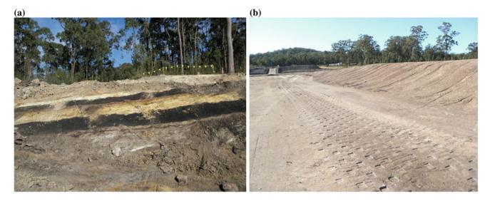
Fig. 45.2 Tuffs encountered while constructing the Hunter expressway. a Several tuff bands in a cutting. b Reworked material in compacted fill
