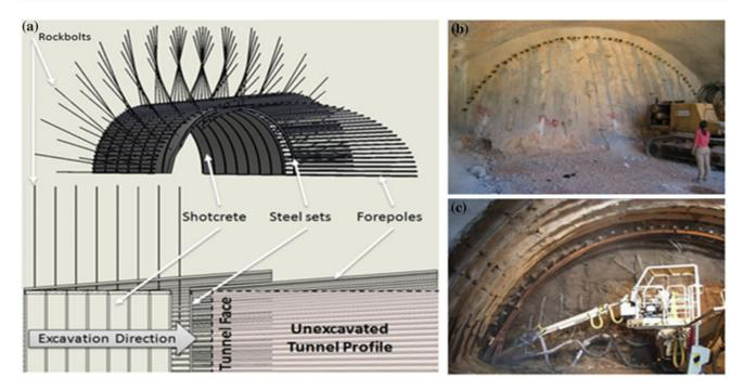
Fig. 157.1 a Nominal temporary structural support system used as part of the observational method of support. Elements shown are: forepoles without niches; steel sets (i.e. H-piles); *shotcrete*; and
