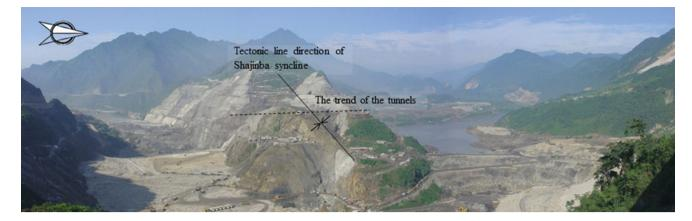
Fig. 83.2 The direction of the tunnels is intersected with the tectonic line of Shajinba syncline
