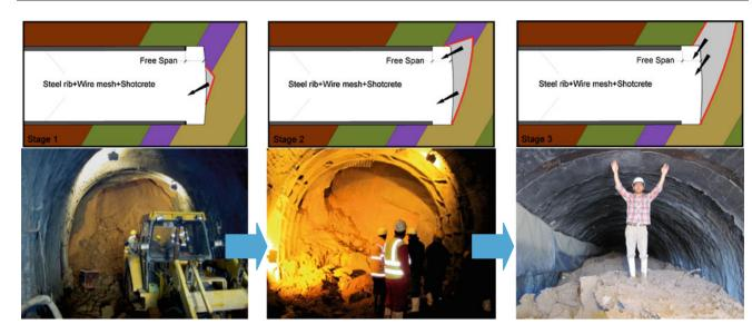
Fig. 107.5 Collapse in initial part of Sabzkuh tunnel (T1) (Eftekhari et al. 2013b)
