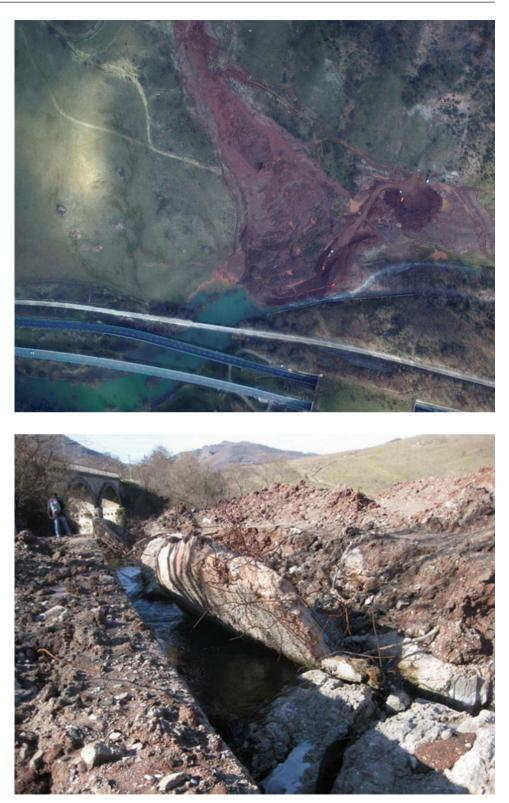
**Fig. 135.2** Basento River occluded by landslide debris and parts of existing retaining wall
