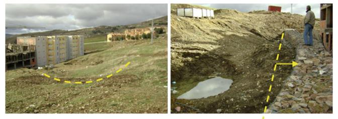
Fig. 191.3 Titling and moving retaining wall
