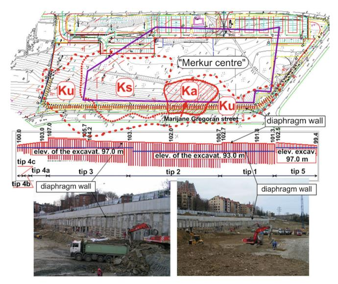
Fig. 47.4 Protection of foundation excavation
