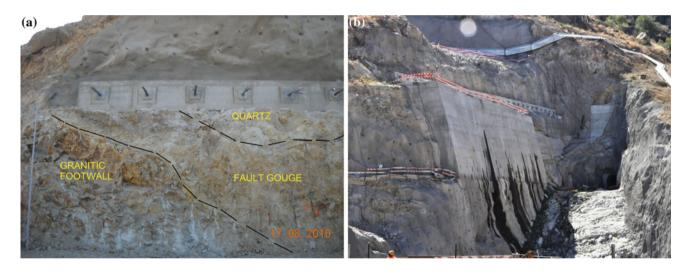
Fig. 10.5 a Fault nº 24. b Support wall and pre-stressed anchor beam
