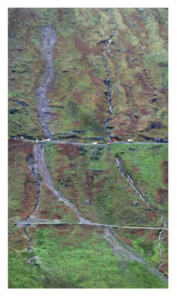
**Fig. 113.1** Debris flow of 03:00 h on Sunday 28 October 2007 at the A83 rest and be thankful. The head scar is at 370 m, A83 at 240 m and the old road at 180 m. Both recent (*lighter area*) and older (*darker*) erosion is visible below the main road and to the left of the recent scar
