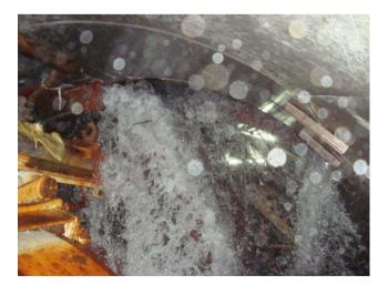
Fig. 171.3 Water ingress from segment No. 1905
