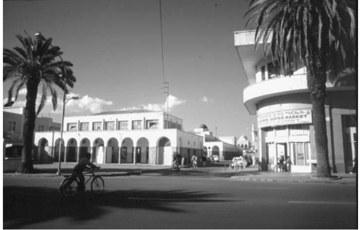
Figure 9.6 View (left and center) of fish, meat, and vegetable markets, and the Great Mosque adjoining the Viale Mussolini (now Harnet Avenue) in Asmara (1938, Architect Guido Ferrazza). On the right, Palazzo Mutton (the Mutton Building), resembling the well-known Novocomum by Giuseppe Terragni (Architect Antonio Vitaliti).
