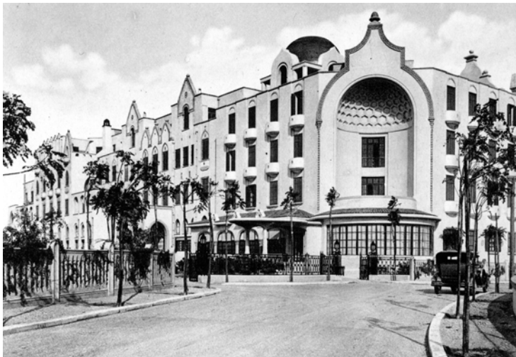
Intro.2 Rhodes: the Hotel of the Roses (Grande Albergo delle rose), with its original ornamentation (1927, Architects Michele Platania and Florestano di Fausto).
