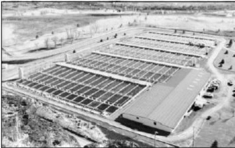
Fig. 15.12. Raceways used for trout production. Source: DEQ [5].
