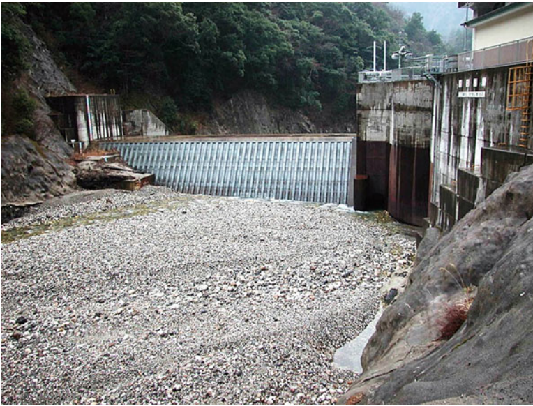
Fig. 5.16. Upstream area of Asahi reservoir, Japan, showing entrance to gravel bypass tunnel on the right and cofferdam which directs flood flows into the tunnel (photo G. Morris).
