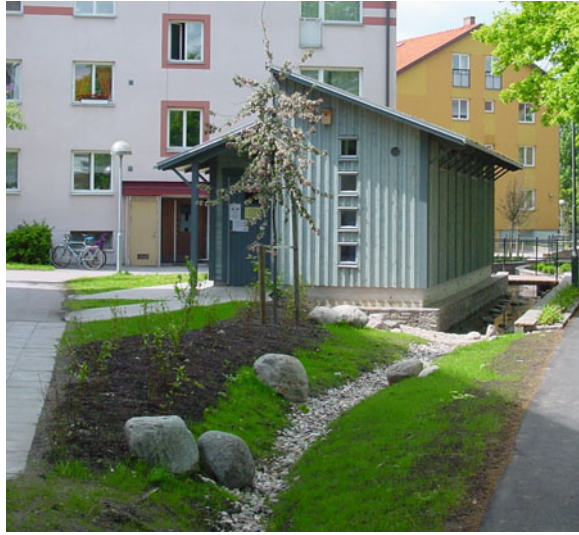
Fig. 4.8 One of 13 recycling buildings in the Augustenborg area
