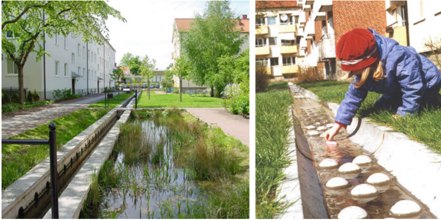
Fig. 4.7 Open storm water management system in the Augustenborg residential area. Photo Malmö City Urban Planning Office
