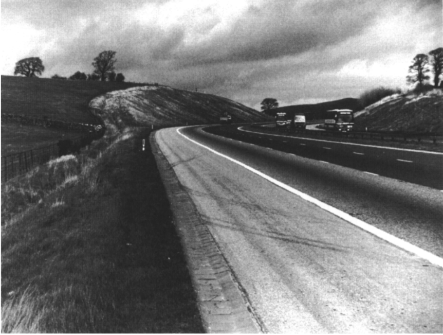
Figure 3.5 Should this road embankment have been contoured and managed to resemble the adjoining fields?
