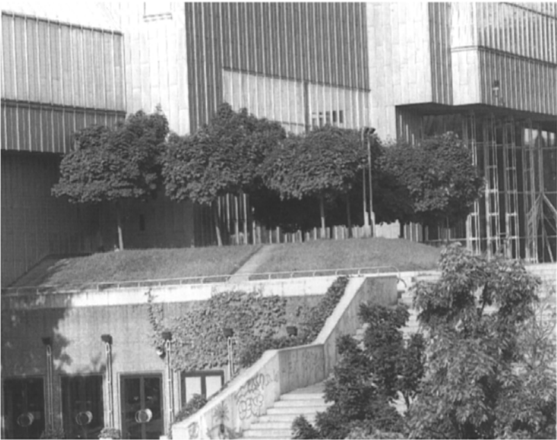
Figure 9.15 Vegetated roofs are interesting, beautiful, good for thermal insulation and of value as wildlife habitats. Above, London. Below, Cologne.
