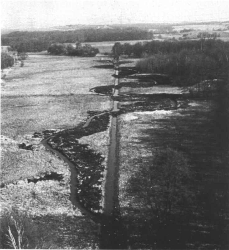
Figure 9.6 The River Wandse, in Germany, previously straightened by river engineers, was restored to its old meandering course in the 1980s. (Photo courtesy of Freie und Hansestadt Hamburg.)
