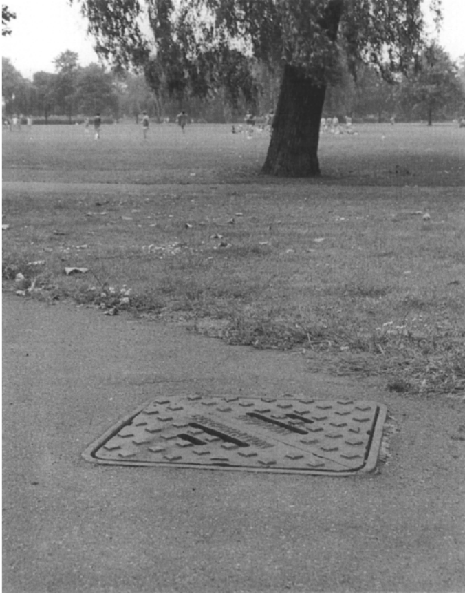
Figure 9.9 A manhole marking the route of the River Wandle, beloved by John Ruskin, as it passes through Wandle Park. Some day, it will be reclaimed.
