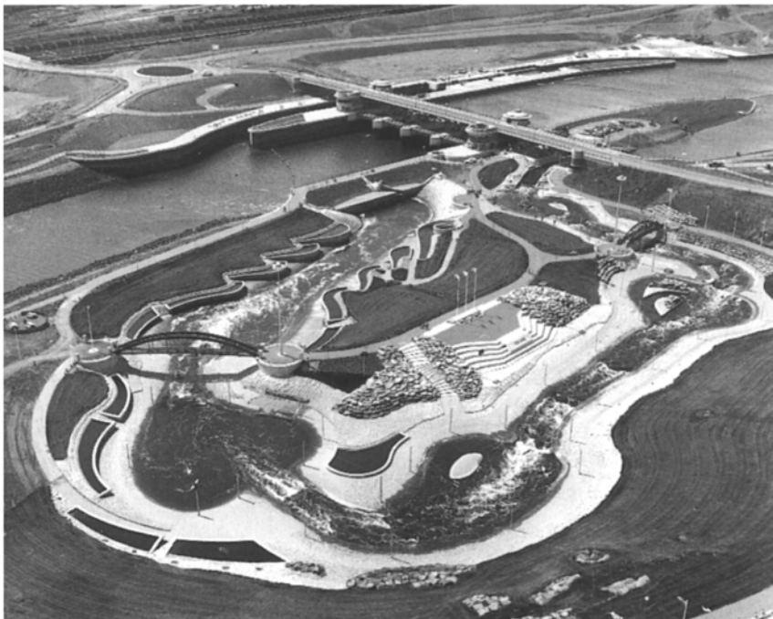
Figure 9.22 The Tees Barrage and Teesside Whitewater Course Flagship Schemes of Teesside Development Corporation is an excellent modern example of a multipurpose river control structure. (Courtesy of SGS Environmental and Teesside Development Corporation.)
