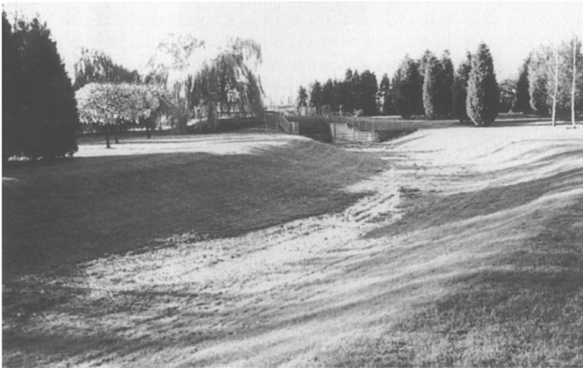
Figure 9.14 Storm detention basins on the River Cray in south-east London. The wet basin (above) is beautiful in time of flood, reminding one of the swamps that used to characterize the winter landscape of northern Europe. The dry basin (below) is a soggy area in an otherwise dull expanse of public park: it should be re-designed as a wetland habitat.
