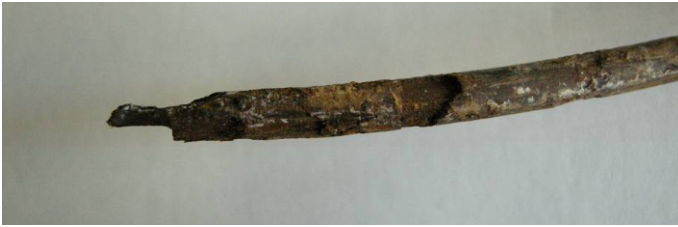
Figure 1. Example of penetrating corrosion attacks observed on a wire of the failed cable
