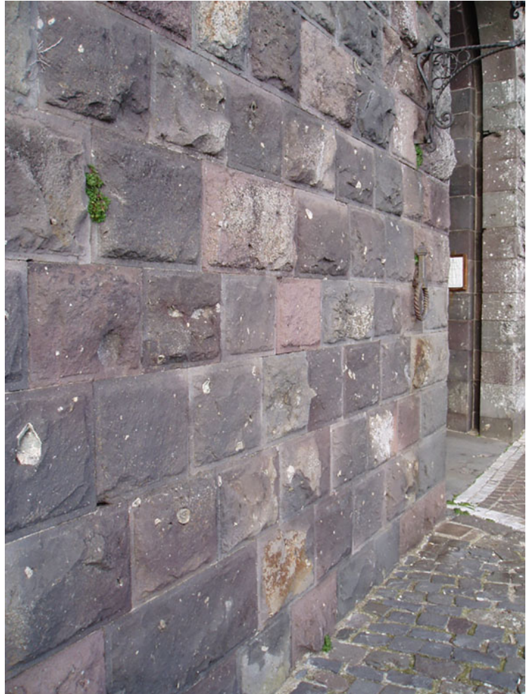
Fig. 2.10 Front wall of the Torre Alfina castle showing large amounts of a wide variety of crustal and mantle xenoliths in the lamproite lavas
