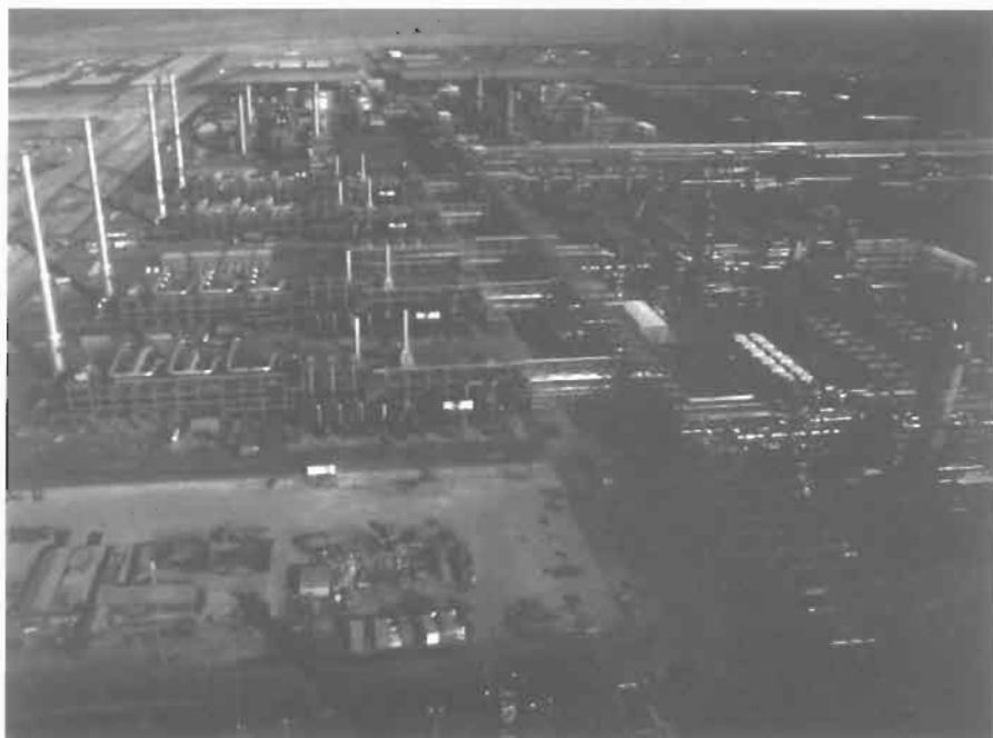
Figure 2-2a. Shedgum, Saudi Arabia, gas treating complex. 4 \times 540 MMscfd Improved Econamine trains using DGA on right, four Claus plants with incinerator stacks on left. For each Improved Econamine train, contactor is on right, regenerator on left. From left, air cooler sequence is regenerator condenser, lean DGA cooler No. 1, lean DGA cooler No. 2, and contactor side cooler. Courtesy Fluor Daniel
