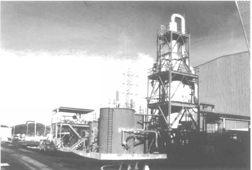
Figure 9-24. Stretford plant on geothermal, noncondensable gas. Courtesy of ABB Environmental Systems
