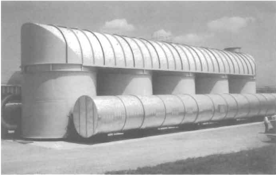
Figure 13-4. A 145,000-scfm five-bed regenerative oxidizer with 86% heat recovery at a paper and film coating facility. Courtesy of Smith Environmental Corporation
