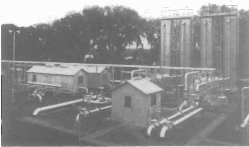
Figure 12-2. A typical natural gas dehydration plant employing dry desiccant in vertical vessels. Courtesy of United Gas Pipe Line Company
