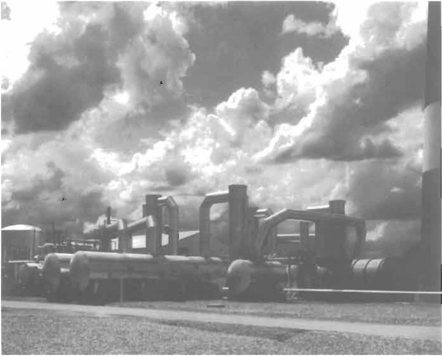
Figure 8-4. Claus-type sulfur plant producing 875 long tons of sulfur per day. Courtesy The Parsons Corp.
