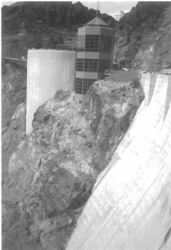
Figure 17.1 Hoover Dam on the Arizona–Nevada border, USA, (top) and the abutment rock (lower).
