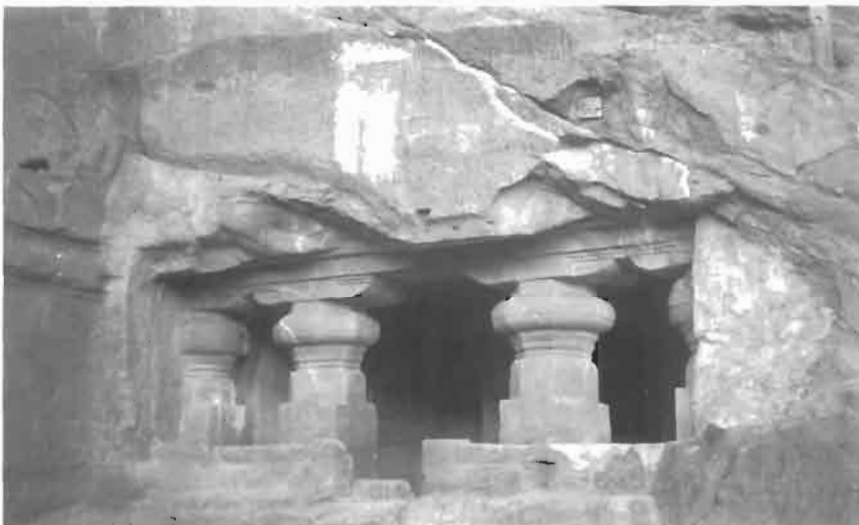
Figure 2.1 9th century monolithic Buddhist temples excavated in the Deccan basalts in India.
