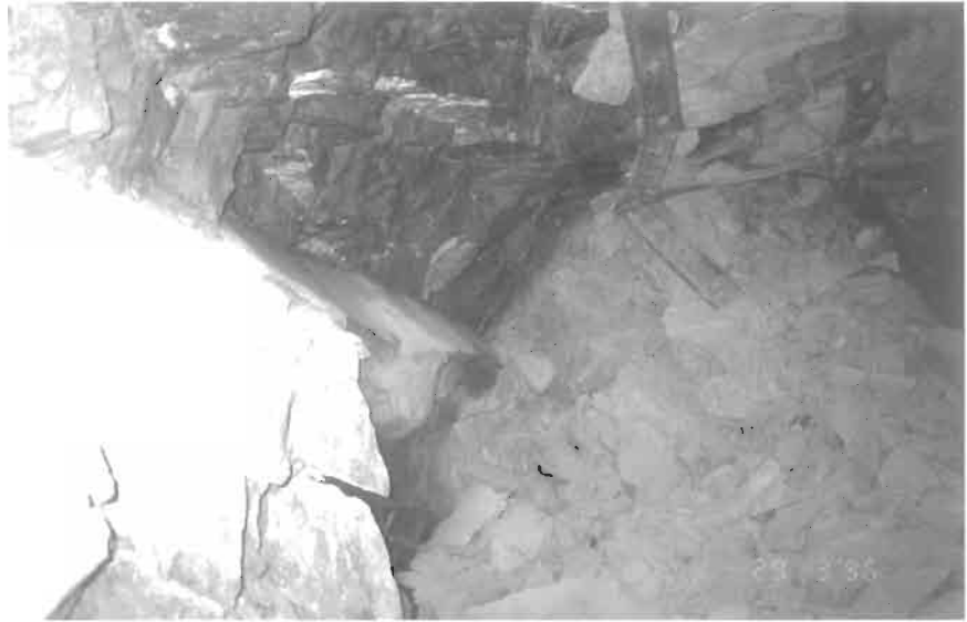
Figure 20.2 Interaction of high stresses and rock mass fractures has combined to cause failure of the rock mass and the installed support in an underground gold mine.
