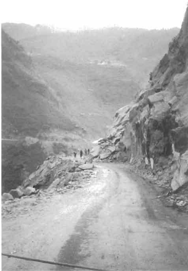
Figure 18.3 Unstable rock masses along Highway 22 from India to Tibet.
