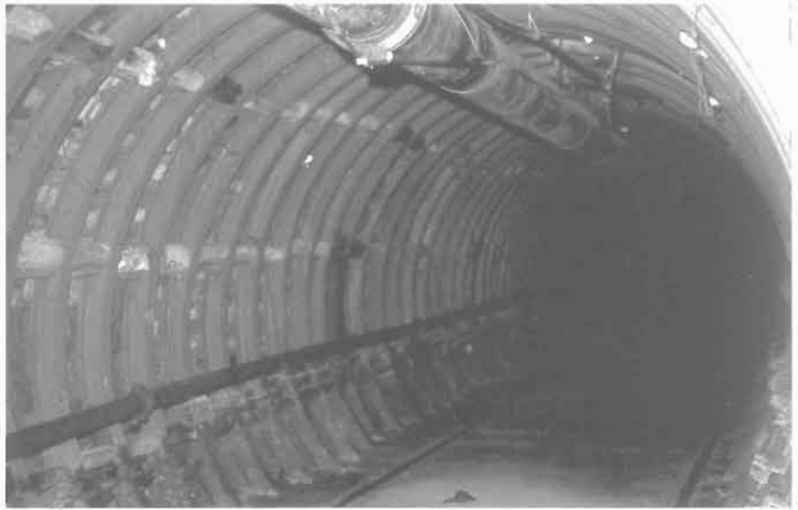
Figure 19.4 Pilot tunnel with steel arch support.
