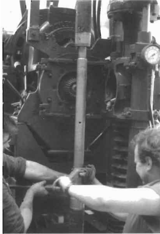
Figure 4.6 Hydraulic fracturing straddle packer system being lowered into a borehole during stress measurement tests in Cornwall, UK.
