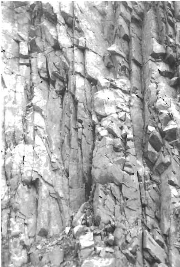
Figure 2.3 Zone of highly fractured rock.
