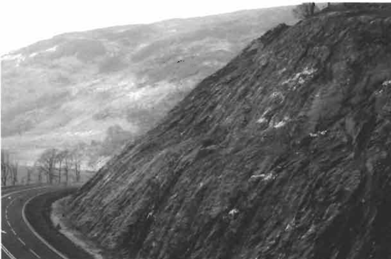
Figure 1.4 Example of a rock face made by pre-split blasting to give a stable, relatively smooth finish.
