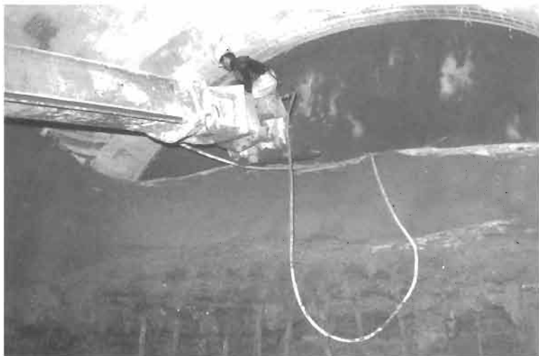
Figure 16.9 Construction of the Bochum metro in Germany.
