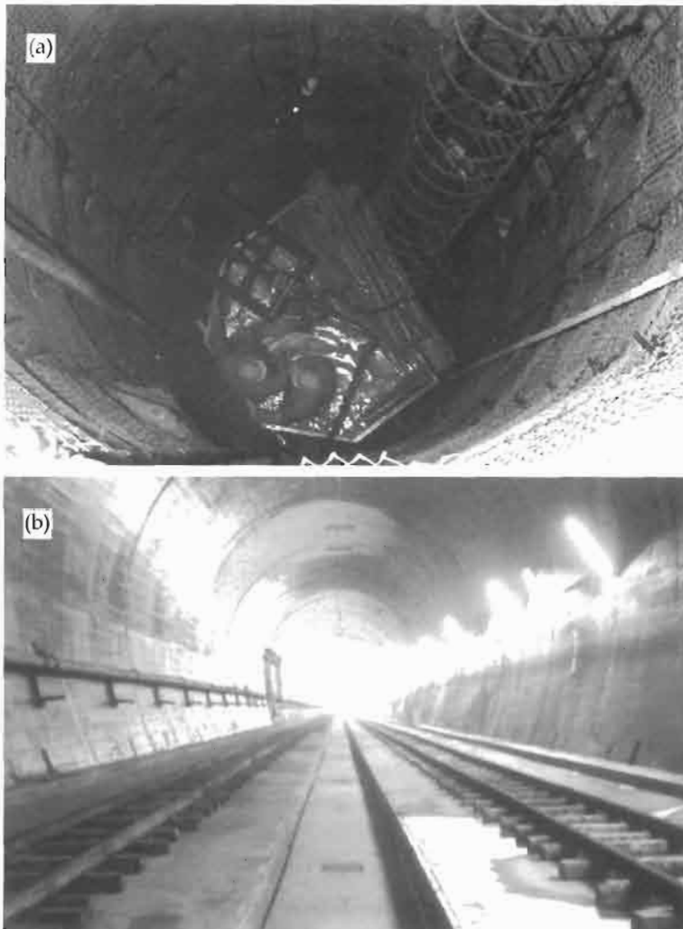
Figure 16.3 Illustrations of (a) rock reinforcement and (b) rock support.
