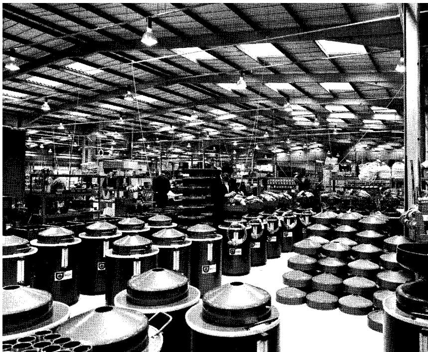
Figure 3.7.2 Factory lighting of correct illuminance, free from shadow and glare, making use of high pressure discharge lamps. (Courtesy Thorn Lighting Ltd)
