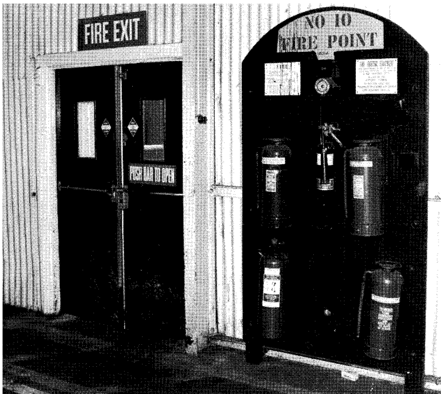
Figure 4.2.5 Clear unobstructed fire point (Courtesy Reed Medway Sacks Ltd)
