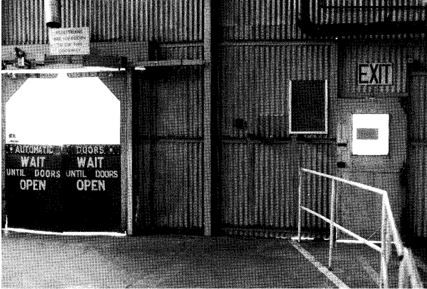
Figure 4.3.17 Separation of truck and pedestrian gangways
