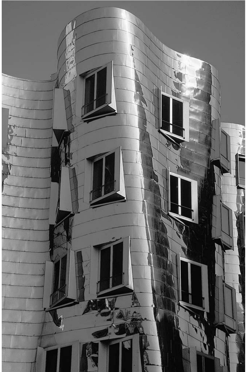
▲ 4.45 Der Neue Zollhof. Detail of stainless steel cladding with mirror finish on middle building. Photo: Author.
