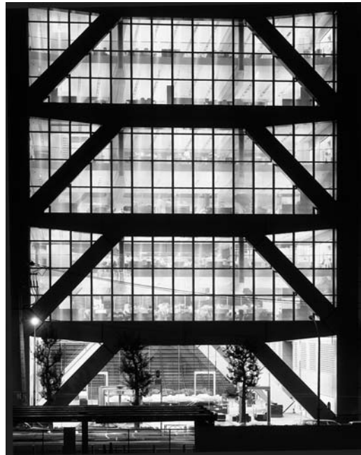
▲ 4.24 Century Tower, Tokyo, Japan. Detail of two-storey high structural frames. Norman Foster, 1987–91. Photo: Martin Charles.
