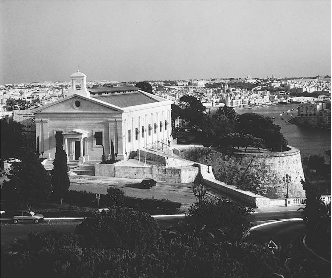
▲ 6.10 Malta Stock Exchange, Valletta, Malta. View of British Garrison Chapel and Valletta fortifications with Grand Harbour beyond. Architecture Project, 1994–2001. Photo: David Pisani.
