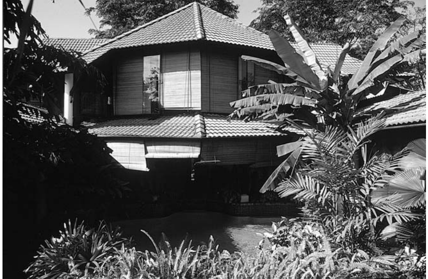
► 1.8 Precima House, Kuala Lumpur, Malaysia. Jimmy Lim, 1987–9. Lim's suburban house designs are strongly influenced by regional archetypes and techniques of climate control. Photo: Author.
