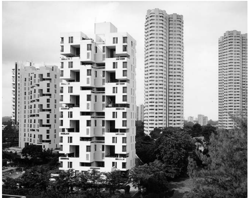
► 1.16 Ardmore Condominium, Singapore. Moshe Safdi, 1984. Pioneering high-rise design features two-storey sky-courts, one of earliest of its type. Photo: Cymie Payne.
