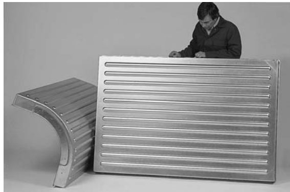
► 4.16 Sainsbury Centre For Visual Arts. Two of original aluminium cladding panels. Photo: Richard Davies.
