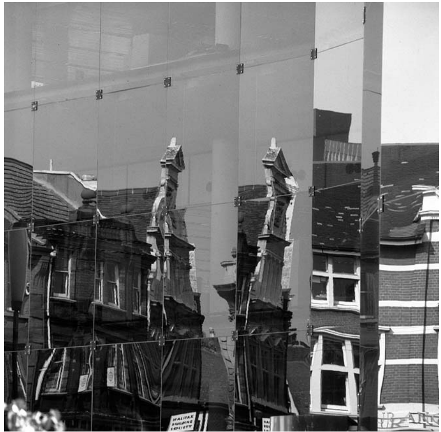
▲ 4.17 Willis Faber & Dumas Headquarters, Ipswich, UK. Detail of glass wall. Norman Foster, 1971–5. Photo: John Donat.
