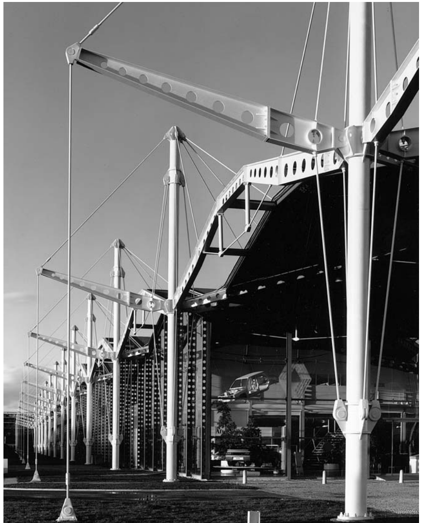
▲ 4.19 Renault Distribution Centre, Swindon, UK. Norman Foster, 1980–2. Photo: Dennis Gilbert.
