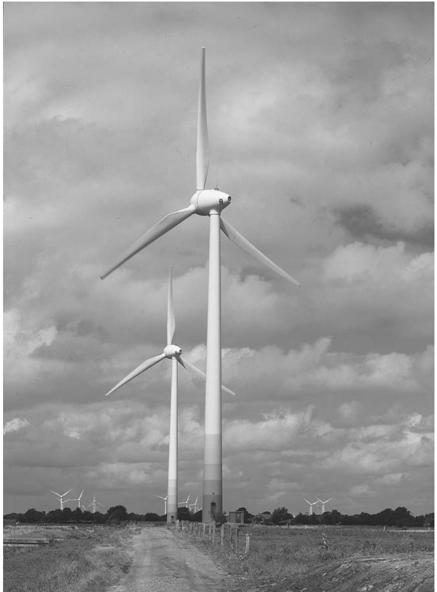
▲ 4.57 Enercon E66 Wind Turbines, Holtriem wind farm, Germany. Norman Foster, 1993. Photo: Nigel Young/Foster and Partners.
