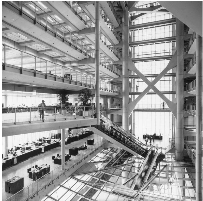
▲ 4.22 Hong Kong Bank. Interior of atrium with suspended glazed structure over entranceway. Photo: Ian Lambot.
