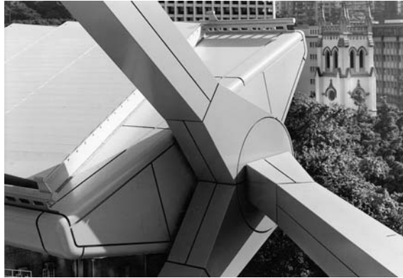
► 3.19 Hongkong and Shanghai Bank. Computer-controlled sunscoop deflects sunlight into atrium via mirrored ceiling. Photo: Richard Bryant.
