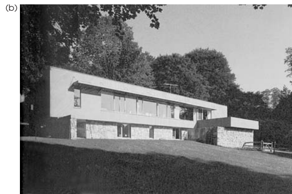
► 5.7 Cantilever House, New Canaan, by Marcel Breuer, 1947. Original design (a), and after final structural changes and extensions (b). Source: D. Masello, 1993.
