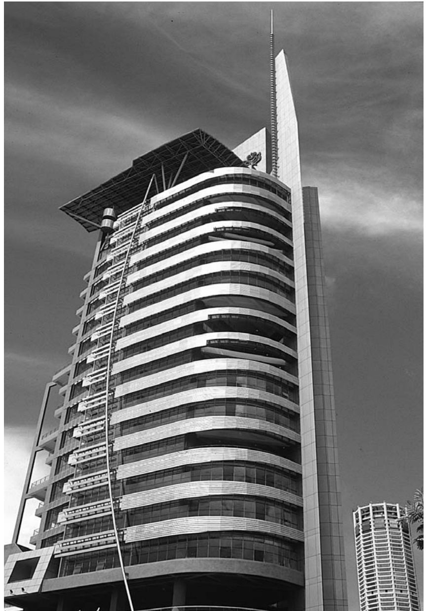
▲ 3.22 UMNO Party Headquarters, Penang, Malaysia. Hamzah and Yeang, 1995–8. Streamline form and external fins help control flow of air around and through tower, assisting cooling and ventilation. Photo: Author.
