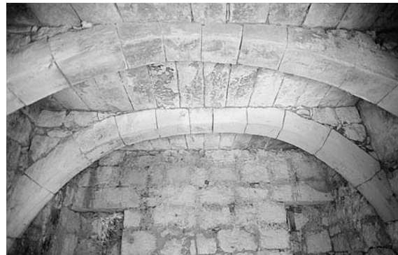
► 6.18 Vernacular stone house, Malta. Interior, showing vaulted roof construction. Photo: Author.
