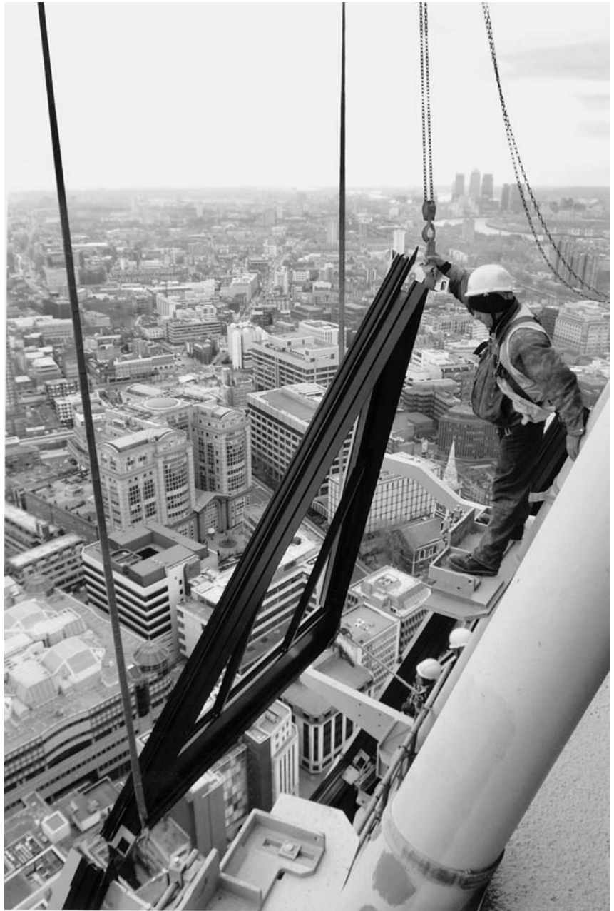
▲ A11.7 Swiss Re, London, England. Glazed cladding unit being hoisted into place. Norman Foster, 1997–2004. Photo: Norman Childs.
