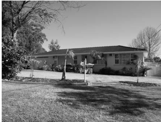
► 5.4 Typical suburban house, Sydney. Photo: Author.
