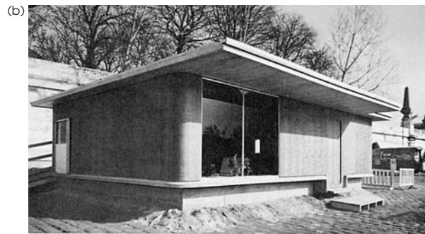
► 3.11 Metal House, 1955, plan (a), on site 1960 (b) by Jean Prouvé. Source: J. Prouvé, 1965.
