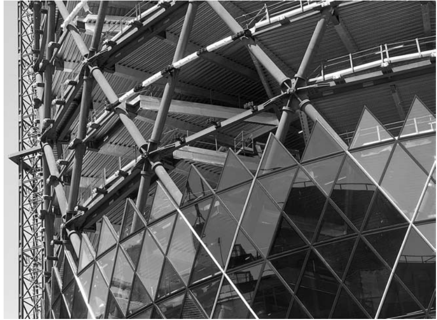
▲ 4.69 Swiss Re Headquarters. Detail of steel structure and cladding. Photo: Nigel Young/Foster and Partners.
