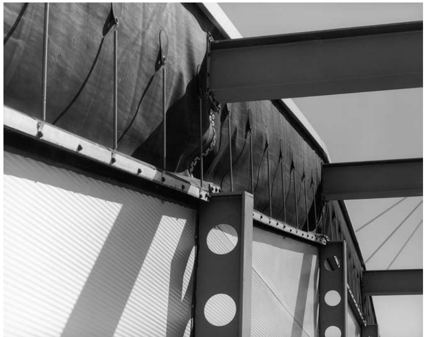
▲ 4.20 Renault Distribution Centre. Detail of flexible eaves showing spring fixings. Photo: Dennis Gilbert.
