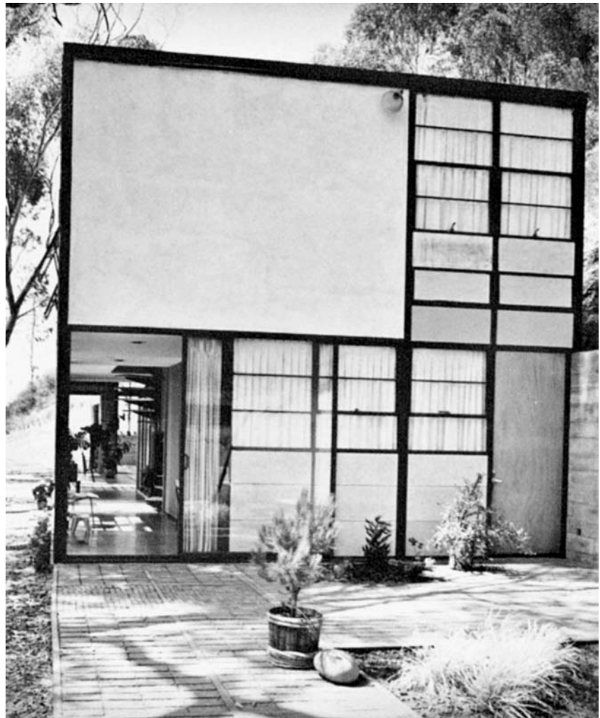
► 3.7 Eames House and Studio, Santa Monica, California, USA. Charles and Ray Eames, 1949. Made entirely from stock factory components, the neo-Japanese aesthetic helped soften house's prefabricated origins. Source: Museum of Modern Art, 1973.
