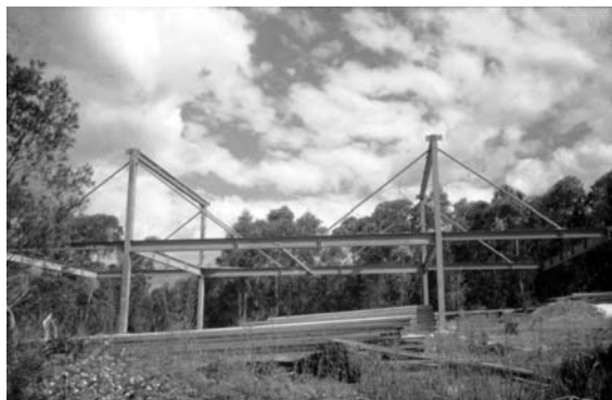
► 5.6 Steel-framed structure of Rose House. Photo: Marcell Seidler.
