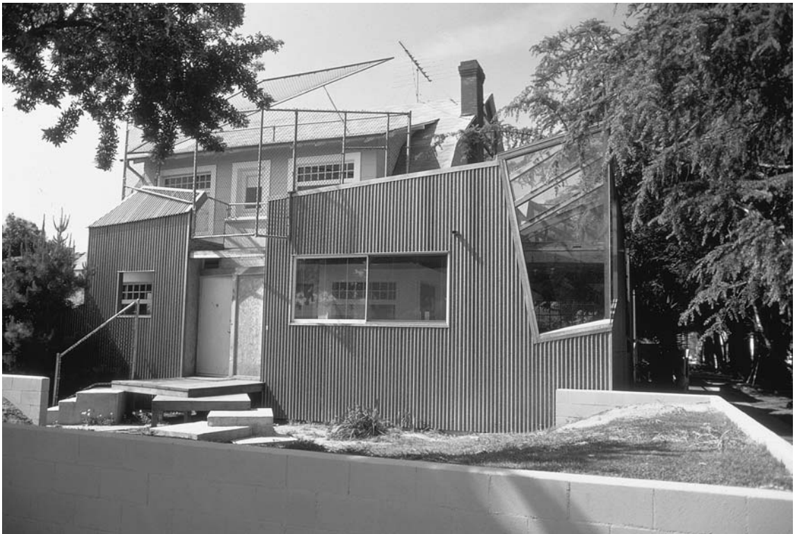
▲ 4.6 Architect's own house, Santa Monica, California, USA. Frank Gehry, 1978. Photo: Tim Street-Porter/Esto.
