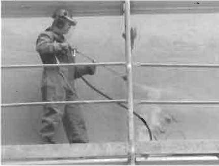
(c) Floor decontamination (Hammelmann GmbH, Oelde).
