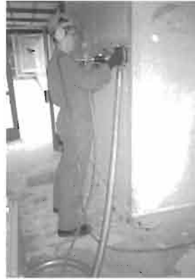
(b) Removal of PCB-contaminated plaster (DSW GmbH, Duisburg).
