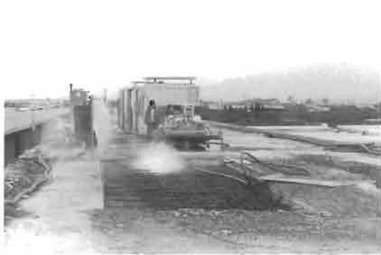
(e) Hydrodemolition (Aquajet AB, Holysbrunn).
