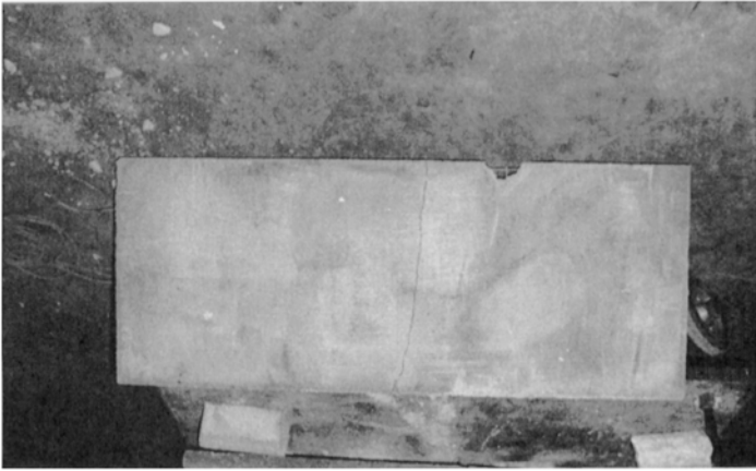
FIG. 10.26. Cracking pattern of cellular concrete panels.
