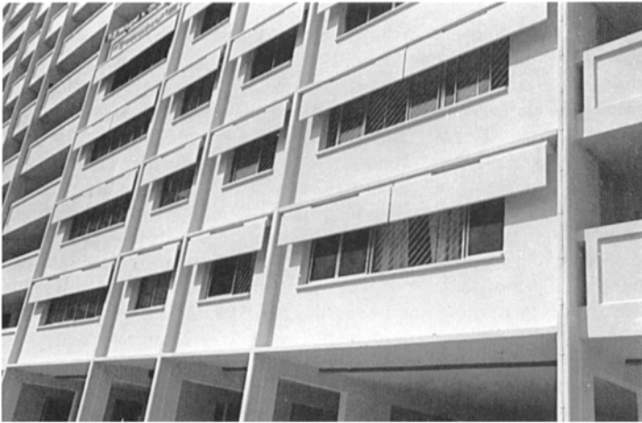
FIG. 10.14. A view of the building after installation of the sunscreen.
