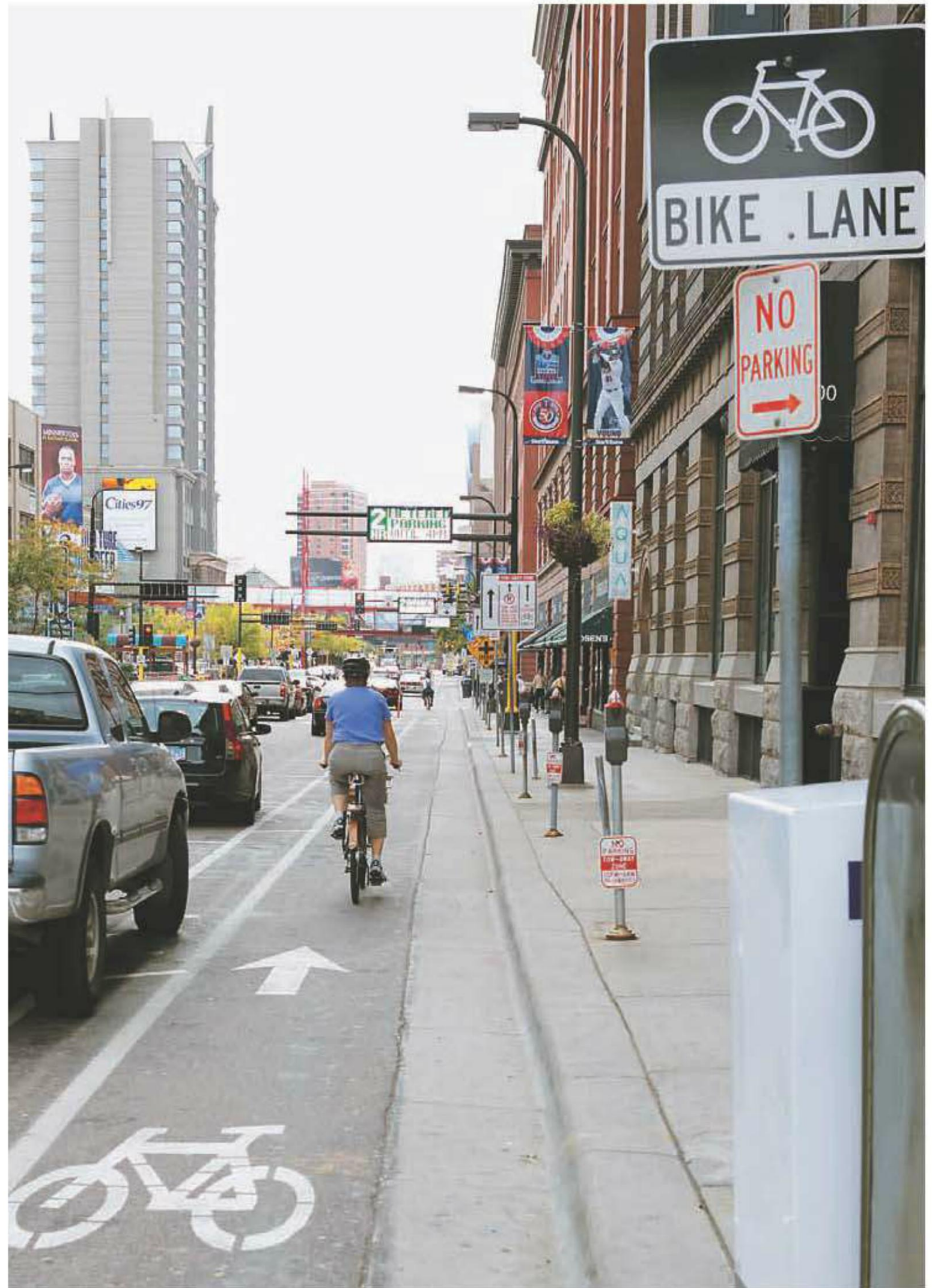
Bike lanes are configured in many ways. This bike lane in Minneapolis puts the riders between the curb and parked cars.
