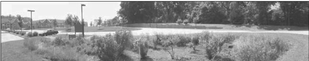
This traffic island has a “bioinfiltration” system to capture water. Photo courtesy Villanova Urban Stormwater Partnership.
