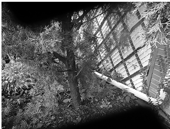
FIGURE 8.33 Planted area (filter strip) at a roof downspout of the author's residence.
