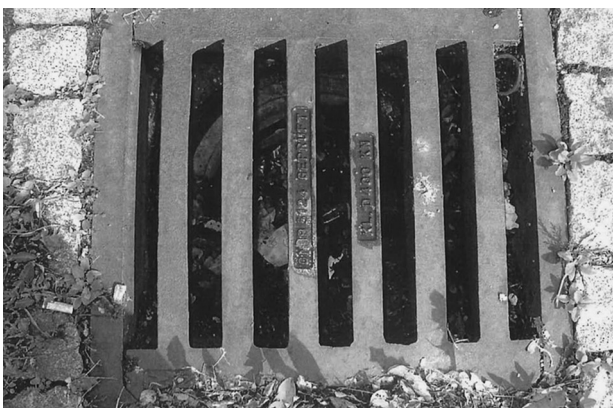
FIGURE 4.5 An inlet at a parking lot median, in a roadside service center in Austria.
