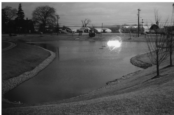
FIGURE 9.22 A rock-lined pond (designed by the author).
