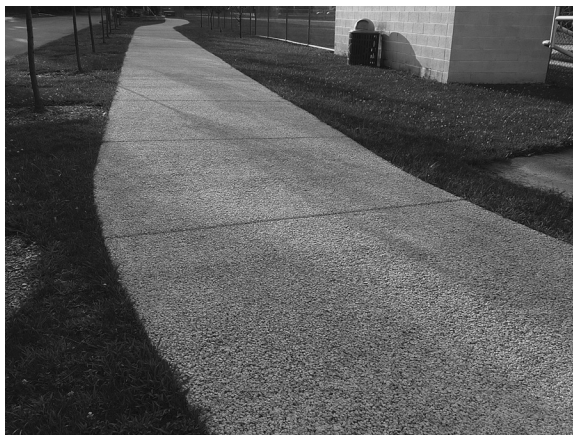
FIGURE 8.10 A pervious concrete sidewalk in Hogan Park, New Jersey.
