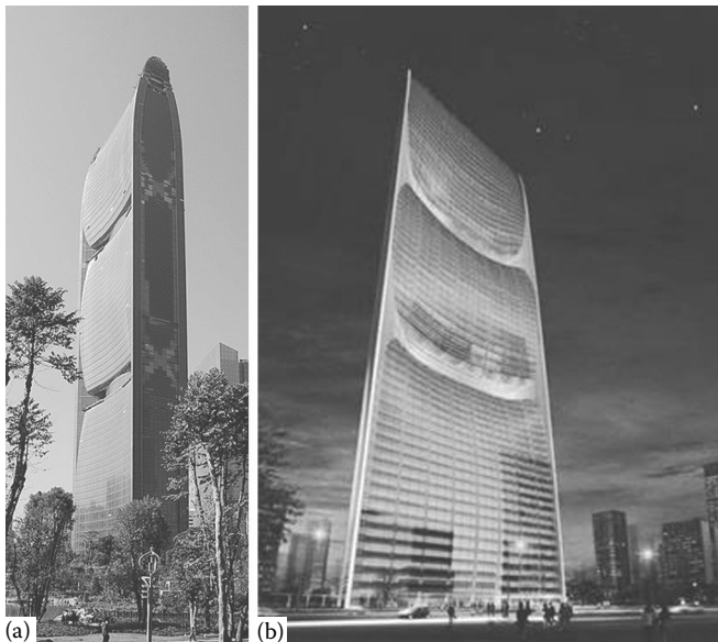
FIGURE 8.2 Images of Pearl River Tower. (a) Side view and (b) front view.
