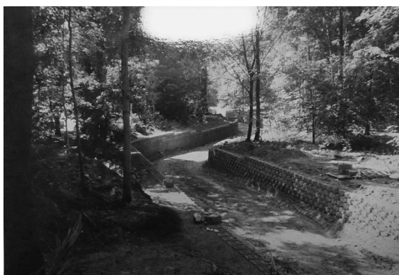
FIGURE 4.51 Keystone walls under construction in 1990. (Photo by the author.)
