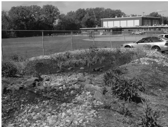
FIGURE 10.8 Rain garden adjacent to high school property to filter pollutants. (Photo by the author, 2014.)
