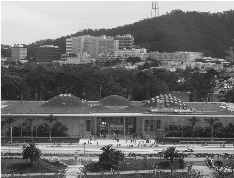
FIGURE 8.24 Undulating green roof of California Academy of Sciences in San Francisco. (Photo by the author, 2010.)
