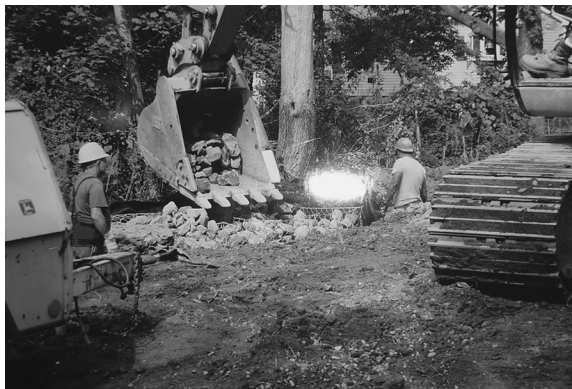
FIGURE 4.47 Gabion wall being installed. (Photo by the author.)
