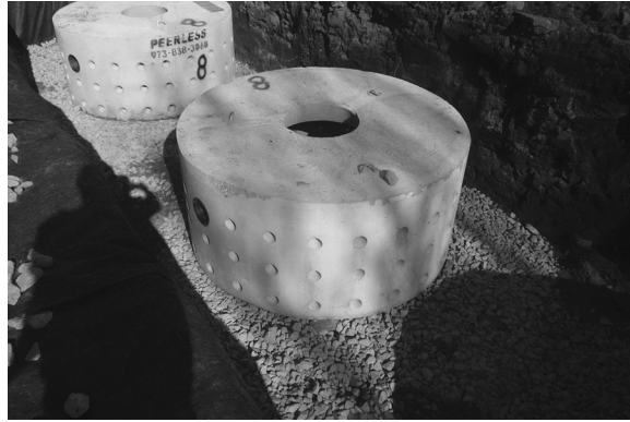
FIGURE 9.24 Seepage pits being installed in stone trench. (Photo by the author.)
