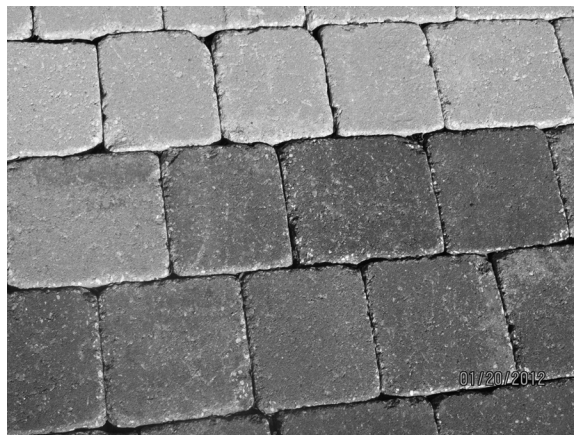
FIGURE 8.16 Unsanded paver walk at Lincoln Mall in South Beach, Florida. (Photo by the author, 2012.)
