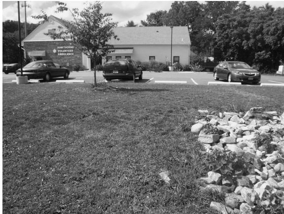
FIGURE 8.39 Rain basin retains runoff from roof and driveway of a North Jersey municipal fire station. The rocks at right protect the basin from erosion at the roof drain. (Photo by the author.)
