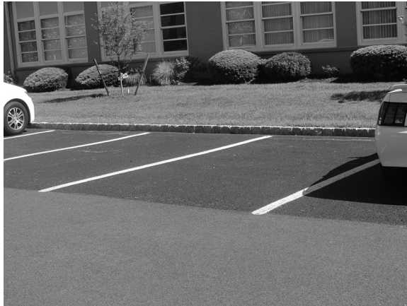
FIGURE 8.7 Porous asphalt at parking stalls, Municipal Building, Clark, New Jersey.
