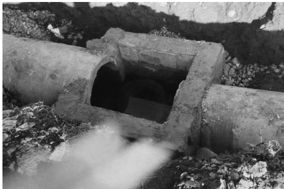
FIGURE 9.16 Pipe connection to an inlet using mortar. (Photo by the author.)
