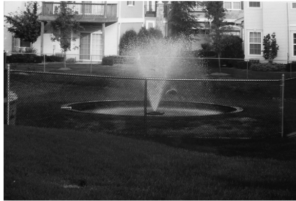
FIGURE 7.1 Grass-lined detention basin with center fountain. (Photo by the author.)
