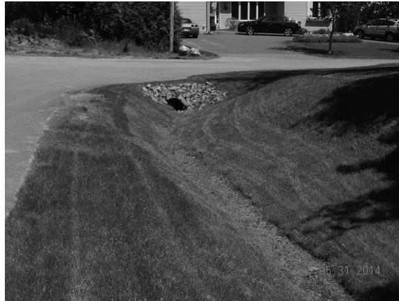
FIGURE 4.45 Grass-lined swale with gravel bed in Saint-Sauveur, Canada. (Photo by the author, 2014.)
