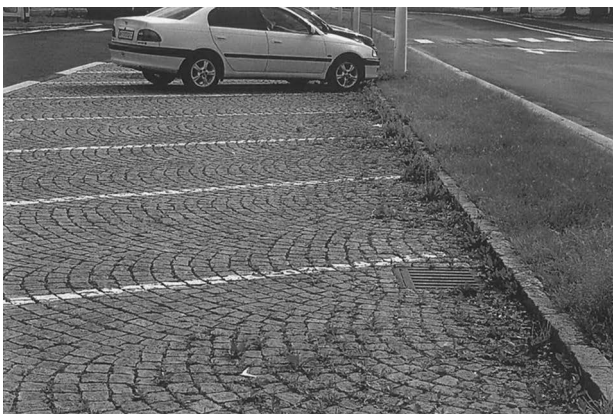
FIGURE 4.4 An inlet along a curb in Budapest, Hungary.
