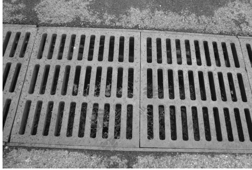
FIGURE 5.4 Grates on a sand filter, unmaintained. (Photo by the author.)
