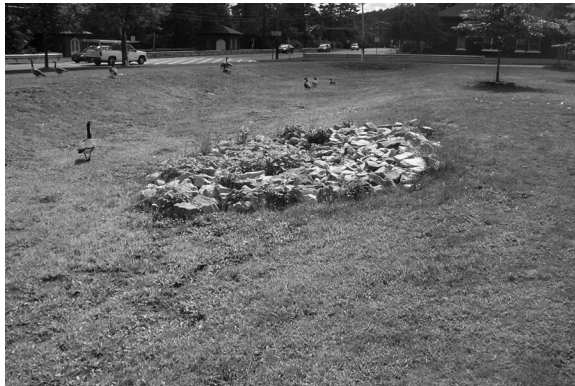
FIGURE 8.40 Another view of lawn depression (a simple, inexpensive rain garden).
