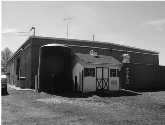
FIGURE 10.7 Rain tank at public works building in Clark, New Jersey. (Photo by the author, 2014.)
