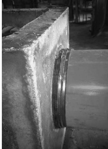
FIGURE 9.18 Cast-A-Seal, boot-type pipe to structure connector. (Made by Press-Seal Gasket Corp.)
