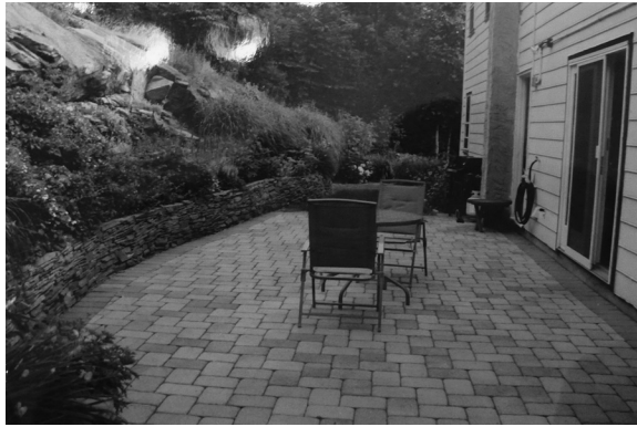
FIGURE 8.47 Raised planter for capturing runoff from uphill area; author's former residence.
