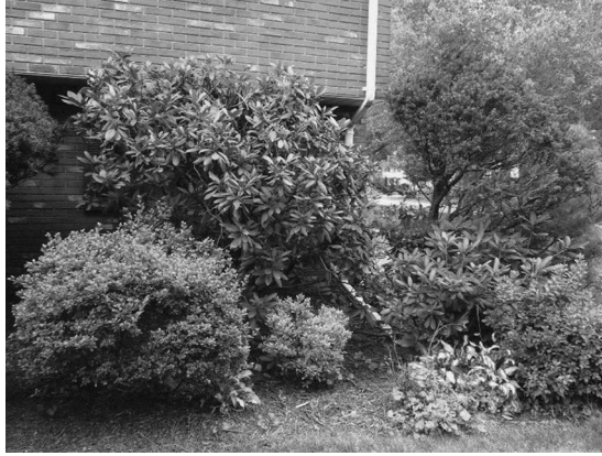
FIGURE 8.46 Roof leader terminating at landscaping at author's residence.
