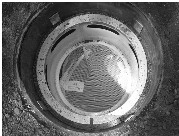
FIGURE 6.4 Lawn inlet screen filter.
