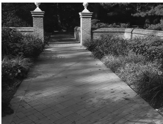
FIGURE 8.14 Pavers at a sidewalk in Van Saun Park in Paramus, New Jersey. (Photo by the author.)
