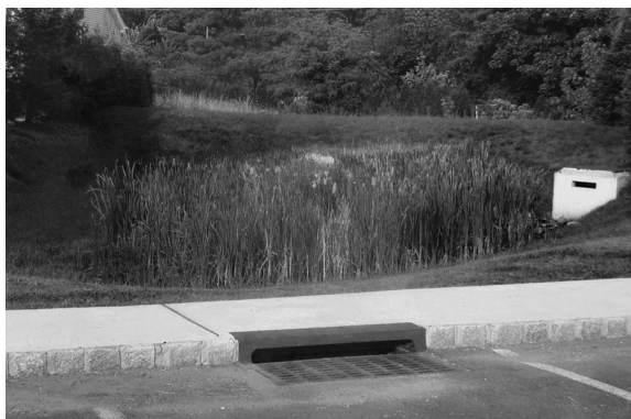
FIGURE 9.21 A detention basin covered with overgrown vegetation. (Photo by the author.)
