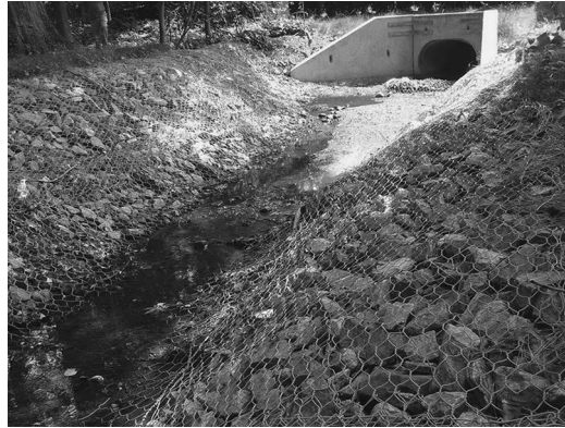
FIGURE 4.48 Reno mattress covering stream banks. (Photo by the author.)
