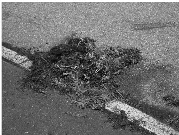
FIGURE 9.31 Street dirt from 100 ft of curbside. (Photo by the author.)
