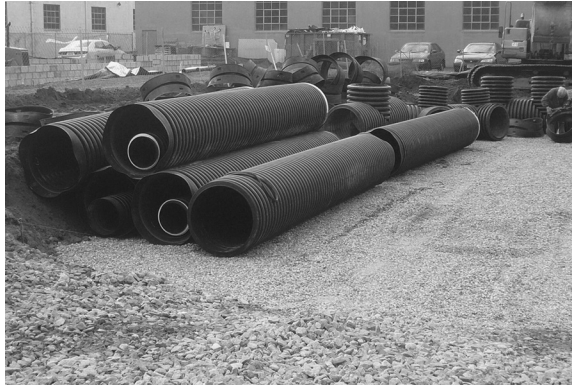
FIGURE 9.7 Stacked 24 in. solid HDPE pipes.
