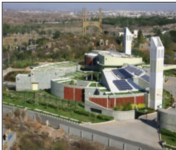
Fig. 6 CII-Sohrabji Godrej Green Business Centre. Source http://www.greenroofs.com/content/guest_features005.htm
