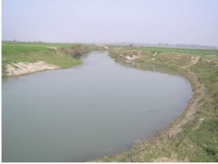
Drain No. 8: Wazirabad barrage gets water through Storm Water Drain (No. 8) via Palla [pH = 7.49, EC = 20]µmhos/cm, TDS = 120.6 mg/l, Turbidity = 8.5 NTU, NH 4 = 0 mg/l, BOD = 2.0 mg/l, TC = 500 MPN/100ml, FC = 450, DO = 8.3 mg/l]
