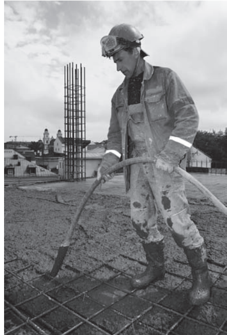
FIGURE 7.13 Consolidating concrete with an internal vibrator. (Shutterstock/Dmitry Kalinovsky)
