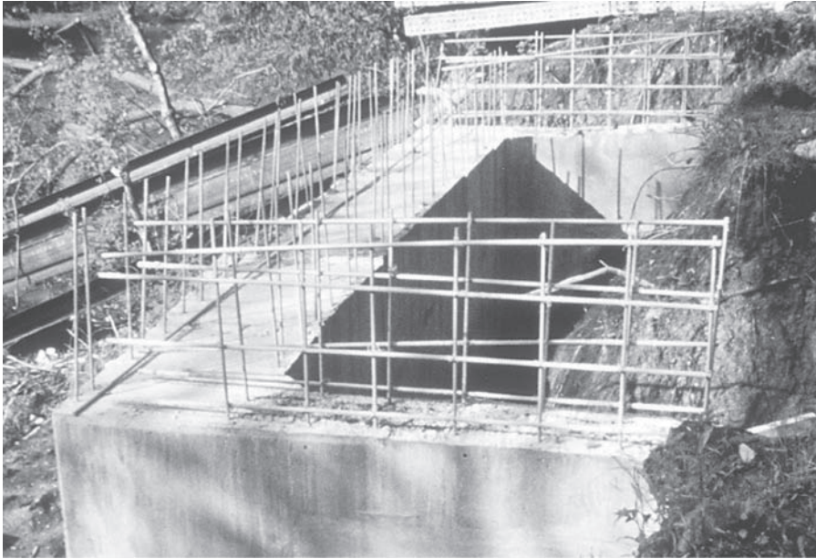
FIGURE 11.1 FRP reinforcing bars used for bridge abutment. (Courtesy of West Virginia University Constructed Facilities Center)
