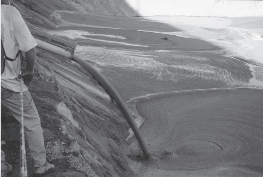
FIGURE 7.45 Filling a sink hole with flowable fill.
