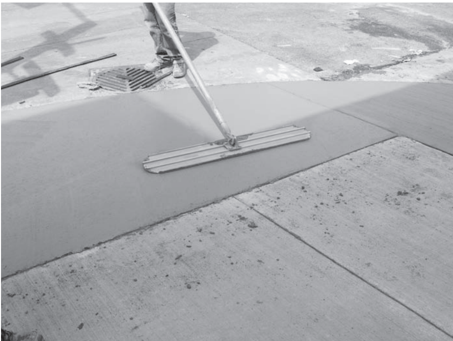
FIGURE 7.19 Finishing concrete manually with a straightedge. (Fotolia/alisonhancock)
