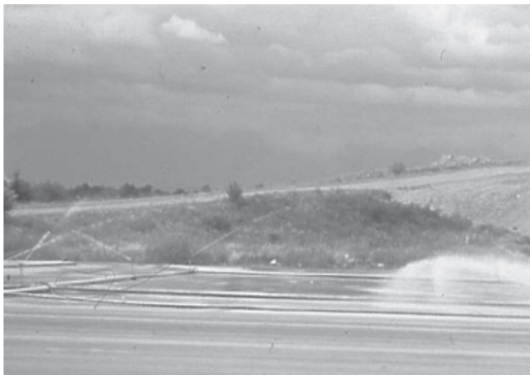
FIGURE 7.25 Curing concrete by spraying. (Courtesy of FHWA)
