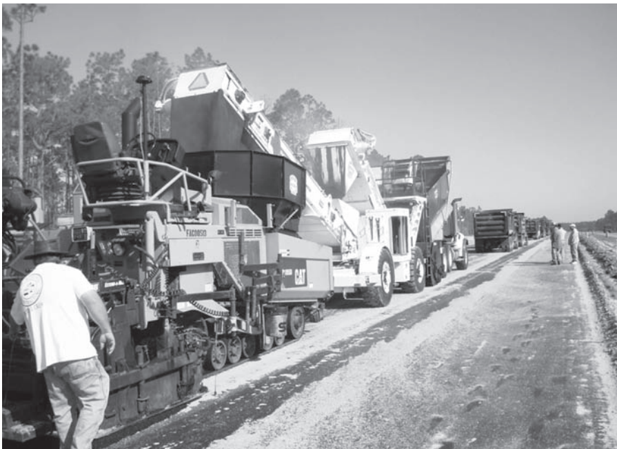
FIGURE 9.40 Material transfer devices used to transfer the asphalt concrete from the trucks to the paver.
