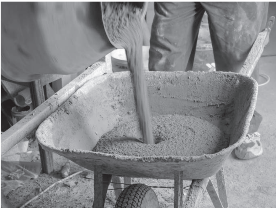
FIGURE 7.7 Loading concrete in a wheelbarrow. (Fotolia/Laure F)
