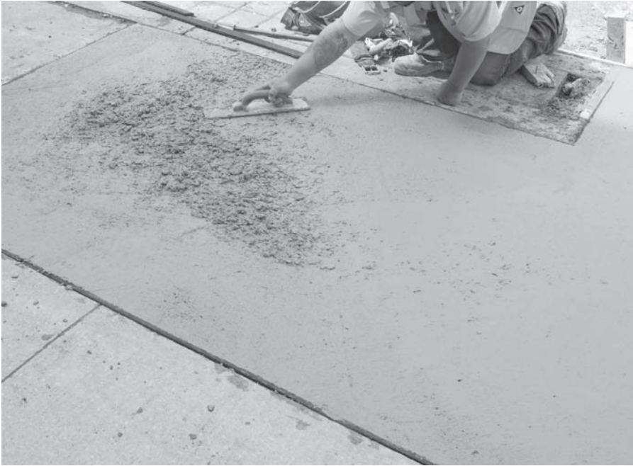
FIGURE 7.18 Finishing concrete with a trowel. (Fotolia/alisonhancock)
