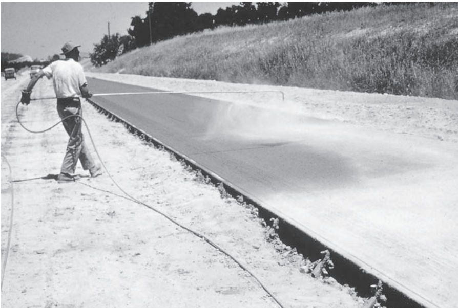
FIGURE 7.30 Curing concrete by manually applying membrane forming compound.
