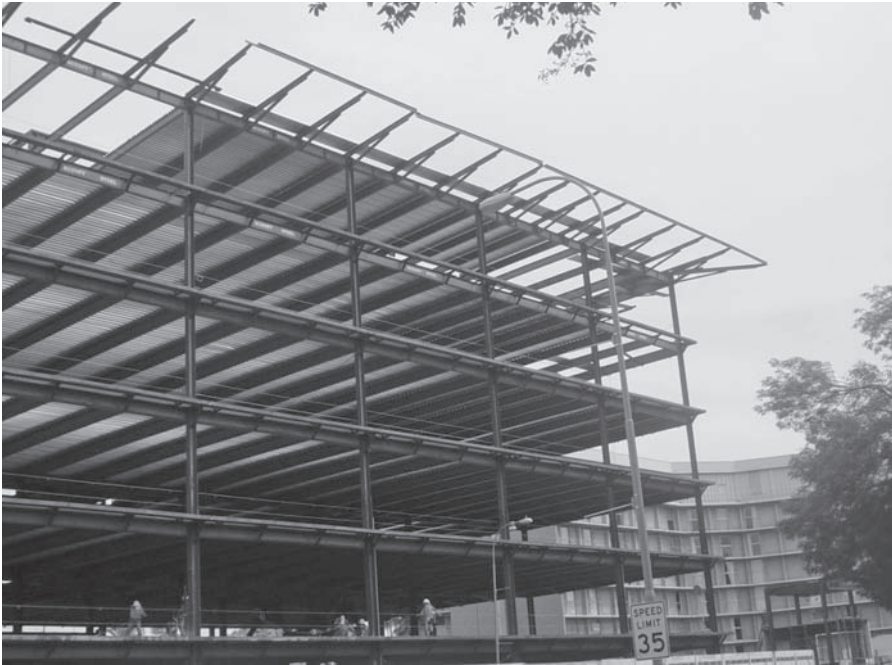
FIGURE 3.8 Structural and cold-formed steel used to make columns, beams, and floors for the structural support of a building.
