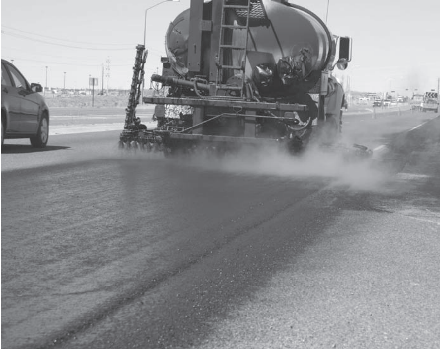
FIGURE 9.8 Spraying tack coat (emulsion) on existing asphalt pavement before placing an asphalt overlay. (Courtesy of FHWA)
