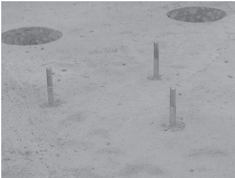
FIGURE A.49 Three probes driven into concrete.
