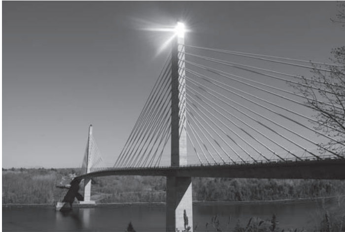
FIGURE 11.8 Retrofit bridge cables made of carbon fiber reinforced polymer. (Penobscot Narrows Bridge and Observatory, Maine) (Fotolia/Chris Soucy)
