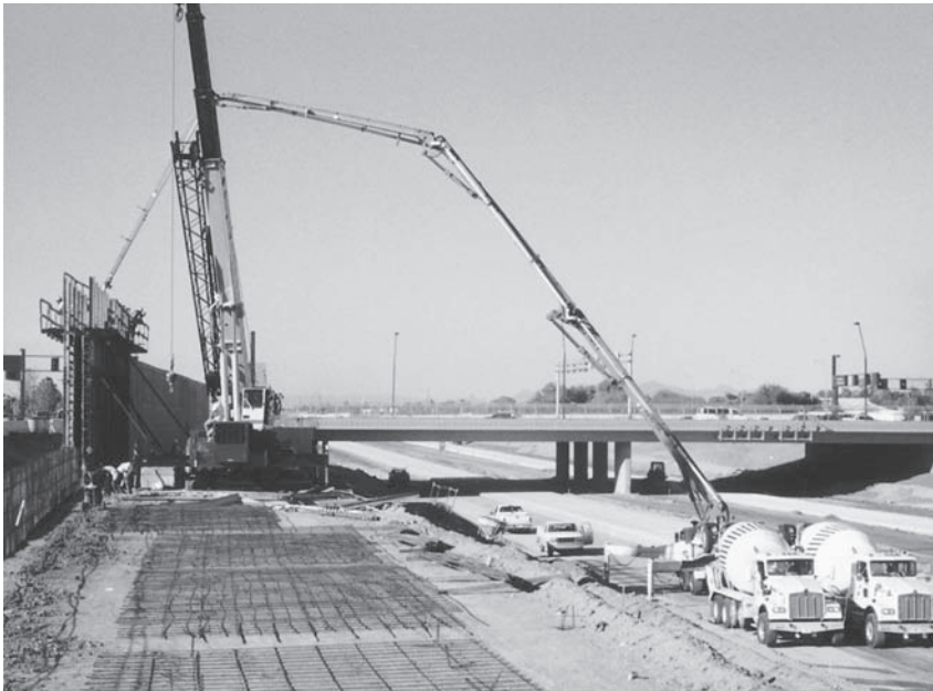
FIGURE 7.12 Pumping concrete in a retaining wall.
