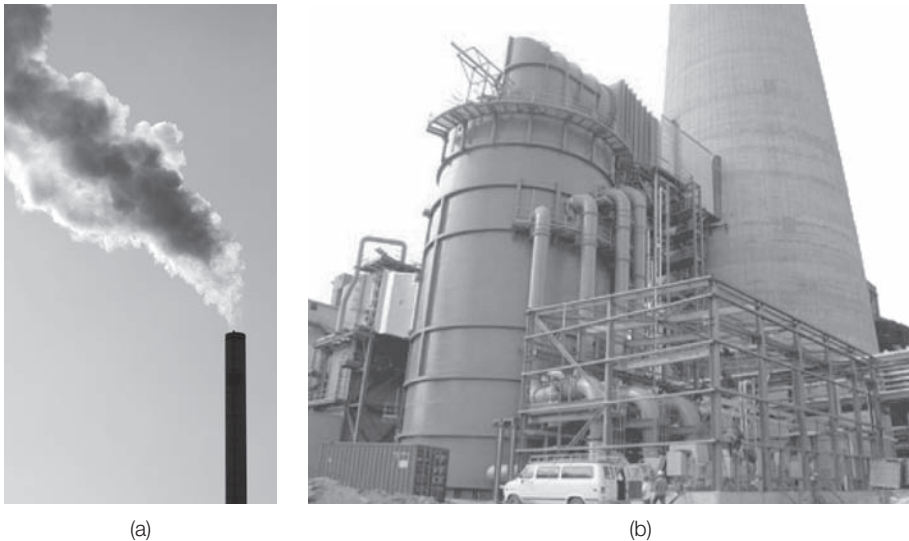
FIGURE 6.13 Fly ash resulting from the combustion of ground or powdered coal (a) being discharged from a coal fired electric plant before environmental regulations were put into effect (Fotolia/manfredxy) and (b) collected into a bag house.
