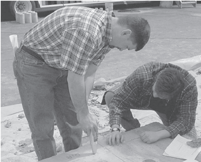
FIGURE A.46 Testing concrete slab with a rebound hammer.
