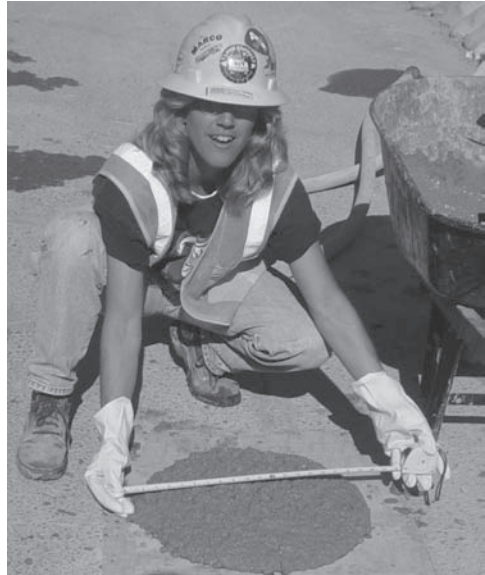
FIGURE 7.44 Measuring the spread during the slump flow test.
