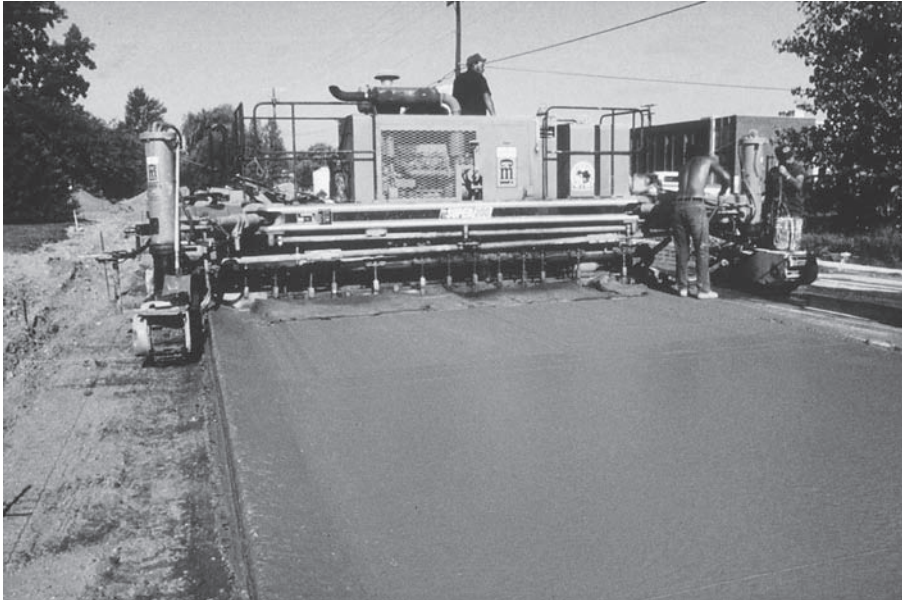
FIGURE 7.10 Placing concrete pavement with a slip-form paver.
