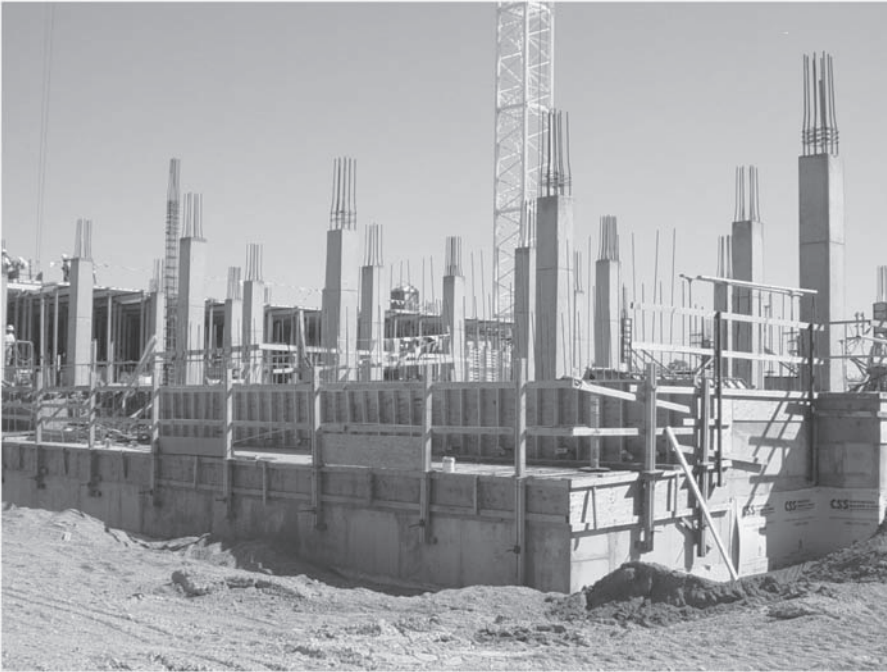
FIGURE 3.13 Steel rebar used to reinforce PCC columns.
