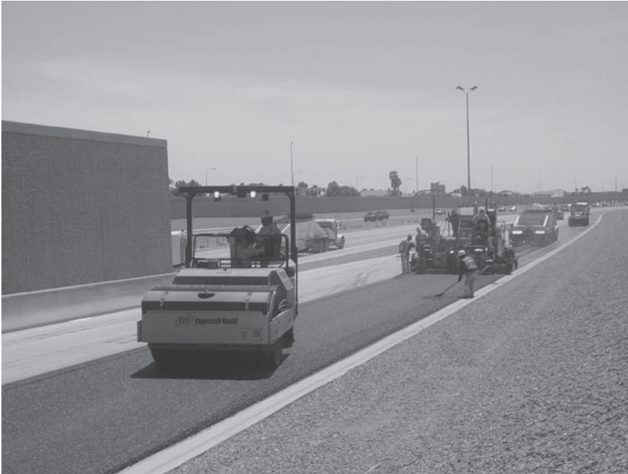
FIGURE 9.6 Compaction of asphalt concrete.
