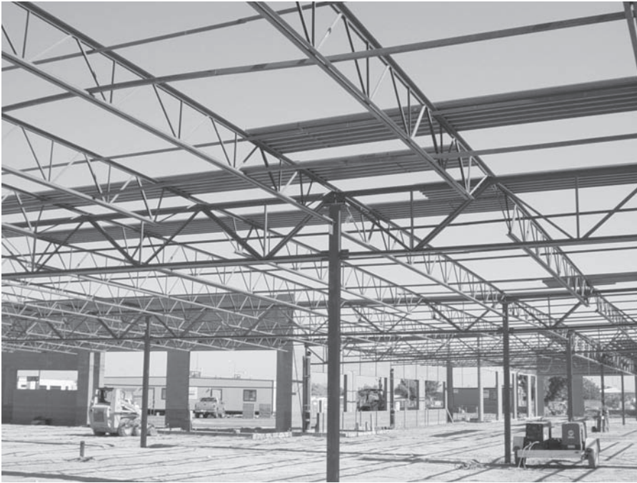
FIGURE 3.1 Steel trusses and columns for the structural support of a building.
