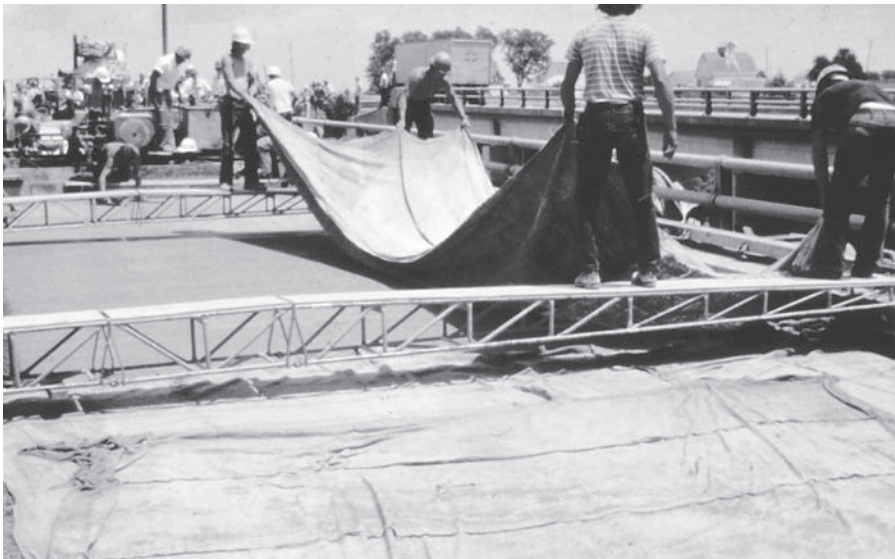
FIGURE 7.28 Curing concrete with impervious fabrics.
