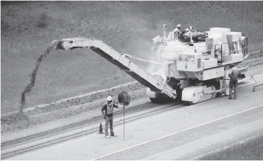
FIGURE 9.41 Milling old pavement.
