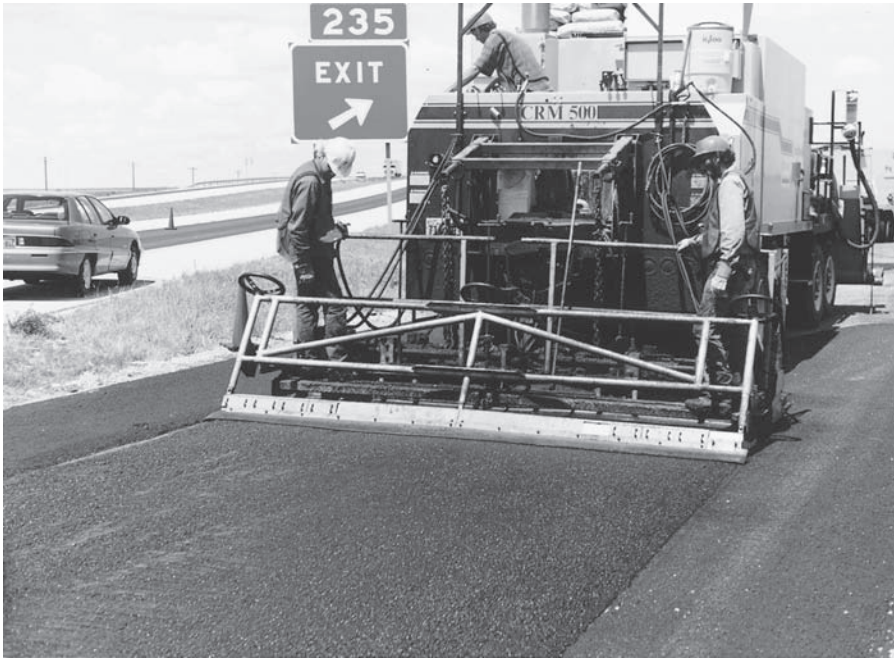
FIGURE 9.10 Applying microsurfacing for preserving existing pavement. (Courtesy of FHWA)
