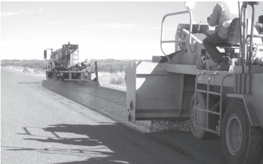
FIGURE 9.9 Applying chip seal (emulsion followed by aggregates) for preserving existing pavement. (Courtesy of FHWA)
