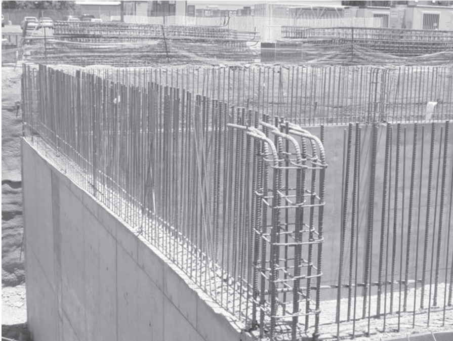
FIGURE 3.2 Steel rebars used to reinforce portland cement concrete wall.
