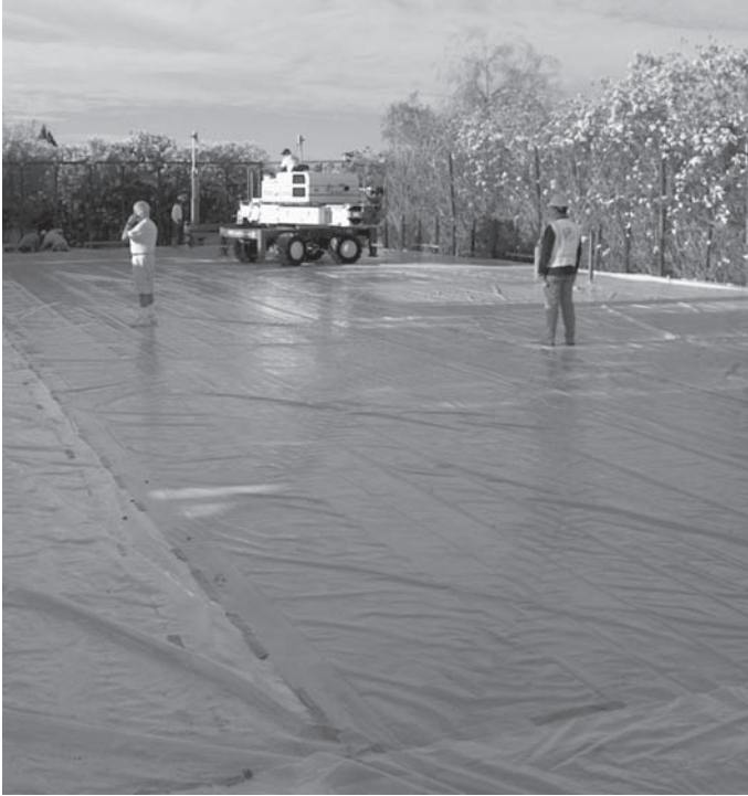
FIGURE 7.29 Curing concrete with plastic sheets.
