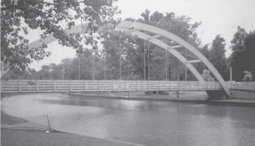
FIGURE 10.7 An arch bridge made of structural glued laminated timber (glulam). (Courtesy of the American Institute of Timber Construction)
