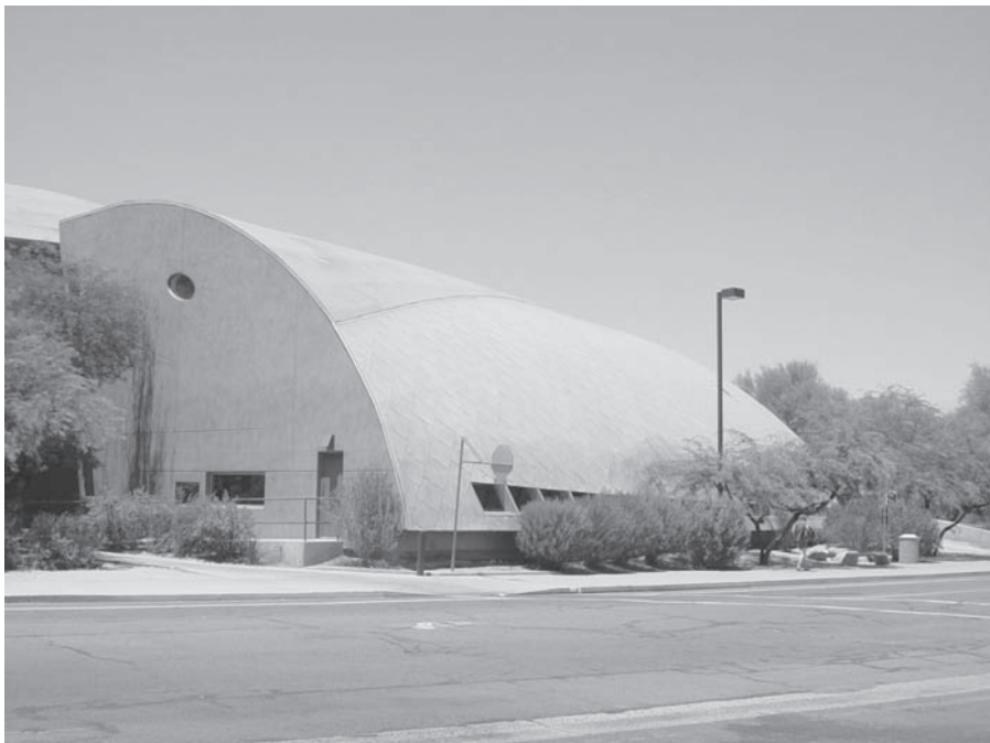
FIGURE 4.2 Building facade made of aluminum.
