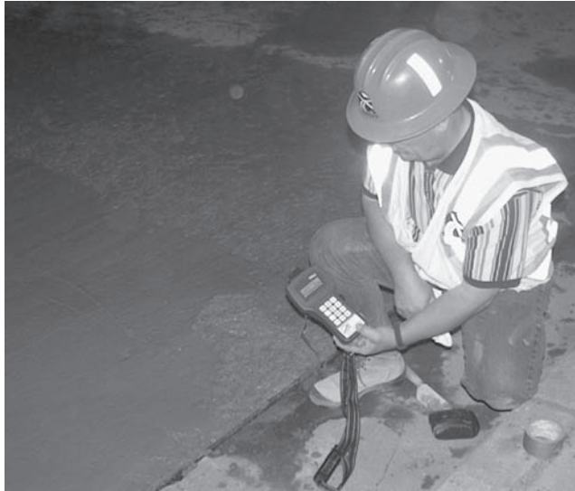
FIGURE 7.42 Checking the maturity of fresh concrete using the maturity meter.
