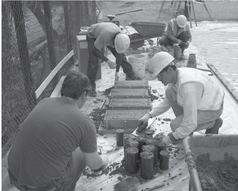
FIGURE A.36 Making concrete cylinders and beams.
