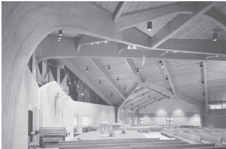
FIGURE 10.6 Frames made of structural glued laminated timber (glulam). (Courtesy of the American Institute of Timber Construction)
