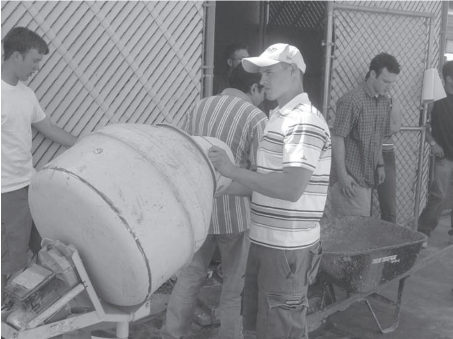
FIGURE A.30 Mixing concrete in a mixer.
