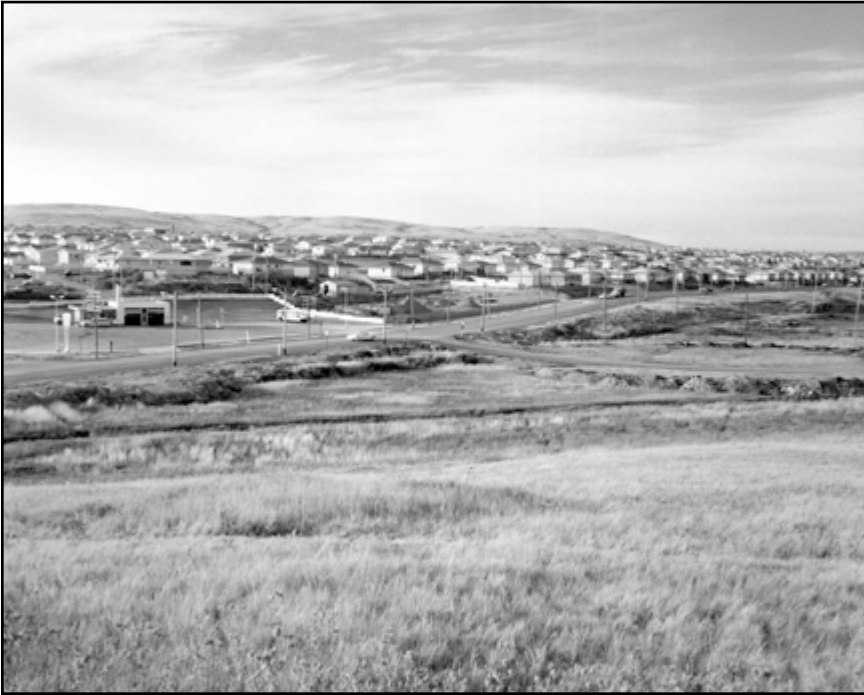
North Mount Pleasant subdivision under construction, 1958.
