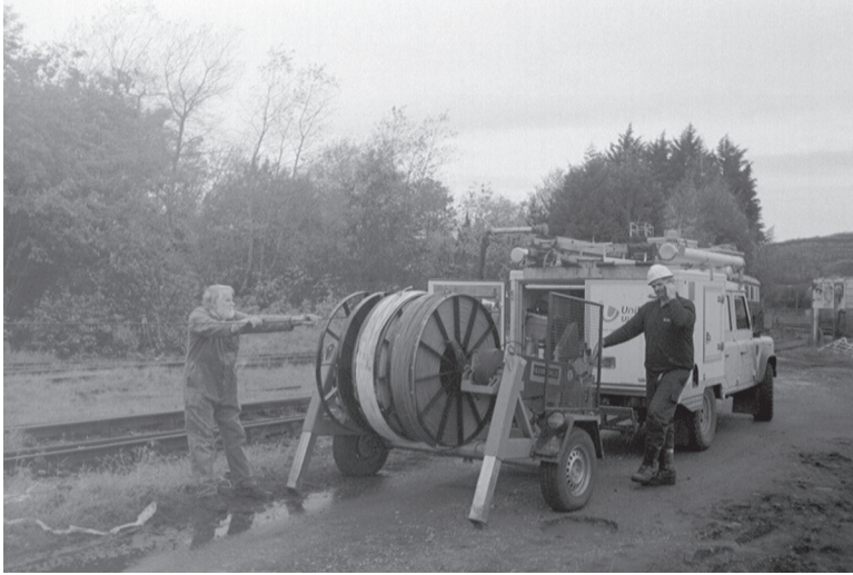
Figure 4.42 Running out the OHL (Photo: L. Lesley)
