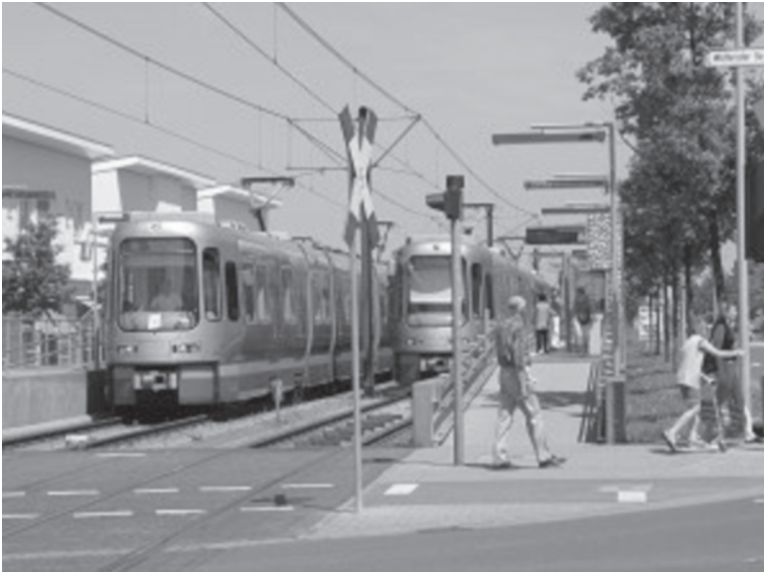
Figure 4.2 High platform in street of Hannover, Germany (Photo: Urbanrail.net)
