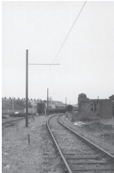
Figure 4.39 Cable-stayed side bracket arms in Carnforth (Photo: L. Lesley)
