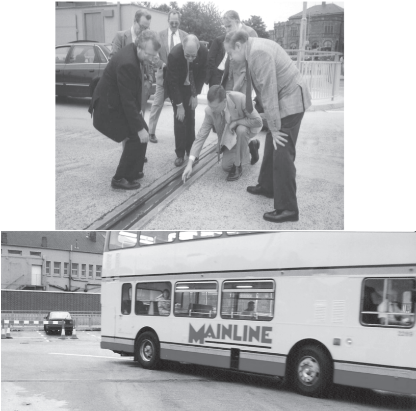
Figure 4.11 Rotherham Bus Station LR55 installation (Photos: L. Lesley)
