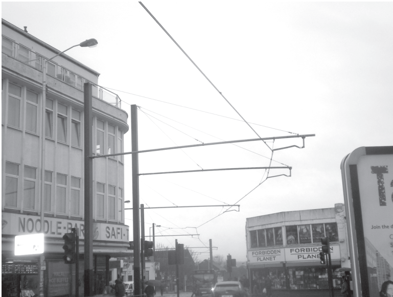
Figure 4.4 Croydon heavy OHL masts (Photo: L. Lesley)
