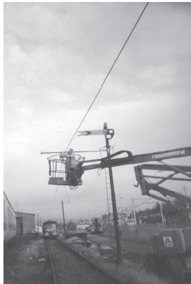
Figure 4.41 “Cherry picker” used for OHL installation (Photo: L. Lesley)
