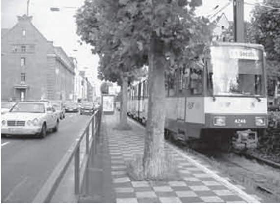
Figure 4.55 Long platforms for light rail two-car consists in Dusseldorf (Photo: City Transport Information)
