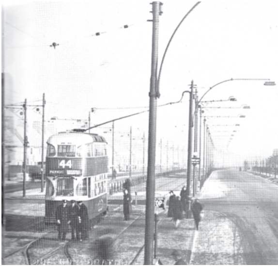
Figure 4.40 Shared traction and lighting poles in Liverpool, 1938 (Photo: Liverpool City Engineer)
