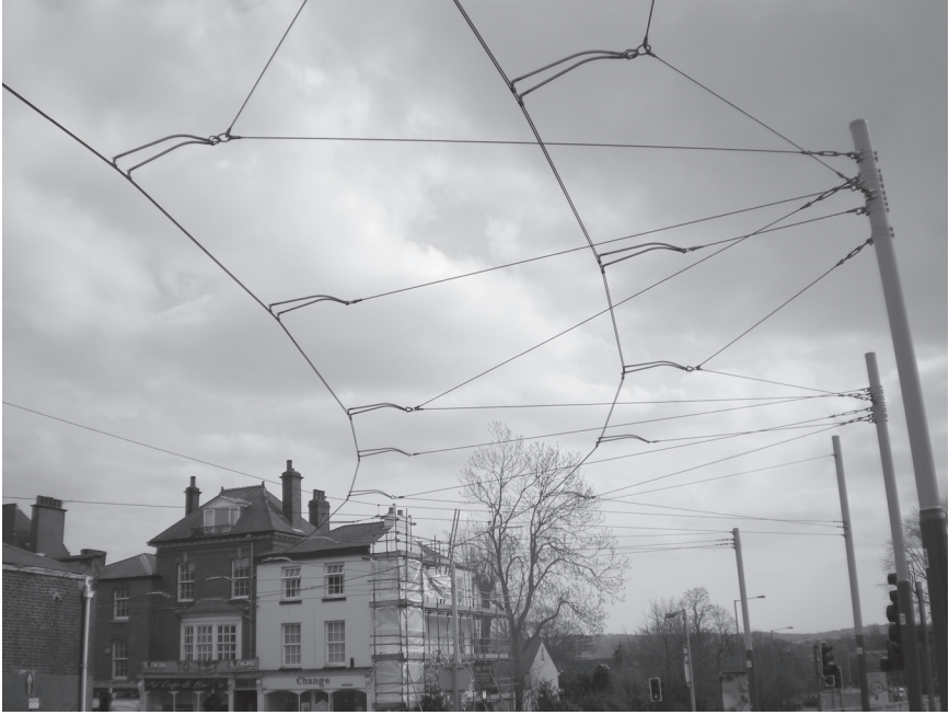
Figure 4.29 Aligning OHL over curved track in Sheffield, 2008 (Photo: L. Lesley)
