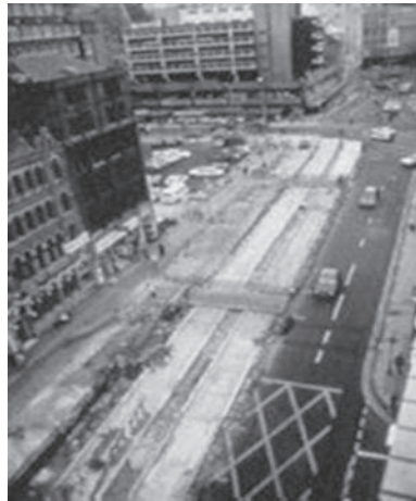
Figure 2.8 Manchester track slab, Market Street, 1990 (Photo: L. Lesley)
