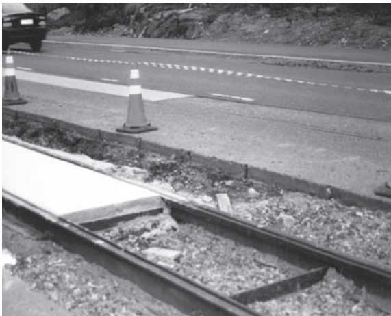
Figure 5.10 Track construction in Helsinki (Photo: M. Bell)
