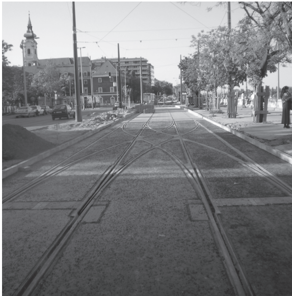
Figure 4.36 Embedded "scissors" crossover in Budapest, 2009 (Photo: L. Lesley)
