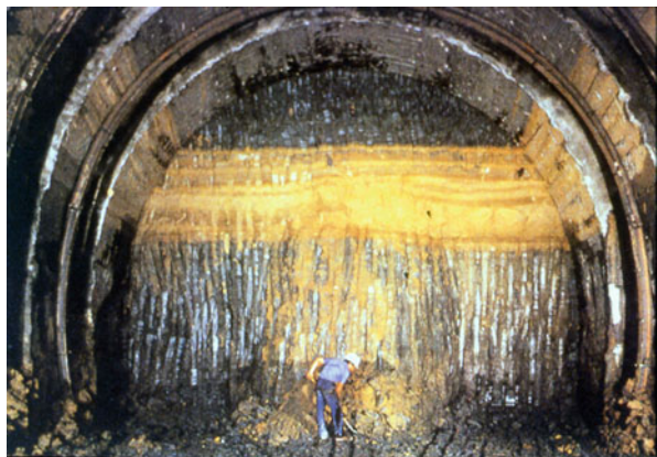
Fig. 6.46 Tunnel excavated with precutting method. (By Rodio)
