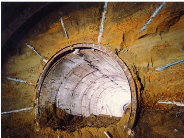
Fig. 6.15 Radial injections from the pilot tunnel using PVC-valved pipes. (By Pizzarotti)
