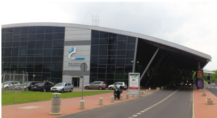
Fig. 5.3 Władysław Reymont Airport in Łódź. Source Author's photograph
