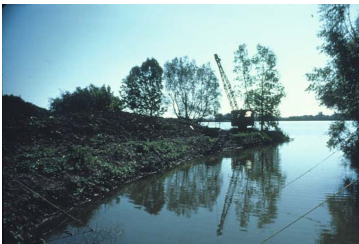
Fig. 7.13 Dredging for marina use. Photo credit: New York Sea Grant
