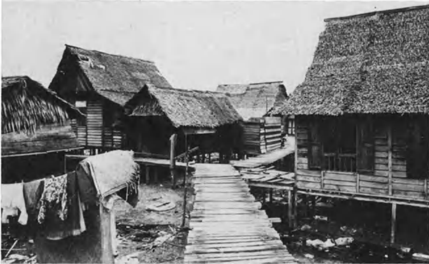
Fig. 3. Kampong Sungei Keladi (control area schemes A and B). A Malay squatter settlement, where the residents have skillfully adapted their housing environment: the entire settlement is built above a shallow creek, which is flooded at high-tide. While Malays traditionally build their houses on stilts (see pictures 7 and 8), the elevated footpaths are a specific feature of this area.
