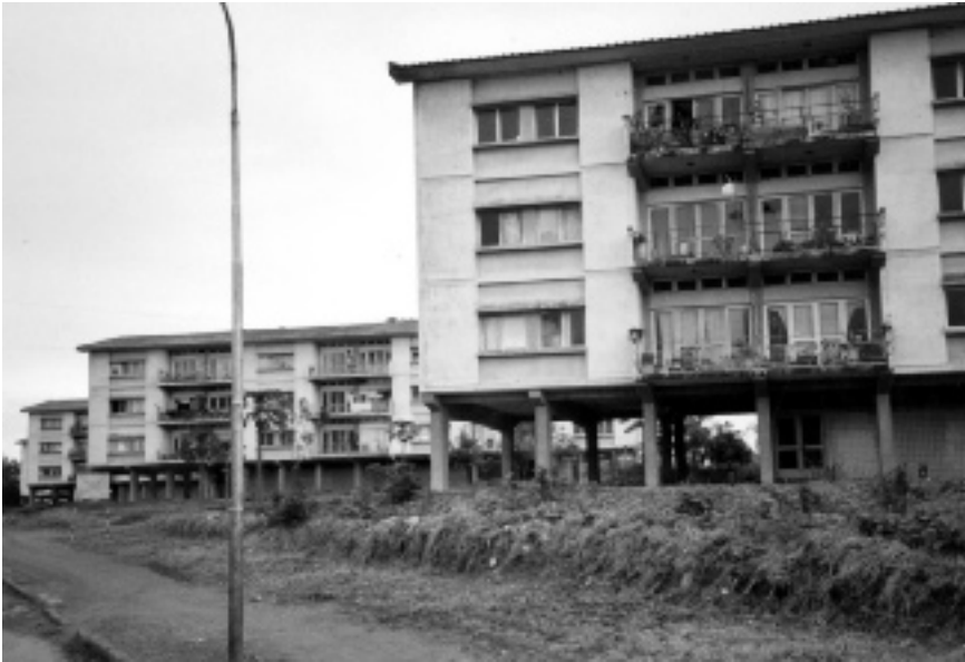
7.2 Modern tenement blocks on the periphery of Huambo, Angola (Harry Smith)
