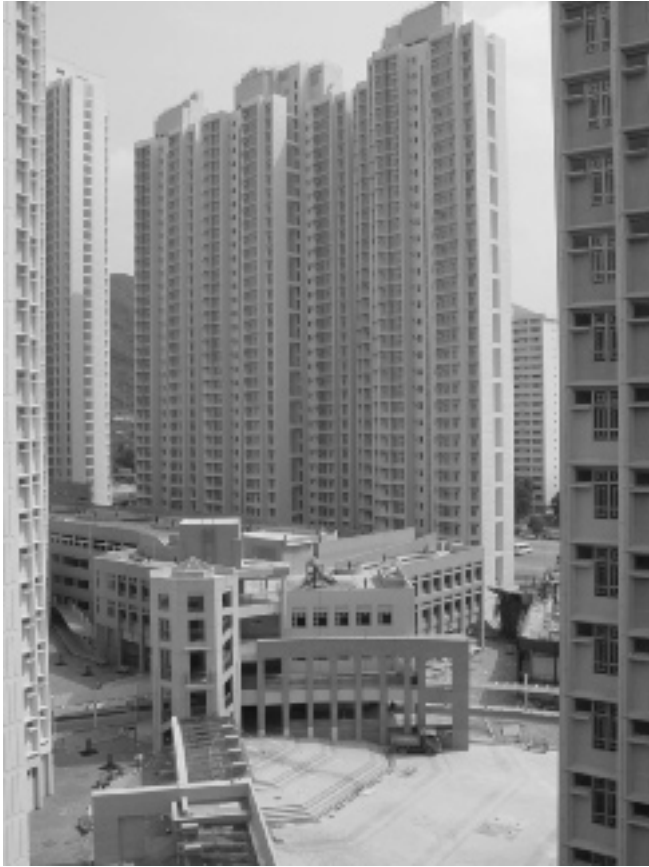
11.6 Hong Kong Housing Authority high-rise housing in Shatin New Town, Hong Kong (Hong Kong Housing Authority)
