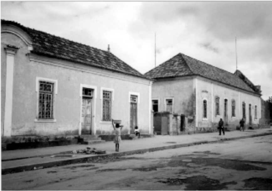
5.6 Portuguese colonial houses in Huambo, Angola (Harry Smith)
