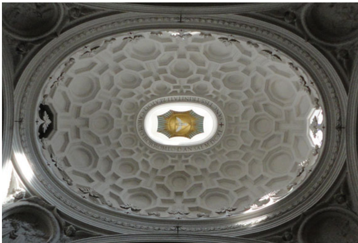
Fig. 7.4 The dome of San Carlino as seen from below. The entrance is to the left ( copyright Sophie Püschmann, with kind permission )
