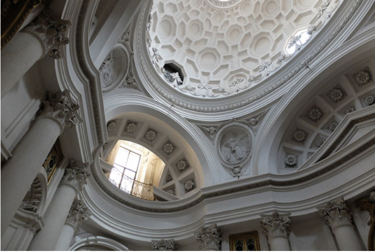
Fig. 7.5 A view of the church from below, at the side of the entrance, including part of the dome and the corresponding supporting arcs and pendentives over the mixtilinear cornice ( copyright Sophie Püschmann, with kind permission )
