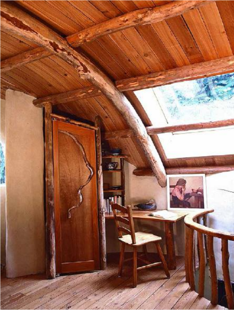
FIGURE 11.1. The varying ceiling height under the arched roof on the second story of Hilda Dawe's cob cottage (built by CobWorks in Canada), lends itself to different kinds of usage in different areas. Against the
