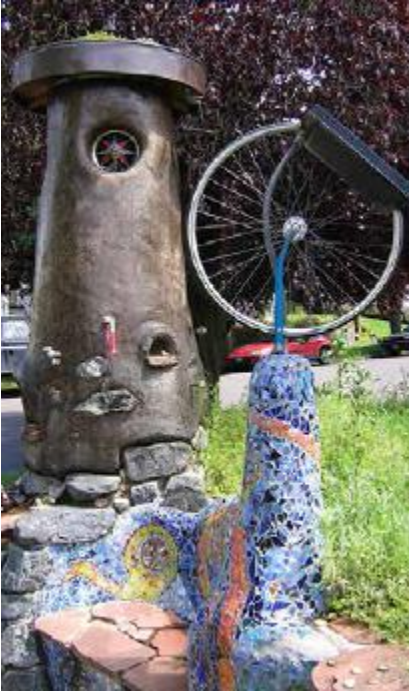
FIGURE 20.3. The Memorial Life-house, conceived as a place of remembrance for a bicyclist killed at this corner. Built of cob, stone and recycled materials, including tricycle wheels with stained glass for windows, a living roof and a solar powered light (note the solar panel attached to the bicycle wheel). [Credit: Joseph F. Kennedy]
