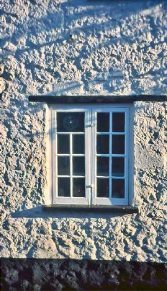
FIGURE 50.1. Traditional house in Beer, England, showing this traditional use of lime and pitch as finishing materials. [Credit: Joseph F. Kennedy]
