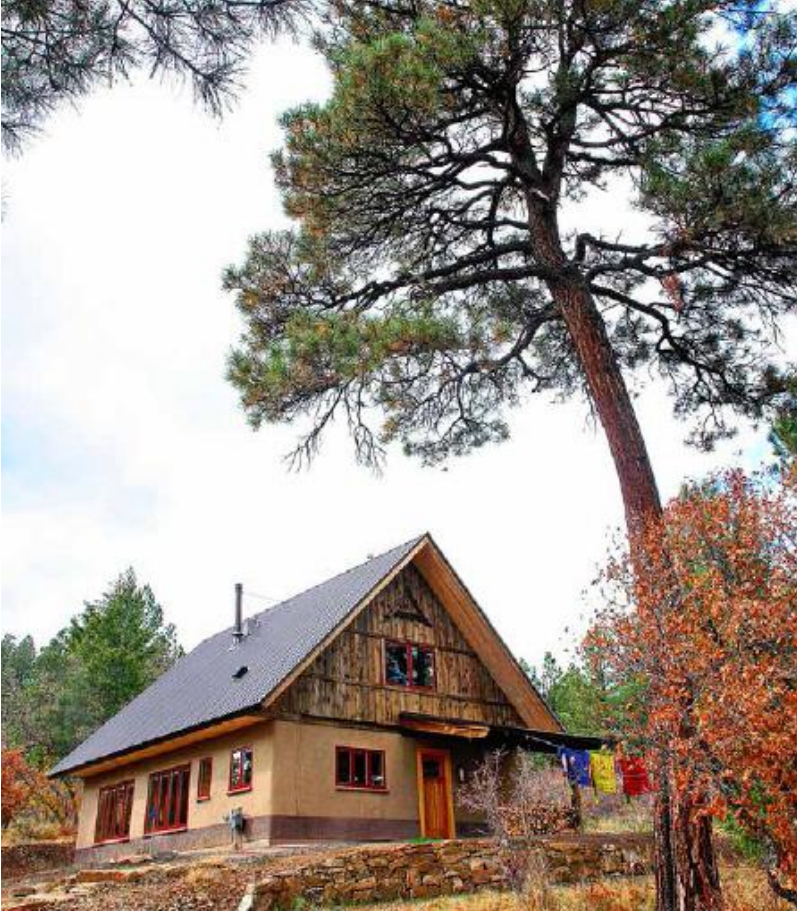
FIGURE 16.3. Large trees near a building site can provide not only cooling shade but also a visual and energetic focal point. This straw bale home in Pagosa Springs, Colorado, was built by Kelly Mathews. [Credit: Catherine Wanek]
