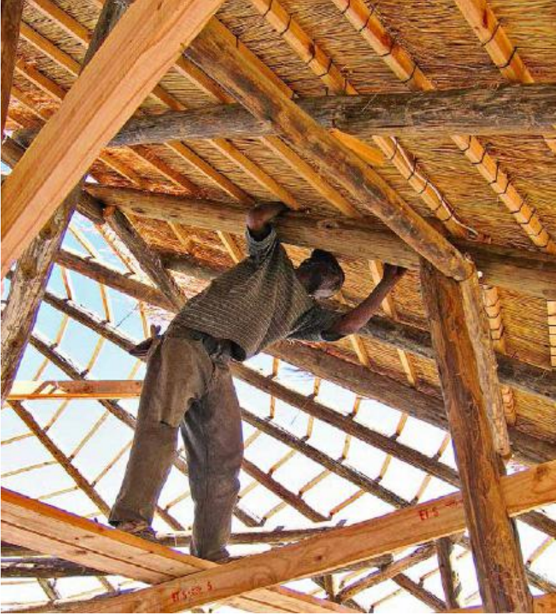
FIGURE 42.5. Thatching a performance space with grass in Dennilton, South Africa. [Credit: Joseph F. Kennedy]
