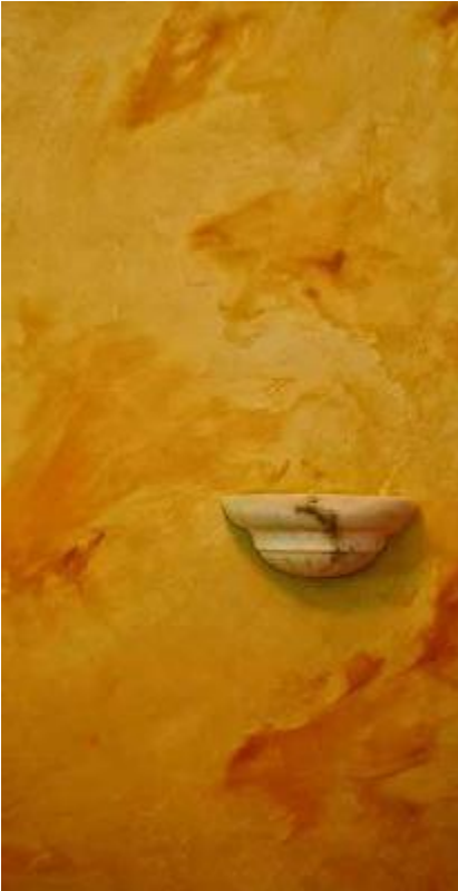
FIGURE 50.5. The color here is actually mixed directly into the plaster and applied by Janine Björnson as part of
