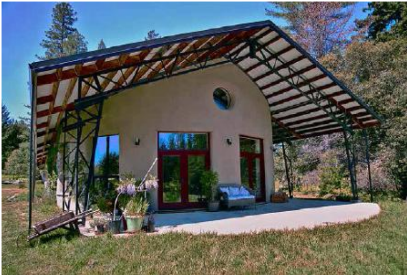
FIGURE 31.2. The wide eaves of this steel-frame structure in rainy northern California shed precipitation far away
