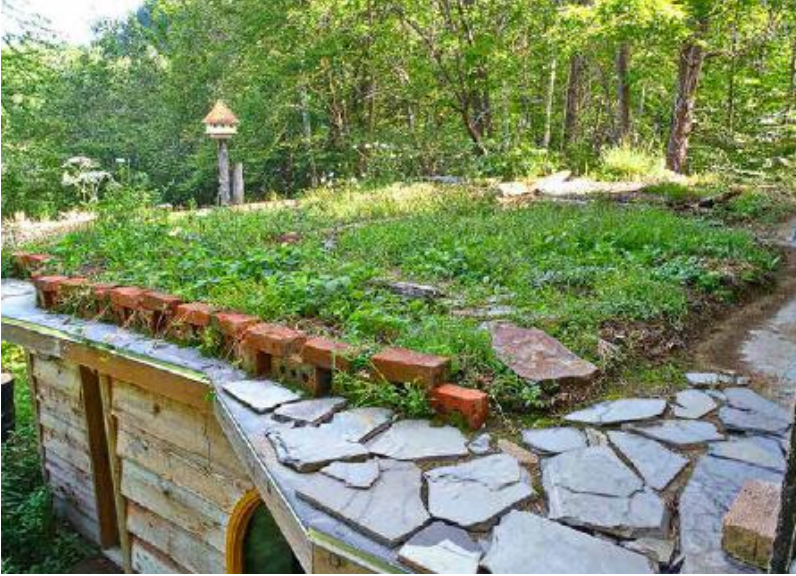
FIGURE 43.4. High-tech or low-tech, urban or rural, a living roof makes use of our rooftops, offering both gardening potential and living space. And it gives a little bit of habitat back to nature. [Credit: Michel Bergeron]
