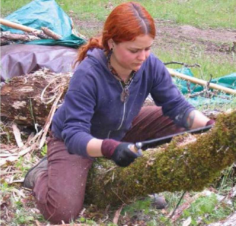
FIGURE 21.4. Using a traditional drawknife to peel the bark from this freshly harvested tree. [Credit: Joseph F. Kennedy]
