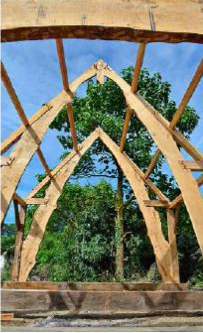
FIGURE 35.3. These full cruck bents of oak were constructed during a 2013 Fox Maple timber-framing workshop in Brittany, France. This was a very early style of bent framing first practiced in medieval Europe. [Credit: Steve Chappell]
