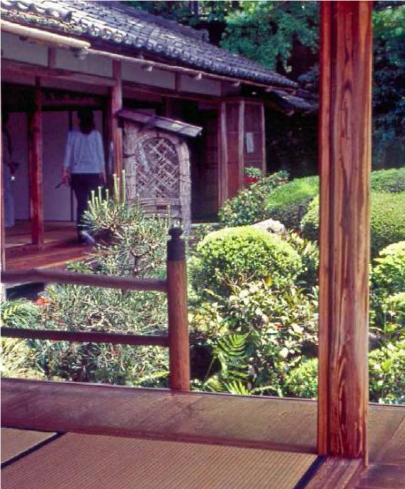
FIGURE 21.7. This traditional house in Japan demonstrates the harmonious juxtaposition of a number of natural building materials, including, wood bamboo, reed mats, earth plasters and clay tiles. [Credit: Joseph F. Kennedy]
