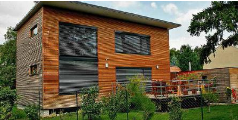
FIGURE 31.9. The challenging energy standards of the German “Passivhaus” concept have been achieved by straw bale architects and builders both in Europe and the
