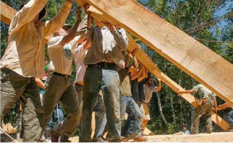
FIGURE 36.8. If executed safely, a hand-raising can be an exhilarating finale to the slow and detailed work of cutting the frame. [Credit: Devin Smith]
