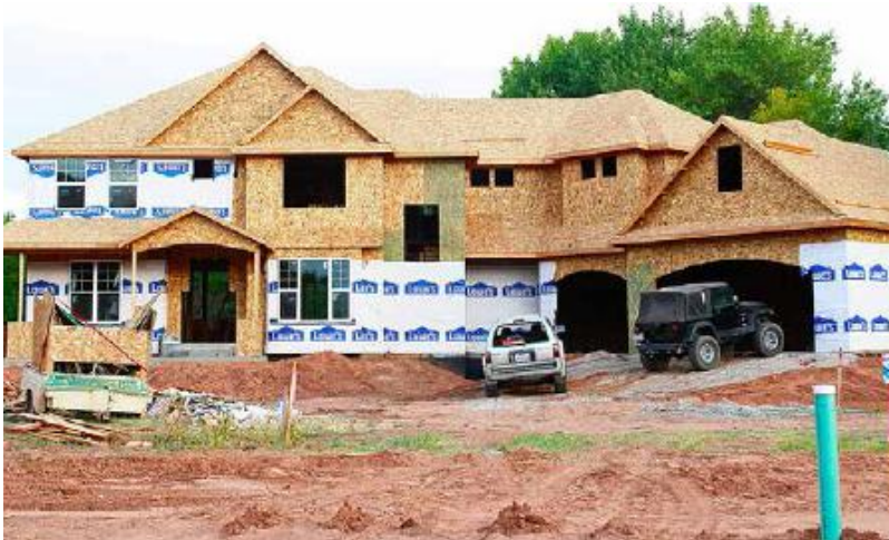
FIGURE 7.1. Conventional construction, Moab, Utah. [Credit: Catherine Wanek]
