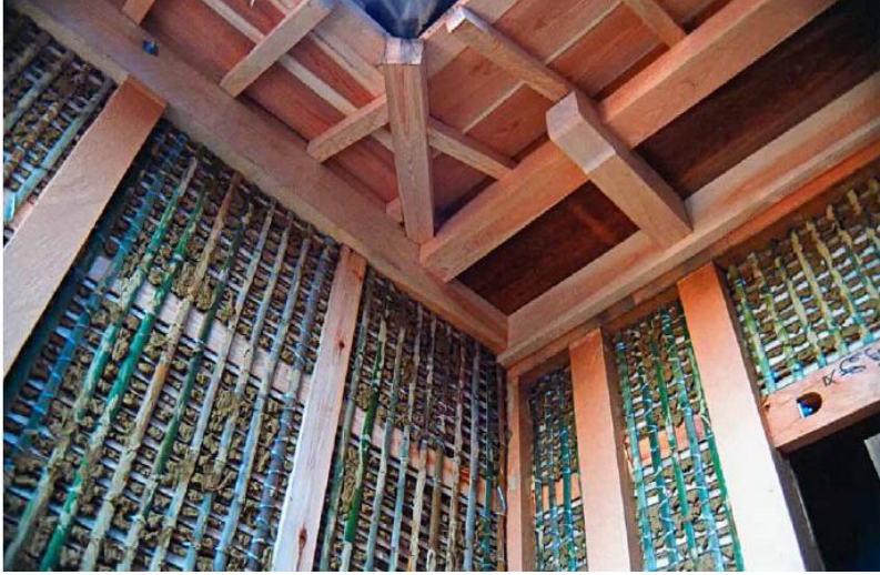
FIGURE 34.2. Bamboo lath between timber frame walls supports mud daub in this Japanese structure. [Credit: Tom Lander]
