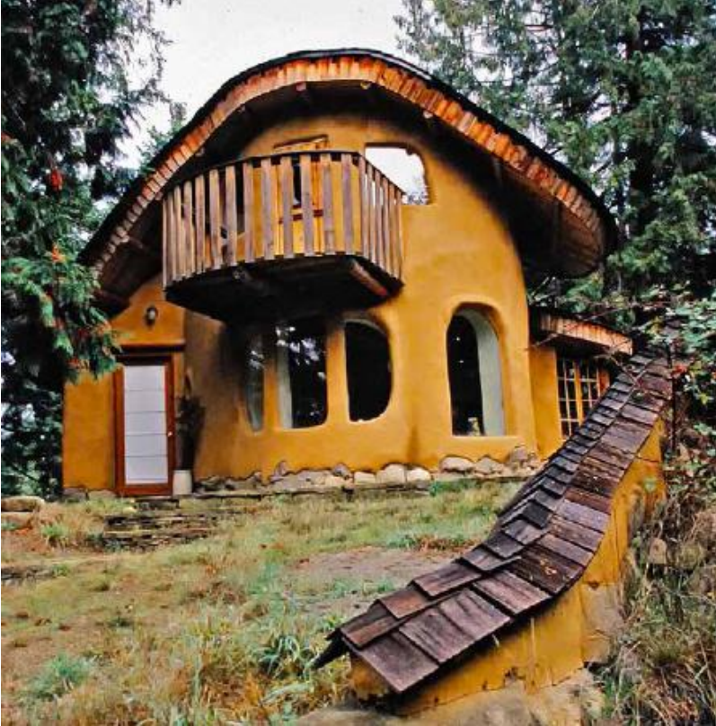
FIGURE 25.6. Hilda Dawe's cob home in British Columbia, Canada, designed and built by Cobworks, demonstrates the sculptural potential of Oregon cob. [Credit: Catherine Wanek]
