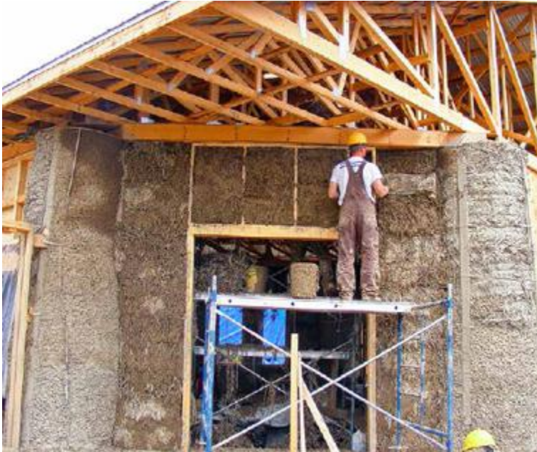
FIGURE 32.9. Standard-size hemp bales are used to infill between the round bale structural columns. Chopped hemp was also incorporated into the plasters, and into the hempcrete used in the walls and foundation. [Credit: Chris Magwood]
