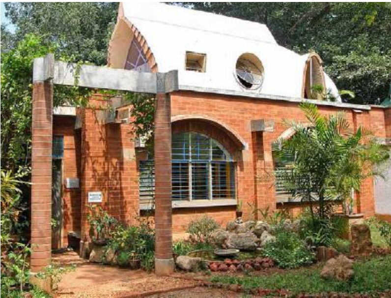
FIGURE 62.1. Office of the Auroville Earth Institute. [Credit: Serge Maïni]
