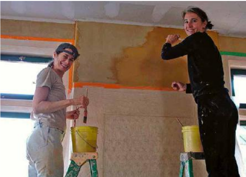
FIGURE 50.2. Applying a clay paint to a straw bale house. [Credit: Courtesy Janine Björnson]
