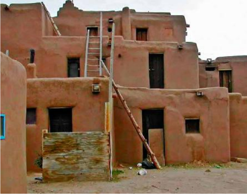
FIGURE 24.1. Taos Pueblo, the oldest continually inhabited settlement in North America, is made largely of adobe. [Credit: Mark Mazziotti]
