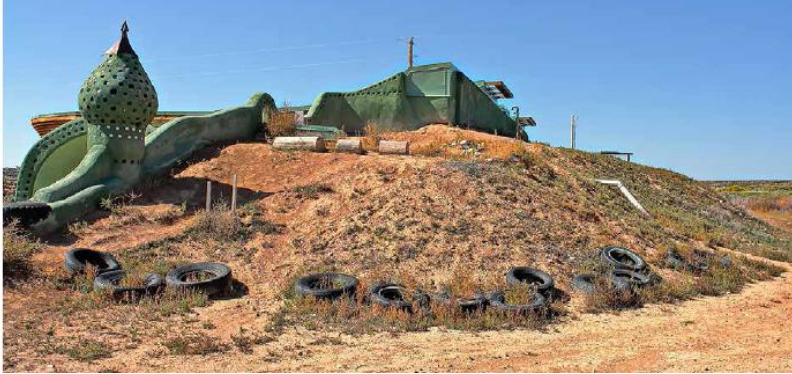
FIGURE 29.3. “Earthships,” a building system developed by Michael Reynolds in Taos, New Mexico, are U-shaped structures made primarily of earth-filled tires, open to the sun on the south side and dug into a hill or covered with earth on the north side. [Credit: Catherine Wanek]
