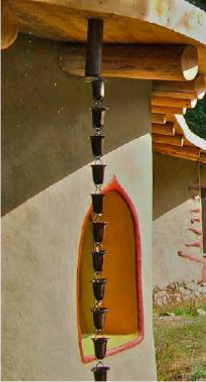
FIGURE 18.6. Water collection and storage don't have to be ugly. This pleasing “rain chain” collects rain from the living roof of a cob building at OUR Ecovillage in British Columbia, Canada. [Credit: Misha Rauchwerger]
