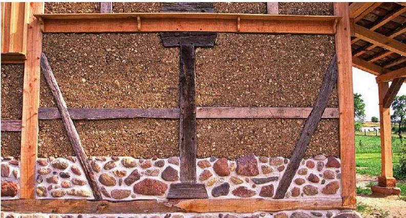
FIGURE 33.5. Straw light-clay provides good insulation, making it appropriate even in cold climates. This small house built by EcoNest Co. awaits its exterior plaster. [Credit: Michael G. Smith]
