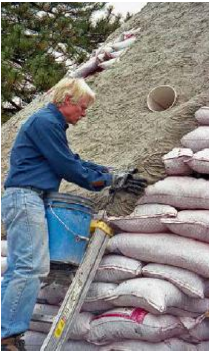
FIGURE 41.6. Kelly Hart used a standard papercrete mixture to plaster his earthbag dome house (see “Digging in for Comfort,” p. 211) in arid Colorado. The papercrete was able to absorb all of the rain falling on the building
