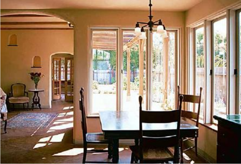
FIGURE 12.1. The basic components of passive solar design are orientation, insulation, glass and mass. In this straw bale home designed by Kelly Lerner, home, south- and east-facing windows let the sun shine in, and the solar heat is absorbed directly into the concrete (mass) floors, and indirectly into the wall plaster. [Credit: Catherine Wanek]
