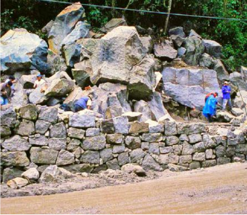
FIGURE 23.4. A road-building crew at work near Machu Picchu in Peru. With enough persistence, human power and hand tools can shape and move even this extremely hard granite. [Credit: Michael G. Smith]
