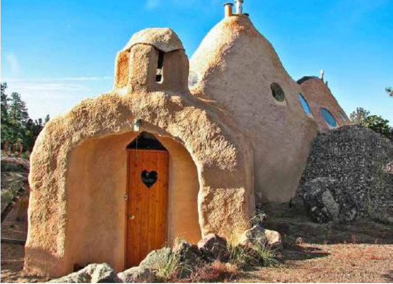
FIGURE 29.2. In the foreground is the vaulted entry to Kelly and Rosana Hart’s earthbag house. Further back, you can see the earth-bermed north side of the house, including the underground pantry dome. [Credit: Kelly Hart]
