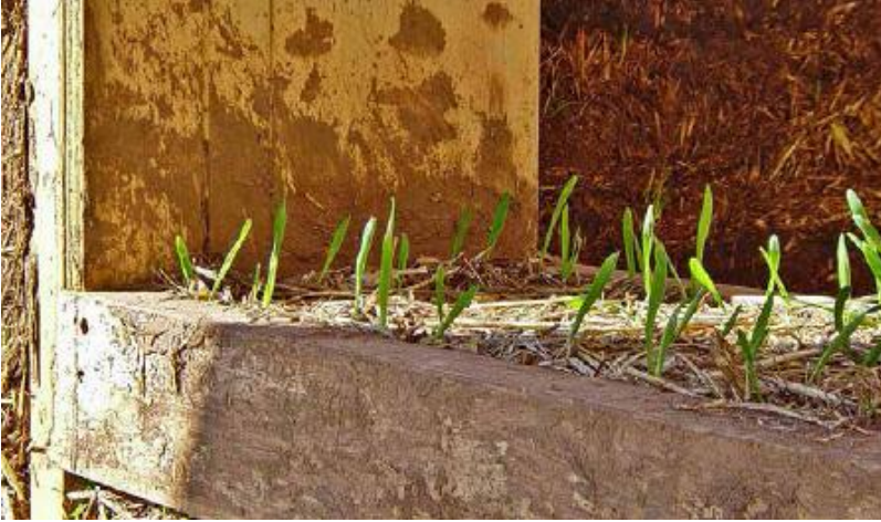
FIGURE 33.2. Seeds in the straw sprout as the wall dries. This is a wonderful example of synergy when working with nature. The sprouts help the wall to dry out. Once the walls are dry enough to plaster, the sprouts will die. Their roots will help bind the wall, while the dead sprouts create extra tooth for anchoring the plaster. [Credit: EcoNest Co]
