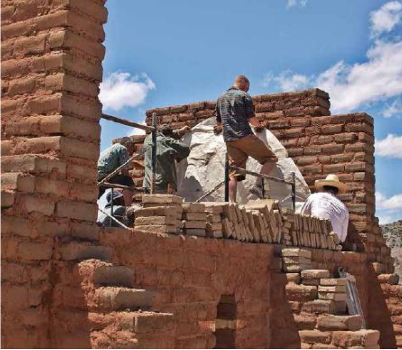
FIGURE 24.5. In Abiquiu, New Mexico, students prepare to build a vault of small adobe bricks, examples of which can be seen stacked on the walls built of traditional adobe blocks. [Credit: Kurt Gardella]
