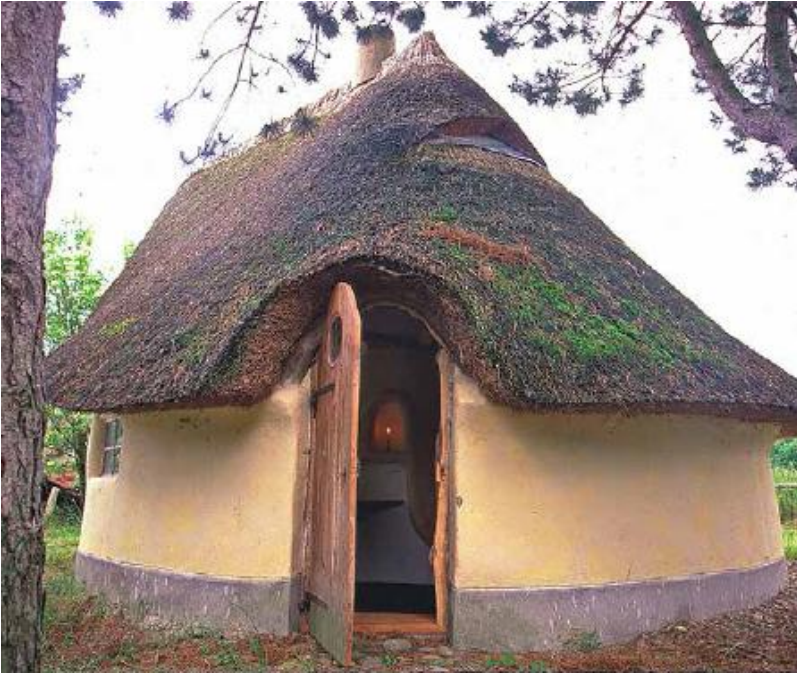
FIGURE 44.5. Flemming Abrahamsson's architectural studio in Denmark, built of cob with a reed thatched roof. The thickness of the thatching provides good insulation for cold winter climates. [Credit: Catherine Wanek]
