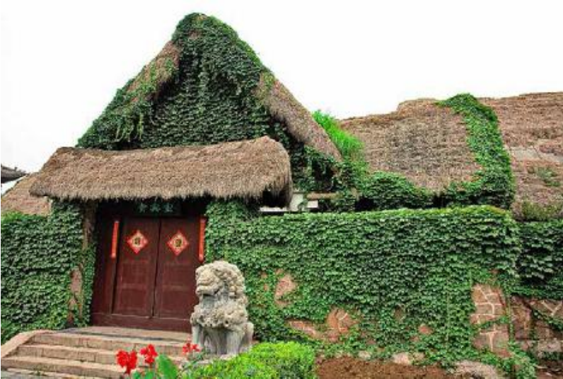
FIGURE 42.7. This thatched roof in China, made from seaweed, could last 80 years or more. It is slowly being colonized by growing plants. [Credit: Catherine Wanek]
