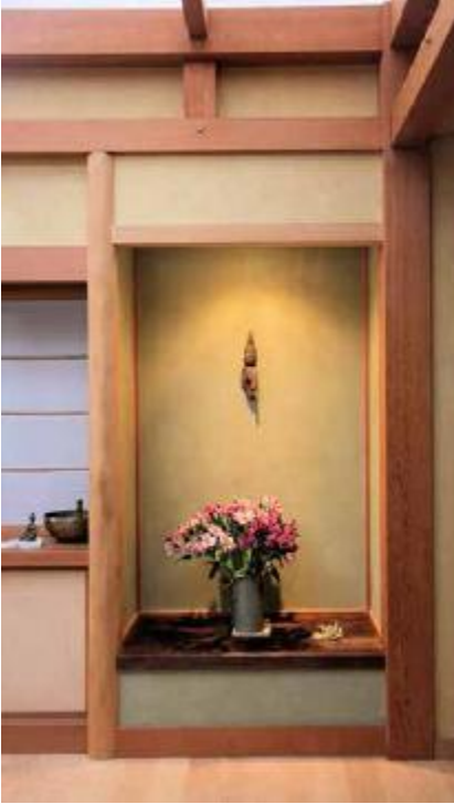
FIGURE 8.1. Finely detailed plaster meets exquisitely crafted timber frame in this “Econest” by builder Robert Laporte and architect Paula Baker-Laporte. [Credit: Paula Baker-Laporte]
