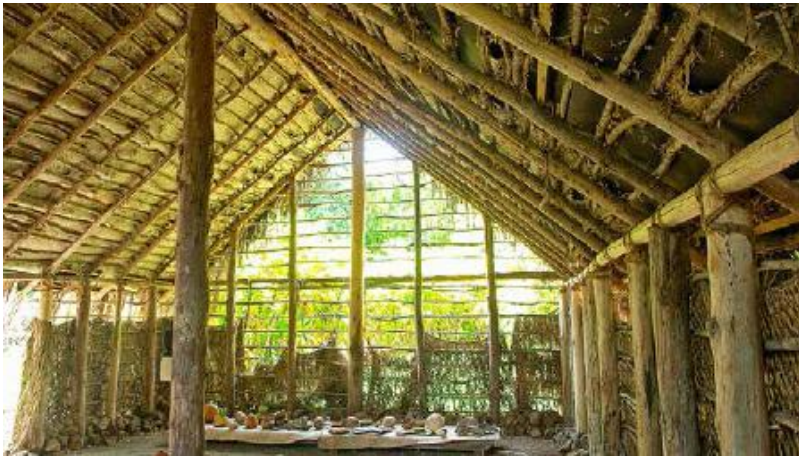
FIGURE 37.2. A traditional Hawaiian Hale house constructed of round-pole timber with lashed joints. Note woven palm front mats for the ceiling and palm thatch used for walls and roof. [Credit: Catherine Wanek]
