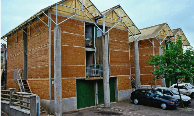
FIGURE 26.2. A contemporary solar rammed earth condo in a neighbourhood development near Lyon, France, constructed entirely from rammed earth and compressed earth blocks, called “Domain de la Terre.” These sturdy and comfortable homes are in high demand. [Credit: Catherine Wanek]
