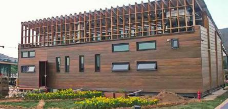
FIGURE 55.2. XAUAT's entry house for the 2013 solar decathlon included straw bale insulation, passive solar heating and a hydronic radiant cooling and heating system. [Credit: Liu Yang]
