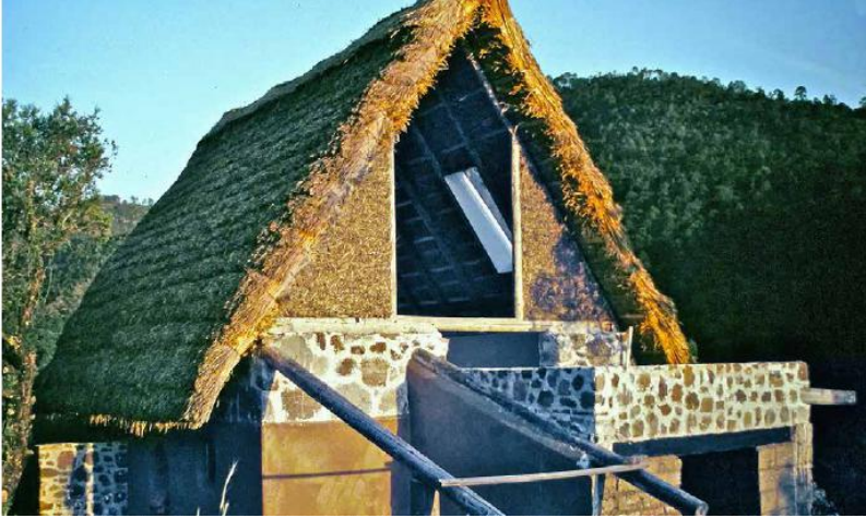
FIGURE 14.4. When Alejandra Caballero set out to renovate this adobe and stone structure in central Mexico, she chose straw-clay for the second-story walls because of its light weight and insulating properties. The thick thatched roof also provides good insulation. [Credit: Michael G. Smith]
