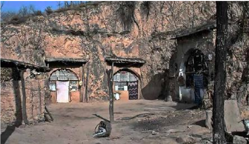
FIGURE 29.1. These traditional cave dwellings, known as Yao Dong , were carved into the silty soil of China's Loess
