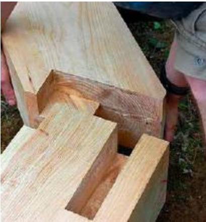
FIGURE 36.6. The foot of a principal rafter is set onto the top of its receiving post. All joints should be tested to make sure they fit prior to assembly. [Credit: Steve Chappell]
