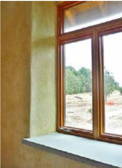
FIGURE 6.2. This detail of the Sonoma Valley homestead illustrates the thick straw bale walls and energy-efficient
