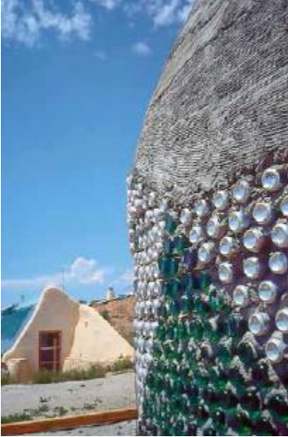
FIGURE 39.3. Aluminum cans and bottles are used to create this outbuilding for an Earthship project in Taos, New Mexico. [Credit: Joseph F. Kennedy]
