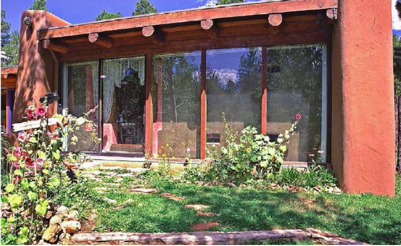
FIGURE 14.2. A south-facing trombe wall helps heat Jan and Tom Moffat’s rammed earth home in Flagstaff, Arizona, a high-altitude climate that can get very cold in the winter. However, this wall proved to be too large, and actually over heated the bedroom space inside during part of the year. The lesson? Passive solar and mass systems must be oriented and sized properly, with appropriate overhangs for the latitude and climate. This size of wall might be perfect for a greenhouse or large common space, while a smaller trombe wall would have worked better for the bedroom. [Credit: Catherine Wanek]
