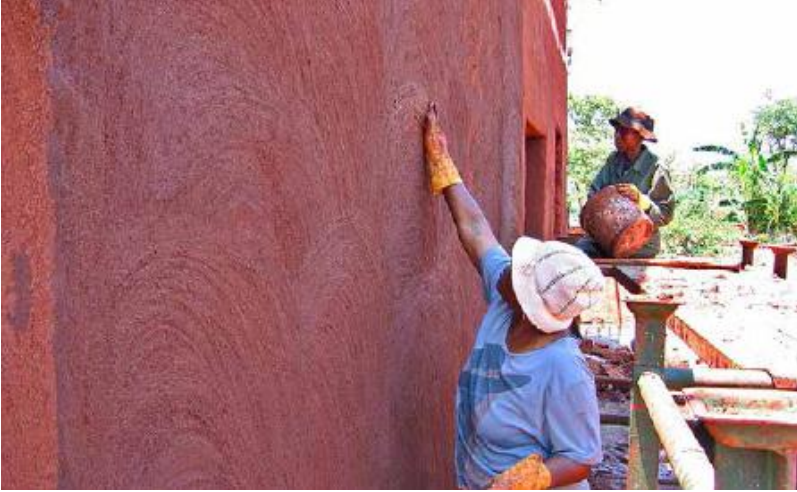
FIGURE 48.4. Applying an earth plaster to a straw bale wall in Mexico. [Credit: Joseph F. Kennedy]
