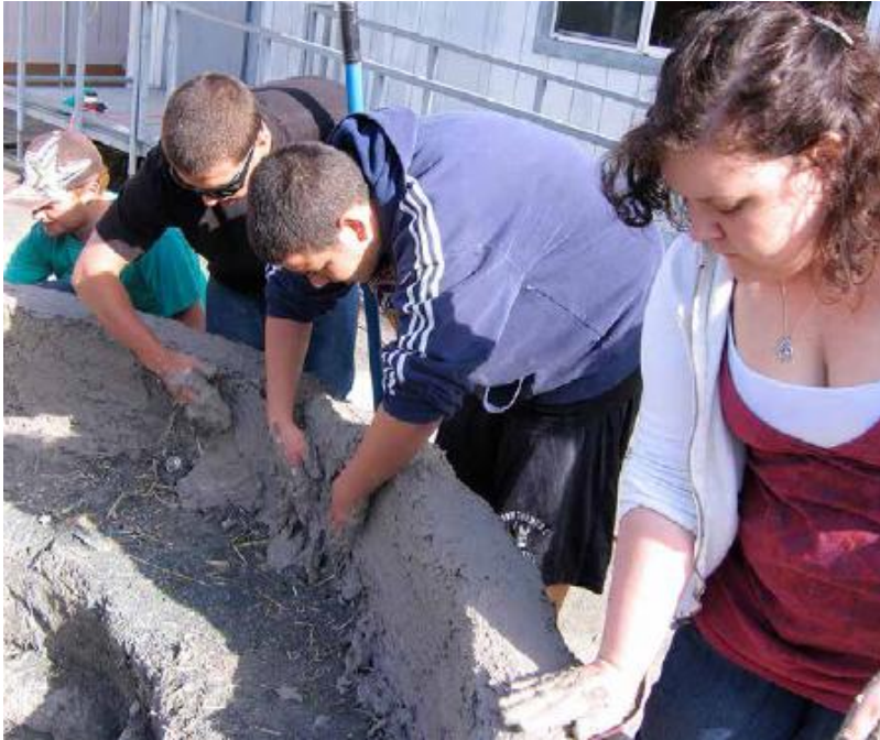
FIGURE I.5. Natural building projects like this cob bench can provide an empowering creative outlet for urban youth, while teaching technical concepts and teamwork skills. [Credit: Joseph F. Kennedy]
