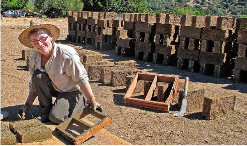
FIGURE 24.3. Making small adobe bricks using a wooden slip form. The cured but not yet dry adobe bricks are stacked to enable good ventilation and even drying. [Credit: Michael G. Smith]
