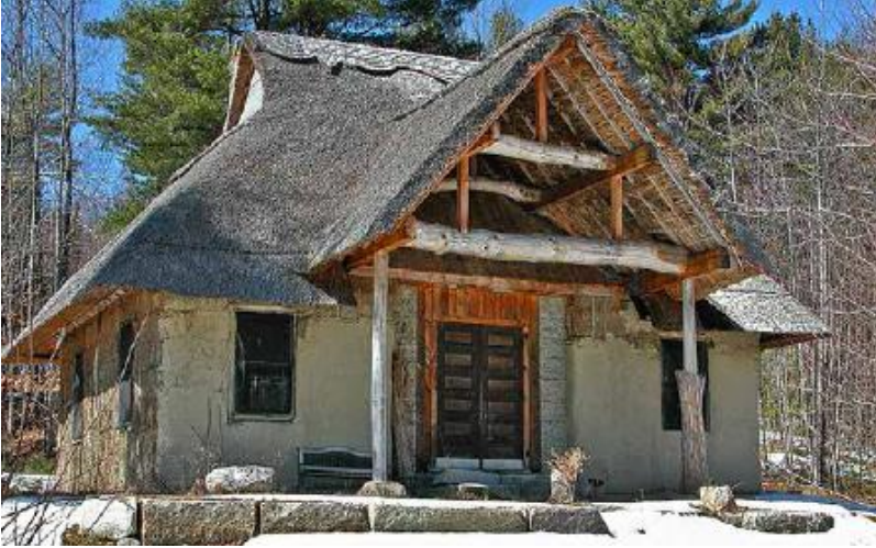
FIGURE 35.6. The library at Fox Maple follows the design of the medieval Japanese minka. This was not planned, but resulted from our decision to build the structure using only materials harvested within 50 miles of the site. It was only afterwards that I recognized its similarity to minkas, which were designed under the same constraint. [Credit: Steve Chappell]
