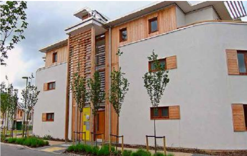
FIGURE 32.5. A hemp-lime apartment building called Tomorrow's Garden City in Letchworth, England. This was featured in two prime-time TV programs. Houses built here used Tradical Hempcrete with Baunit render. [Credit: Tom Woolley]
