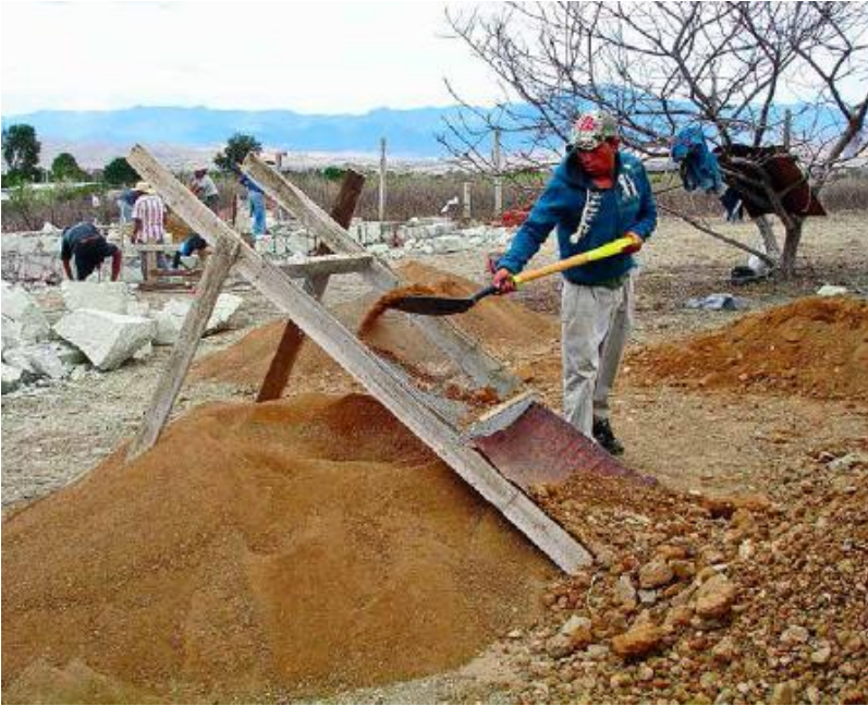
FIGURE 21.2. Sifting clay-rich soil through a fine screen to make cob. [Credit: Valentina Mendez Marquez]
