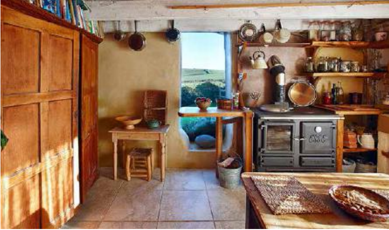
FIGURE 10.1. Katy Bryce and Adam Weismann converted a 17th-century cob granary in Cornwall, England, into a cozy, healthy home. The updated aesthetic includes bigger windows for daylighting and passive heating and a skillful combination of smooth clay plasters and rough-sawn lumber. [Credit: Ray Main]
