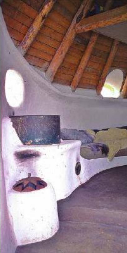
FIGURE 18.2. This rocket mass heater heats Flemming Abrahamsson’s cob studio in Denmark. The cob bench is kept warm by flue gases passing through it from the combustion unit, which can be constructed primarily from salvaged barrels and other waste materials. [Credit: Catherine Wanek]
