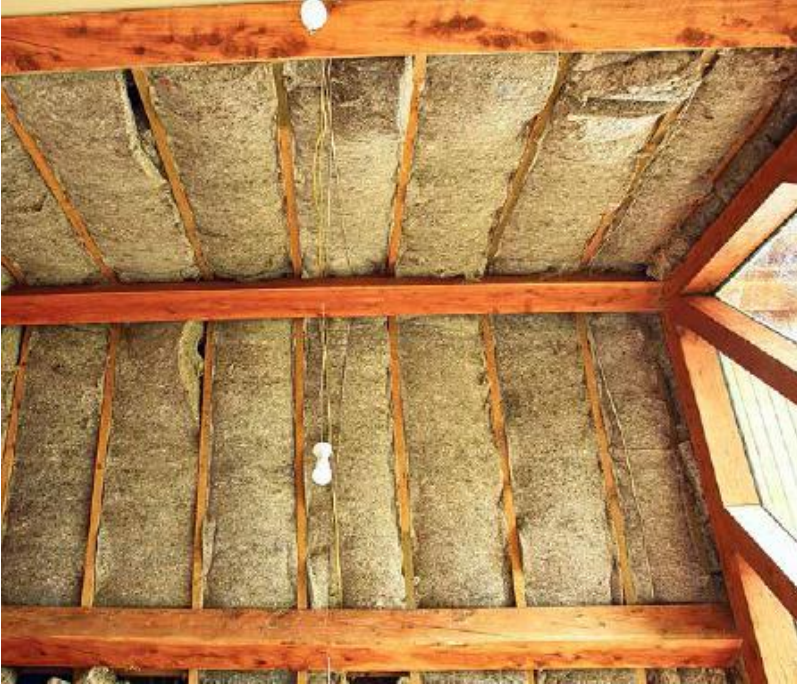
FIGURE 45.1. Wool batts insulate the ceiling of Glenn and Karen Harley’s straw bale home near Christchurch, New Zealand. [Credit: Catherine Wanek]
