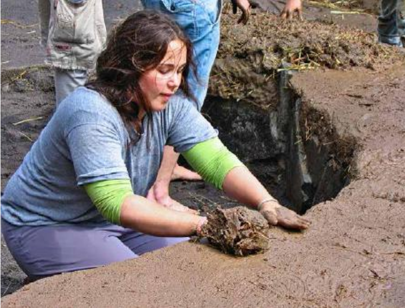
FIGURE 20.1. Creating a cob bench and kiosk at a Portland, Oregon, elementary school. [Credit: Joseph F. Kennedy]
