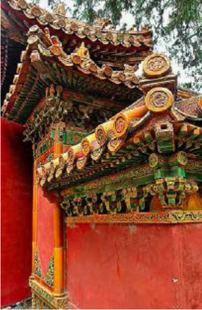
FIGURE 2.6. No less impressive are the construction techniques of the Palace Museum in Beijing, otherwise known as the Forbidden City, and the surviving Buddhist monasteries, some over 1,000 years old. [Credit: Catherine Wanek]
