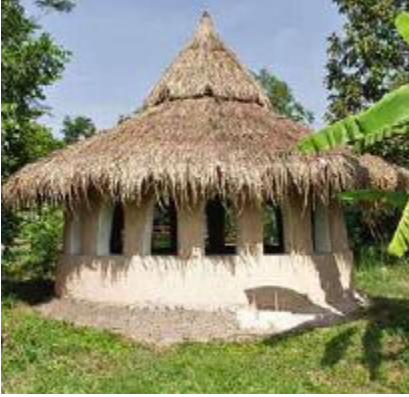
FIGURE 57.2. The first bahn din or “mud house” in Thailand was this meditation hut built at Wongsanit Ashram near Bangkok in 2001. [Credit: Janell Kapoor]
