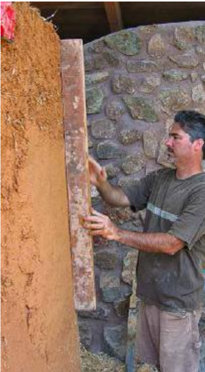
FIGURE 21.8. Using an angled plumb stick to obtain the proper degree of slope in this cob wall. [Credit: Joseph F. Kennedy]
