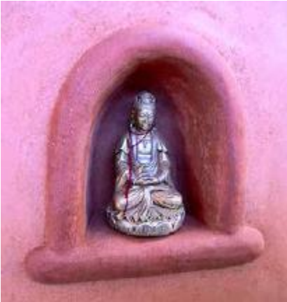
FIGURE 9.3. A small niche is lovingly carved into a cob wall to contain this sculpture. [Credit: Joseph F. Kennedy]
