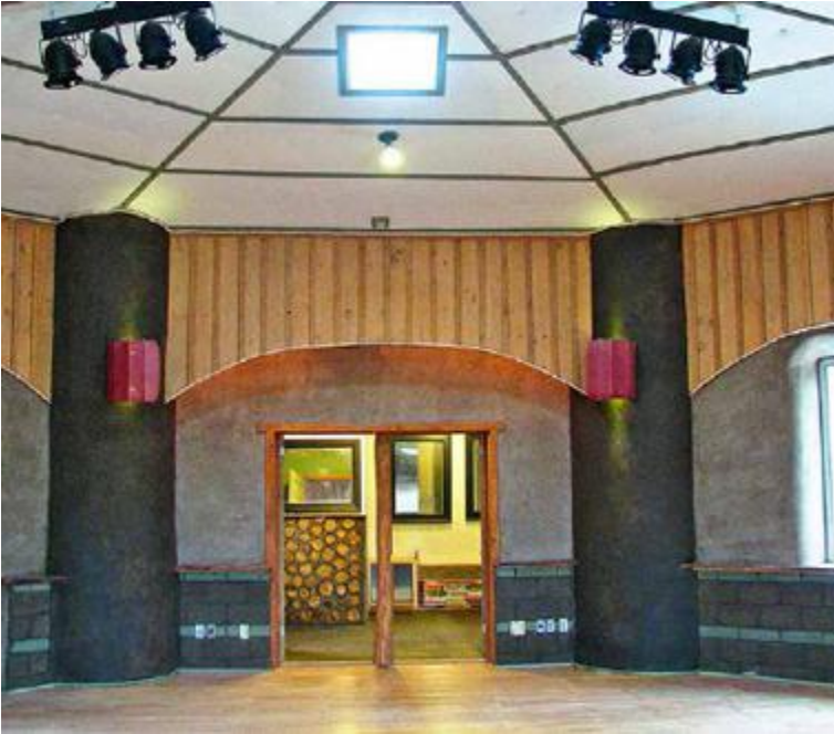
FIGURE 32.10. Inside, the round hemp bale columns are darkened with additional coats of linseed oil on the clay/hemp plaster. The ceiling in the performance space is hemp canvas to help with the acoustics. Local compressed earth blocks are used for the wainscot. The performer room, seen through the doorway, features cobwood walls and an earthen floor. [Credit: Chris Magwood]
