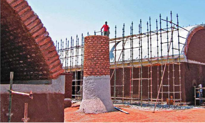
FIGURE 51.3. This vaulted HIV/AIDS hospice in South Africa was constructed of earth blocks by local builders and features innovative sustainability features for passive cooling and lighting, solar hot water production and local food production. [Credit: Joseph F. Kennedy]
