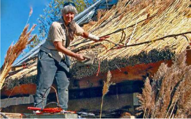
FIGURE 44.6. Deanne Bednar thatching the roof of the Kensington Kids’ Cottage, at Detroit’s oldest and biggest metropark. Reed was collected by park staff and many volunteers. [Credit: Deanne Bednar]
