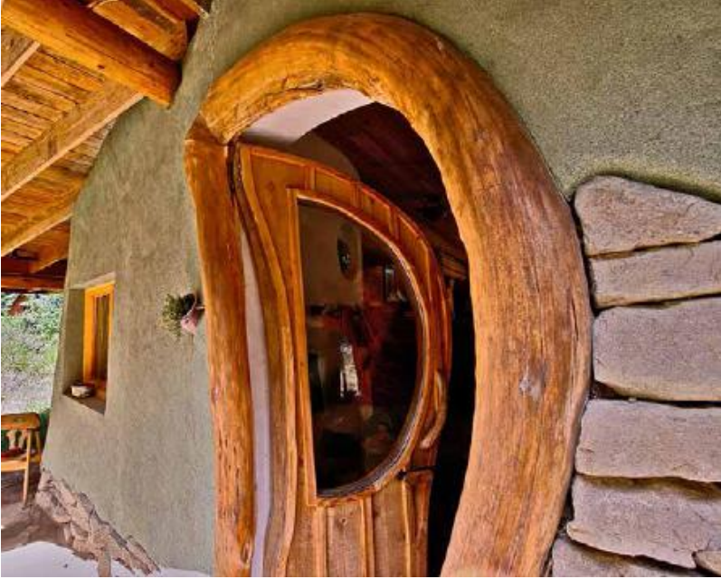
FIGURE I.6. Come on in — the door is open! This family home in British Columbia, built by Cobworks in collaboration with the homeowners, combines cob walls, local stone foundations, milled and unmilled wood and natural plasters. [Credit: Misha Rauchwerger]
