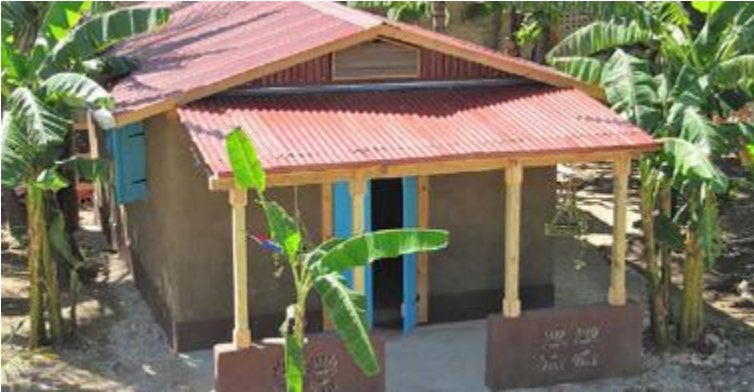
FIGURE 59.6. The Ti Kay Pay (small straw house) demonstration building, built with seismic and hurricane forces in mind, was Builders Without Borders’ answer to rebuilding after Haiti’s devastating earthquake in 2010. [Credit: Martin Hammer]
