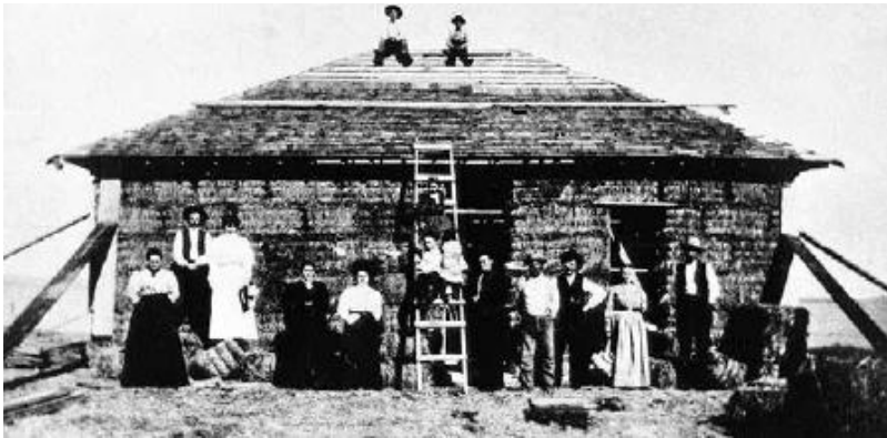
FIGURE 31.1. Pioneers who settled in the sandhills of western Nebraska found themselves in rolling hills with few trees and sandy soils. From the material at hand — bales of prairie grass — they built themselves sturdy homes. Some of these historic homes still stand today, proving the viability of plastered straw bale construction. [Credit: Courtesy Matts Myhrmann]
