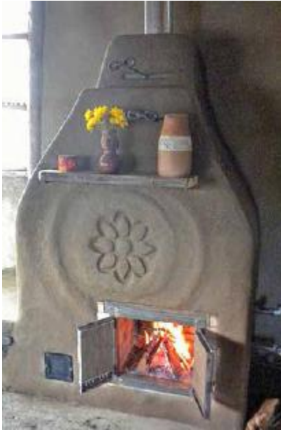
FIGURE 58.5. The author built this masonry heater with a heated bench to the left and water heating capacity. Everything for this heater was sourced within a mile from its location, except for the metal for the hardware, which was purchased but then fabricated within five miles. For more on Max and Eva’s work with earthen building and masonry heaters, see firespeaking.com . [Credit: Eva Edleson]
