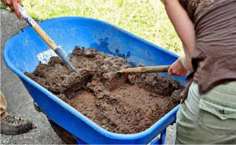
FIGURE 47.4. Mixing an earthen floor mix in a wheelbarrow with two hoes. The ideal consistency is similar to cake batter. [Credit: Mira Stebvika]
