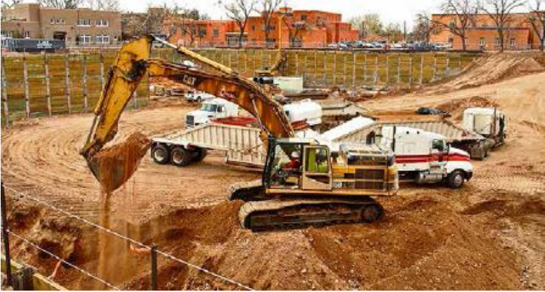
FIGURE 5.2. All construction begins with destruction. [Credit: Catherine Wanek]
