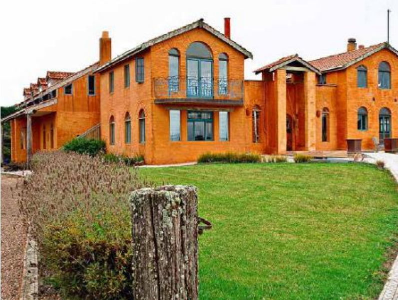
FIGURE 24.2. A single-family home made from stabilized adobe blocks in New Zealand. [Credit: Catherine Wanek]
