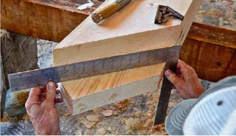
FIGURE 36.2. It is important to make sure that joinery is executed accurately if a tight and sound frame is to result. The margin of error for a strong joint is less than \frac{1}{16} of an inch. [Credit: Steve Chappell]
