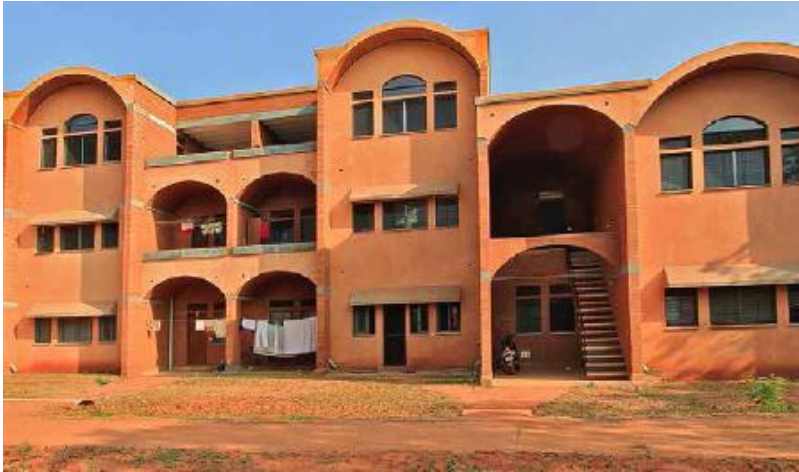
FIGURE 62.5. The Realization Community is built of compressed earth blocks, as are most buildings at Auroville. [Credit: Serge Maïni]
