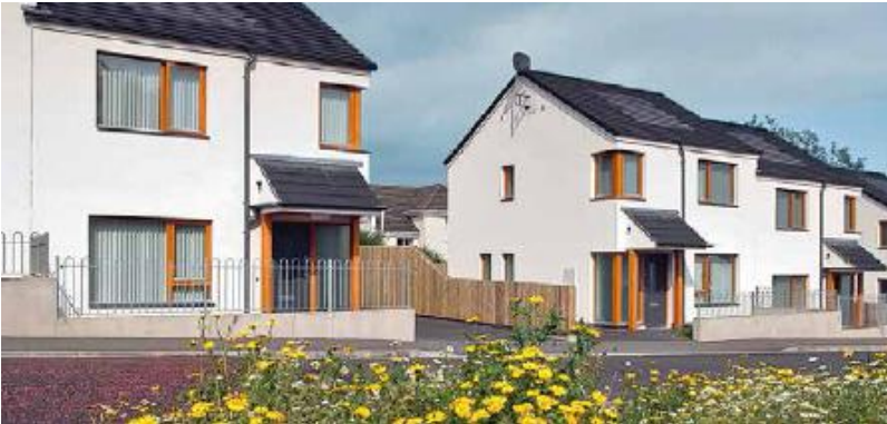
FIGURE 32.6. Drumalla House social housing in Carnlough, Northern Ireland — one of many hempcrete
