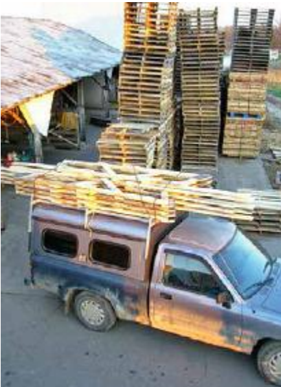
FIGURE 64.3. Pallet truss sections loaded up for transfer to Red Earth Farms. The owner of the pallet salvage operation let the author set up a jig and build the trusses at his mill. He was so impressed with the technology that he built himself an entire fishing cabin with repurposed pallet wood. [Credit: Mark Mazziotti]
