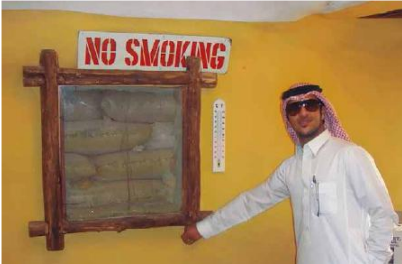
FIGURE 28.6. A visitor indicates the “truth window” in an earthbag structure in Saudi Arabia. The burlap bags used for this building are generally not advised as they more easily degrade over time, potentially impacting structural integrity. [Credit: Meshaal Abanomia]
