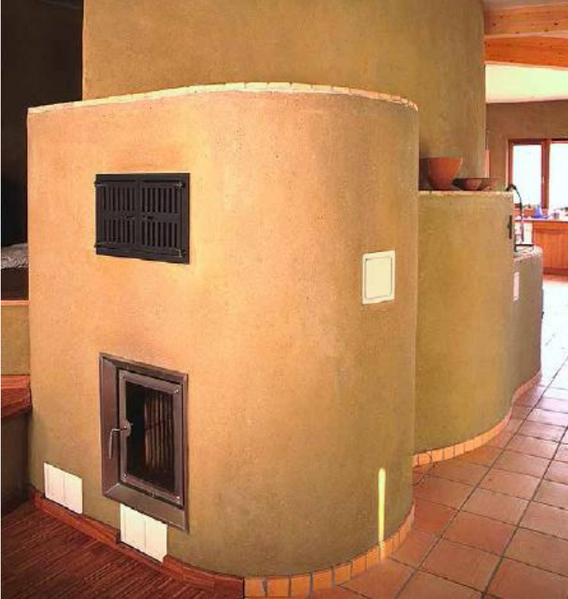
FIGURE 18.1. This sculptural masonry stove in Belgium combines a firebrick core with earthen exterior finishes. [Credit: Catherine Wanek]
