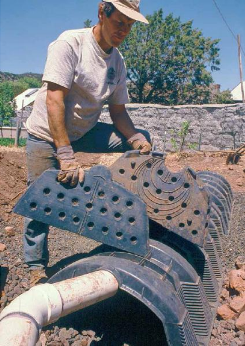
FIGURE 18.11. This plastic infiltrator is the core of a “Watson wick,” an alternative to conventional septic and
