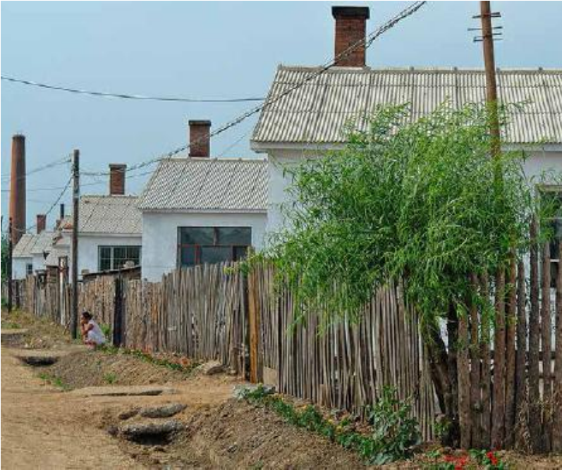
FIGURE 54.1. In northeastern China, this community of 42 modest homes was built with brick structure, with straw bales filling in the walls. Normally Chinese homes are heated with coal, which is expensive and contributes to smoke-related illness. Incorporating straw bales as insulation reduces the need for coal by two-thirds. [Credit: Catherine Wanek]
