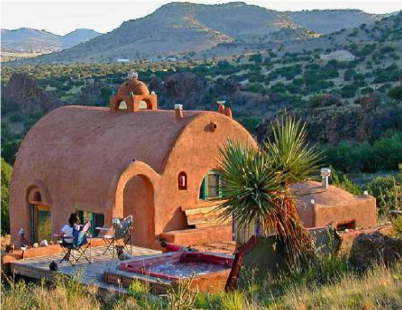
FIGURE 41.5. Domes and vaults are easy to construct from lightweight papercrete blocks. Tom Curry built this vaulted papercrete home, called Sunny Glen, in Alpine, Texas. [Credit: Tom Curry]
