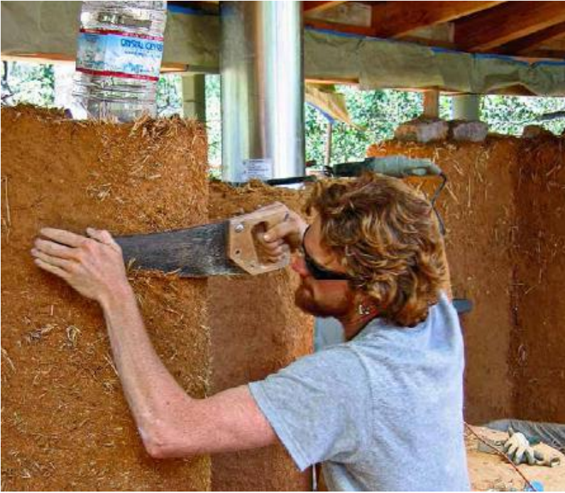
FIGURE 25.5. Cob is most easily trimmed to make surfaces plumb and even at the “leather-hard” stage, when it is firm but not yet dry. [Credit: Joseph F. Kennedy]
