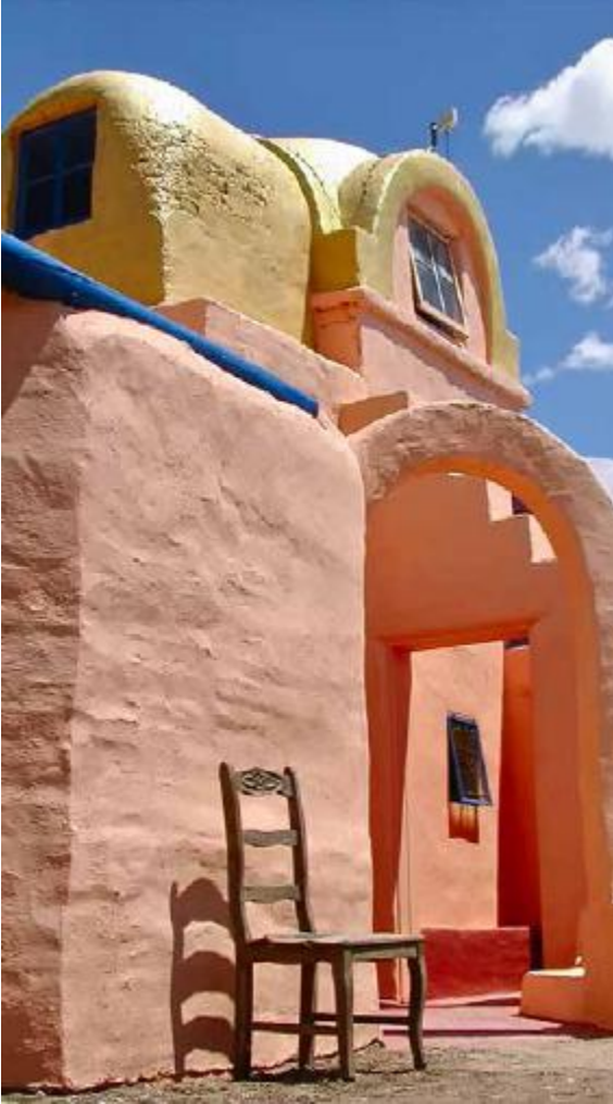
FIGURE 41.1. This papercrete dome at Eve’s Garden Bed and Breakfast was built by Clyde Curry in Marathon, Texas. [Credit: Clyde Curry]
