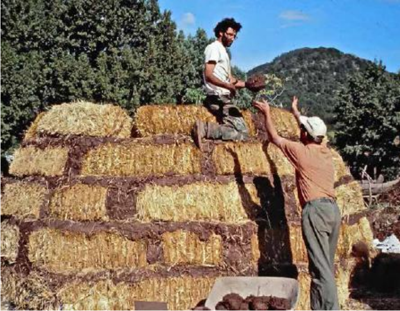
FIGURE I.3. Natural Building Colloquia have inspired a great deal of collaboration and cross-pollination between practitioners of different building techniques. When the “straw bale people” met the “cob people” at the 1995 Colloquium, this hybrid dome was the result. [Credit: Catherine Wanek]
