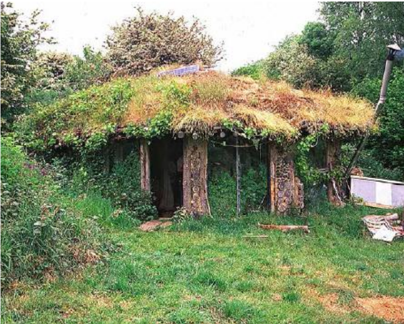
FIGURE 16.5. Jane Faith and Tony Wrench built this inexpensive, cement-free home at an ecovillage in Wales
