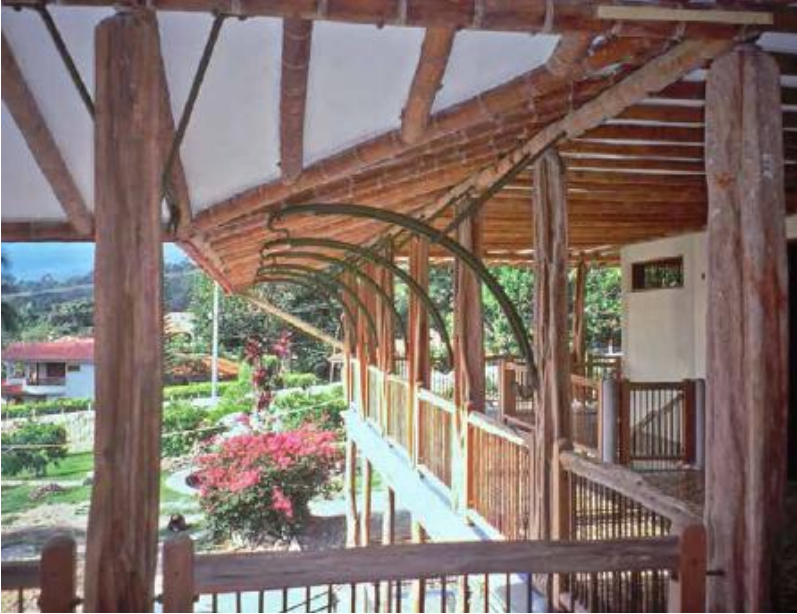
FIGURE 38.7. Note the creative use of indigenous timber, structural bamboo and wrought iron supports in this plastered bamboo dwelling. [Credit: Darrel DeBoer]
