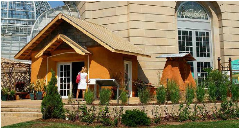
FIGURE 59.4. The Builders Without Borders Ecohouse was an exciting opportunity to create a demonstration of traditional, sustainable building methods on the national mall in Washington, DC. The BWB building team was hosted by the U.S. Botanic Garden and supported by numerous sponsors. [Credit: Catherine Wanek]
