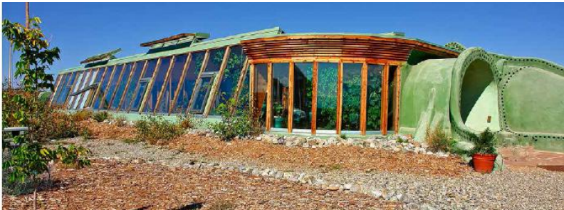
FIGURE 40.1. The angled windows of the Earthship welcome center in Taos, New Mexico, are designed to harvest the winter sun. [Credit: Catherine Wanek]
