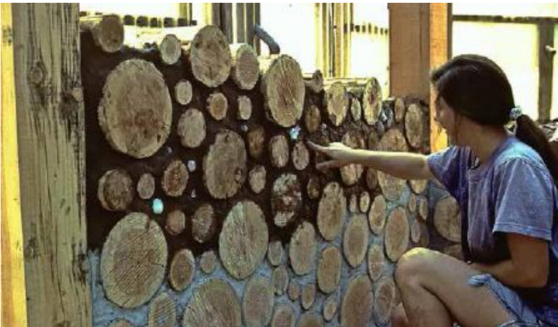
FIGURE 30.6. Cordwood walls can also be mortared with mud (a clay/sand/fiber mixture). This is more eco-friendly, and typically less expensive, than cement mortar.
