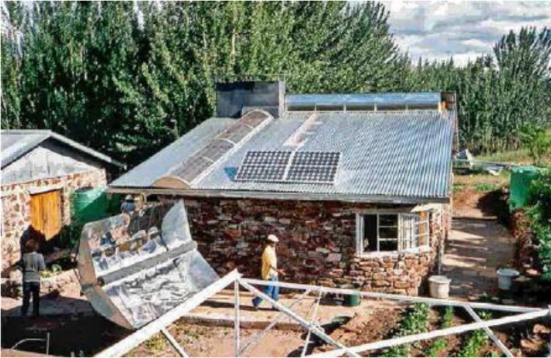
FIGURE 18.3. A kitchen at the Bethel Business and Community Development Center, a sustainability learning and demonstration center in rural Lesotho. Some of the technologies in use here include roof-integrated solar water heating, a parabolic solar cooker, photovoltaic panels for lighting, roof water harvesting and storage and vegetable production right outside the kitchen window. [Credit: Ivan Yahdnitsky]
