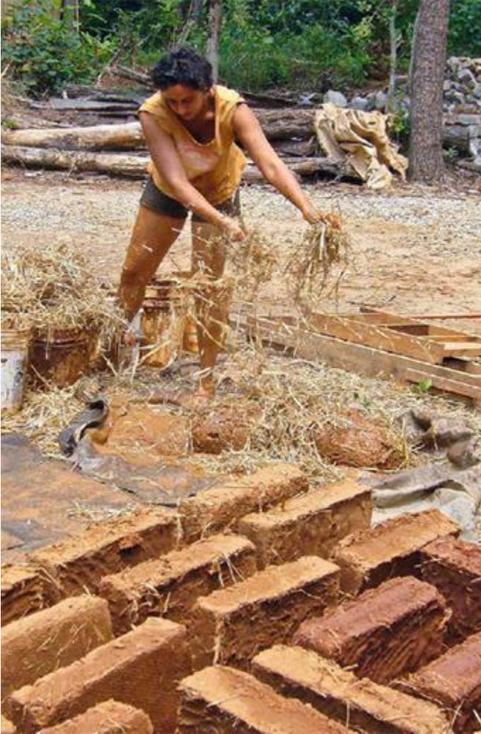
FIGURE 24.8. Janell Kapoor of Kleiwerks demonstrates adobe making at Earthaven Ecovillage in North Carolina. She combines mud and straw on a tarp, a technique borrowed from cob builders. [Credit: Mark Mazziotti]
