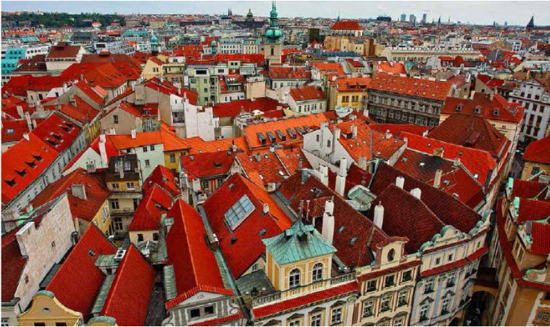
FIGURE 42.6. This roofscape in central Prague shows a combination of tile and metal roofing strategies. The valley where the houses meet can be particularly challenging to waterproof. [Credit: Catherine Wanek]
