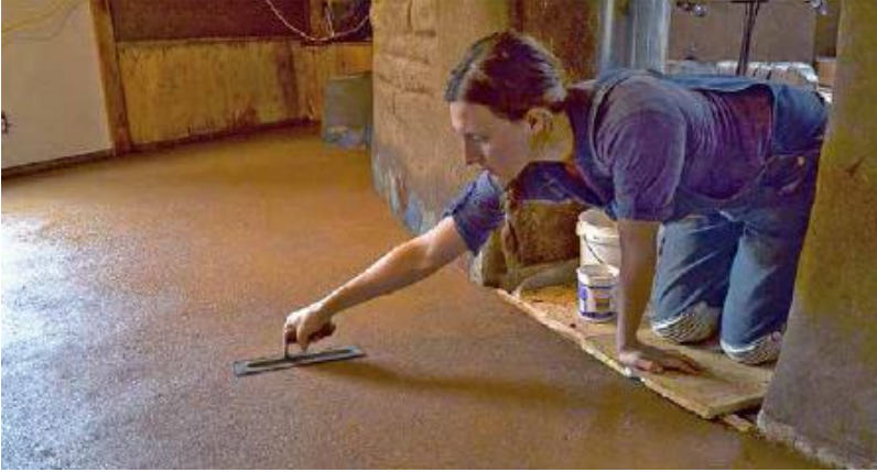
FIGURE 47.6. Burnishing an earthen floor at the leather-hard stage polishes the floor and removes trowel marks. [Credit: James Thomson]
