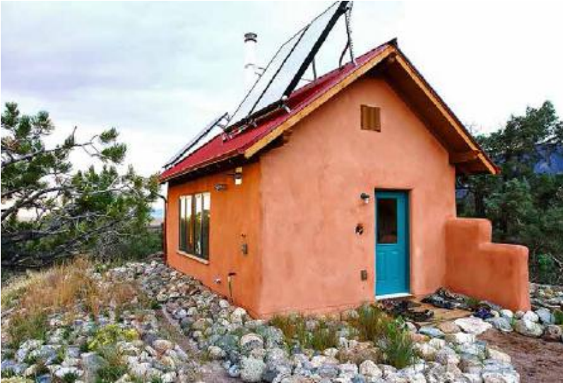
FIGURE 17.1. Keeping your house as small as possible is the best way to reduce its environmental impact. This tiny self-sufficient straw bale cottage was built for a Buddhist teacher in Crestone, Colorado. [Credit: Catherine Wanek]
