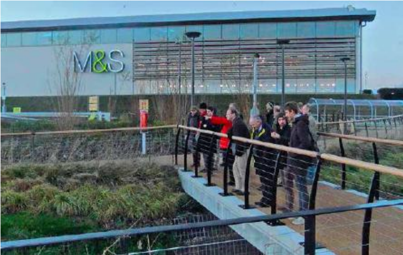
FIGURE 32.7. Cheshire Oaks Superstore with hemp-lime prefabricated walls, perhaps the largest store ever built in the UK. Marks & Spencer's make great claims as to its progress towards a carbon-neutral policy for its buildings. [Credit: Tom Woolley]
