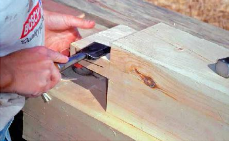
FIGURE 36.3. Paring a tenon with a framing chisel. Chisels must be kept very sharp in order to cut quickly and cleanly. [Credit: Michael G. Smith]
