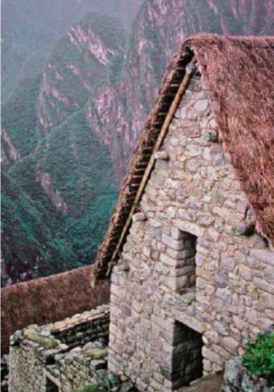
FIGURE 1.1. Everywhere on Earth, vernacular building traditions evolved that used local resources to their best advantage to meet local climatic and cultural conditions. These reconstructed Inca homes at Machu Picchu borrowed both their materials and their forms from the immediate environment. [Credit: Michael G. Smith]
