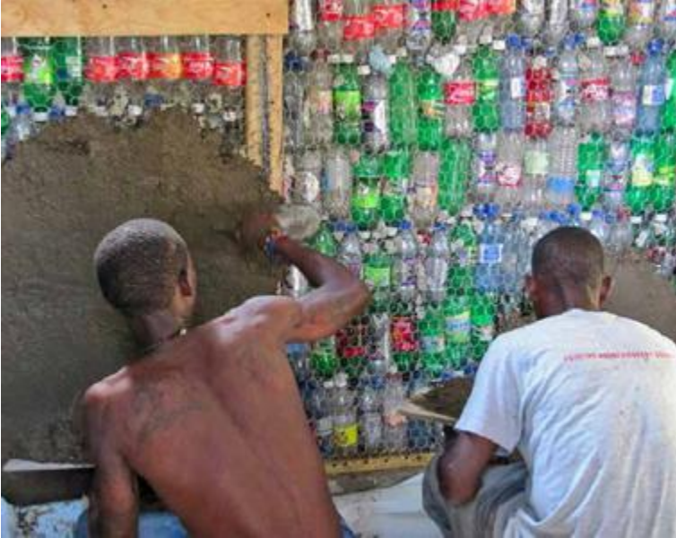
FIGURE 59.7. The Senp Kay (simple house) is a panelized system, using a simple wooden frame, filled with empty plastic soda bottles, covered with metal mesh, then plastered with clay, lime or cement plaster. [Credit: Andy Mueller]
