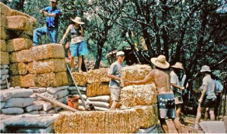
FIGURE 22.4. Bags filled with compacted soil or gravel can make a quick and versatile foundation system, especially well-suited to straw bale and cob walls. The polypropylene bag material degrades rapidly in the sun, so the bags must be protected with plaster. Here, earthbags double as both retaining wall and a foundation for straw bale walls. [Credit: Catherine Wanek]
