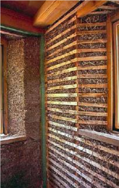
FIGURE 33.1. Two ways to make a straw-clay wall. The wall on the left was made of straw coated with clay slip and tamped into a form temporarily attached to the wall framing. To maximize insulation, the mix for the wall on the right was kept very light, with a minimum of clay slip added to the straw. This mixture was packed by hand into the wall cavity and is contained by wooden lath, which will stay permanently in place. Both walls will later
