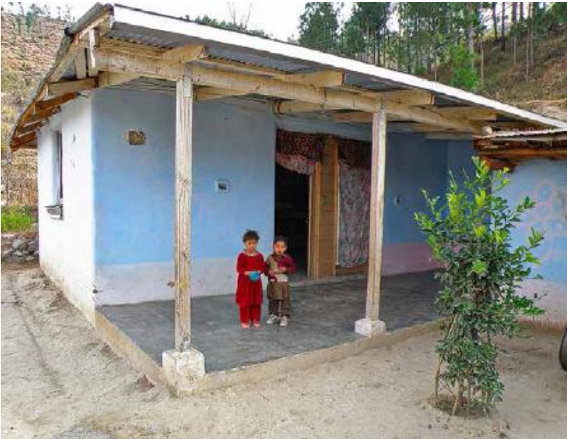
FIGURE 56.1. Finished with clay and lime plaster, the PAKSBAB straw bale homes are sturdy and comfortable, and are built for about half the cost of a conventional Pakistani home. [Credit: PAKSBAB]
