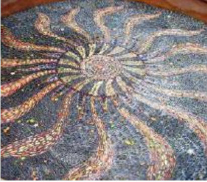
FIGURE 8.3. The revival of a Roman technique of creating finely cobbled paved surfaces by setting flat rounded stones into a dry mortar bed. Built by Bruce Hauschildt. [Credit: Joseph F. Kennedy]
