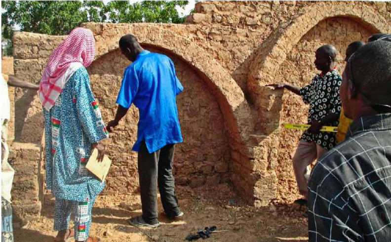
FIGURE 53.2. Starting vaults on a training structure. [Credit: John Norton]
