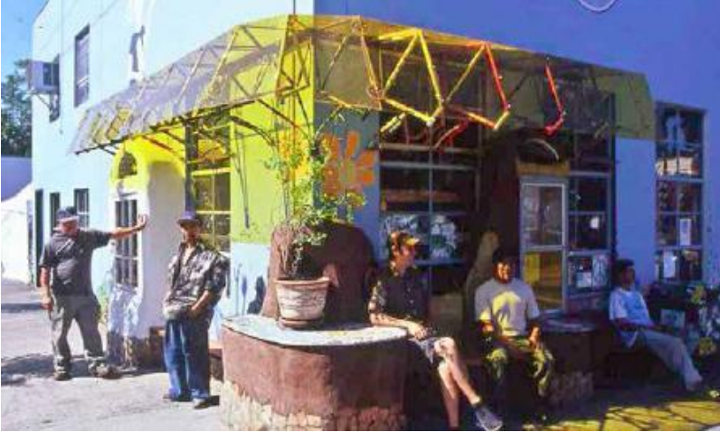
FIGURE 15.4. This bike shop has been creatively remodeled with cob and recycled bicycle parts to create shelter for the day laborers who congregate at this spot. [Credit: Mark Lakeman]
