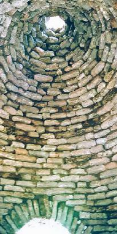
FIGURE 42.3. A domed building built of corbelled earthen bricks in Turkey. [Credit: Catherine Wanek]
