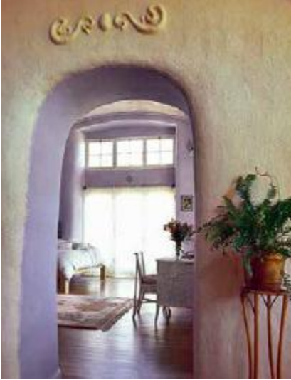
FIGURE 31.8. While functioning to manage moisture and clean the air, interior clay plasters like these in Linda Drew’s straw bale home also allow unlimited variety and creativity. [Credit: Catherine Wanek]
