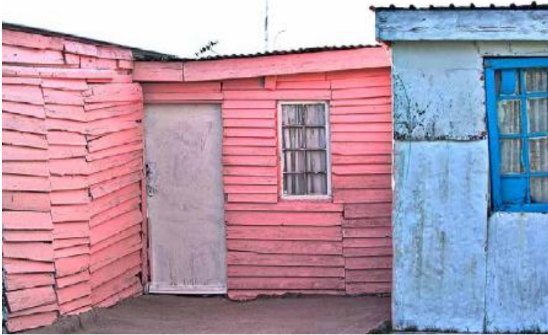
FIGURE 39.1. Resourceful builders in informal settlements (such as here in the Cape Flats in South Africa) are adept at using scrap wood and other discarded materials to make dwellings. [Credit: Joseph F. Kennedy]
