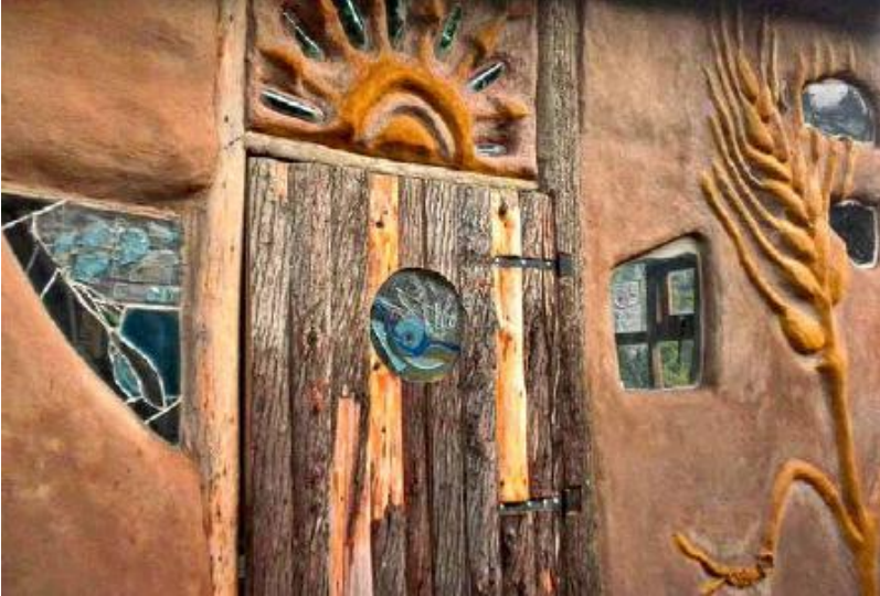
FIGURE 58.4. These earthen bas-reliefs and clay paints surround other artistic glass and carpentry work in a wire mesh wattle-and-daub wall. The clay finish work was applied during a workshop led by Eva Edleson at the community building of the Rio Azul community. [Credit: Eva Edleson]
