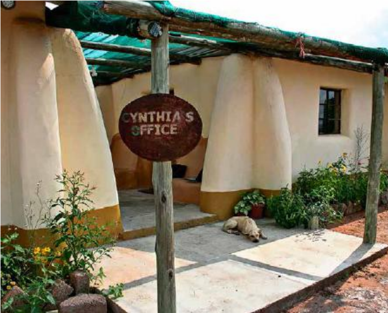
FIGURE 28.4. Completed earthbag building with cement plaster, Dennilton, South Africa. [Credit: Joseph F. Kennedy]
