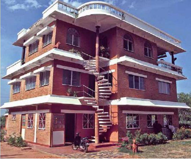
FIGURE 27.5. A three-story building constructed at Auroville of CEBs and ferrocement. [Credit: Serge Maini]
