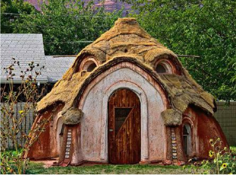
FIGURE 28.7. A sod-covered earthbag dome by Doni Kiffmeyer and Kaki Hunter, Moab, Utah. [Credit: Catherine Wanek]
