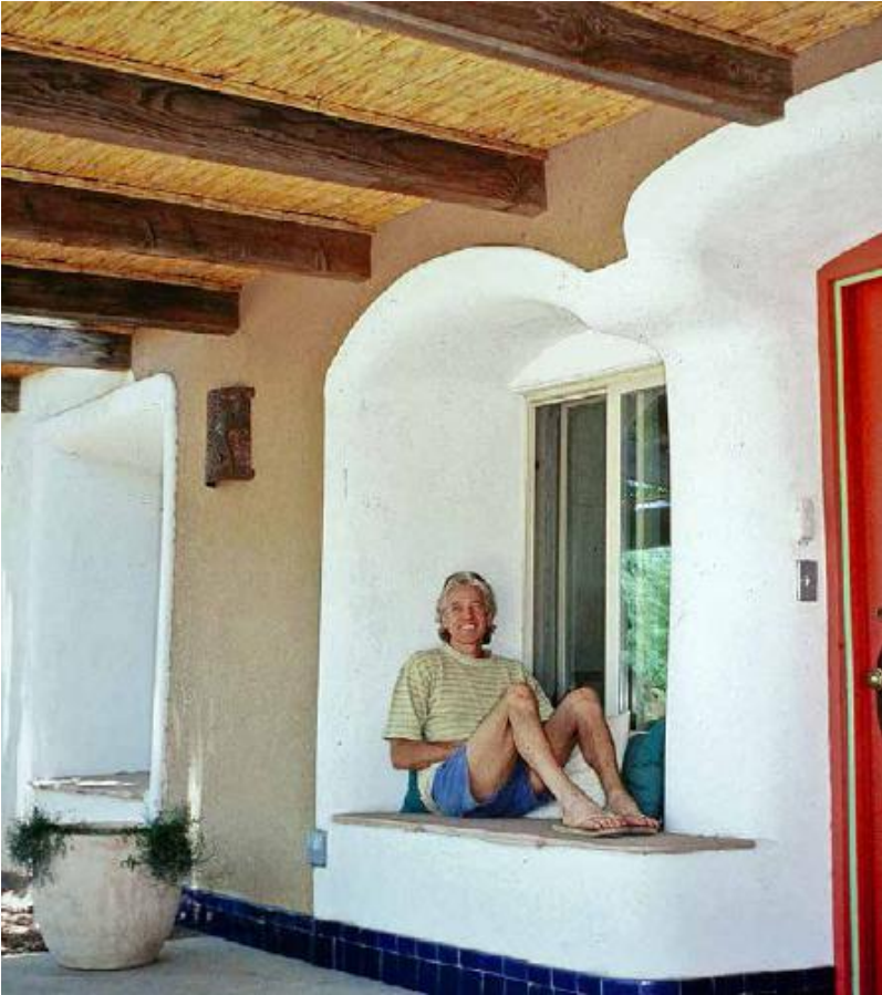
FIGURE 15.3. Plastered straw bales were used by Matts Myrman and Judy Knox to make their concrete block home more comfortable in the exceptional temperature extremes of Tucson, Arizona. The shading veranda was added to create additional outdoor space and to protect the new straw bale wall. [Credit: Janine Björnson]
