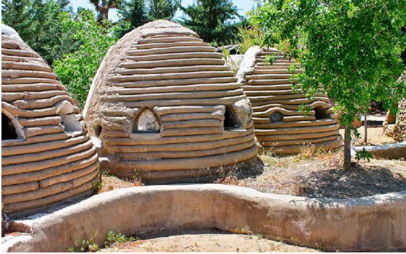
FIGURE 52.3. These student-built earthbag shelters at CalEarth demonstrate a quick and inexpensive solution to housing needs due to natural disaster or human conflict. [Credit: Joseph F. Kennedy]
