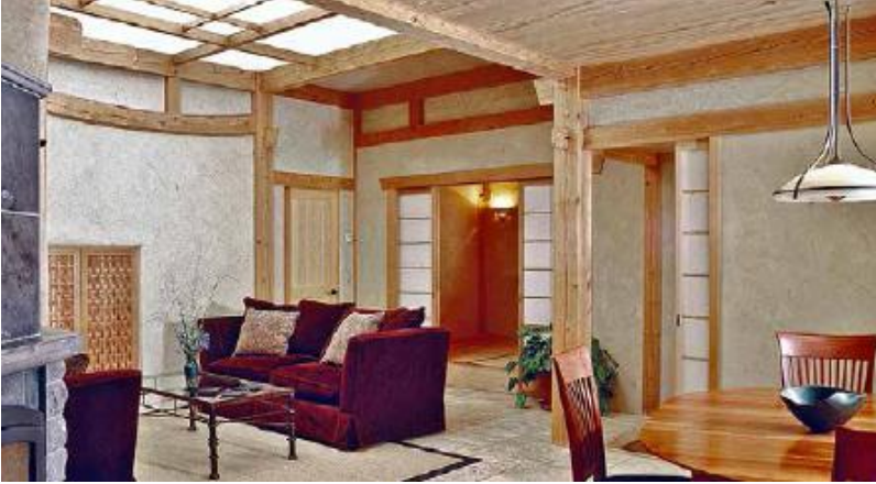
FIGURE 10.3. Timber frame elements and varying ceiling treatments create place within the open space of this compact EcoNest home. The walls are straw-clay with natural earthen plaster. [Credit: Laurie Dickson]
