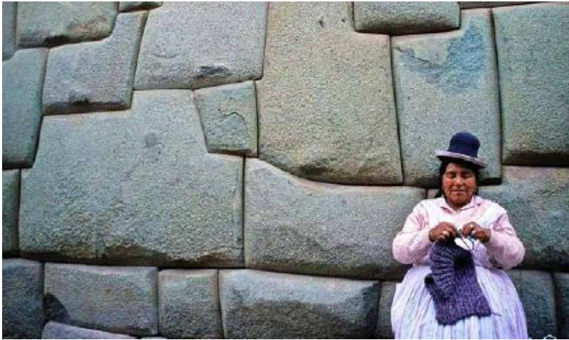
FIGURE 23.1. The Inca civilization may have seen the most skilled stonemasons of all time. The stones in this wall in Cuzco, Peru, fit together so tightly that one cannot insert a piece of paper between them, yet some of them weigh many tons. Very heavy stones with a lot of surface contact produce enough frictional resistance to withstand earthquakes. [Credit: Michael G. Smith]
