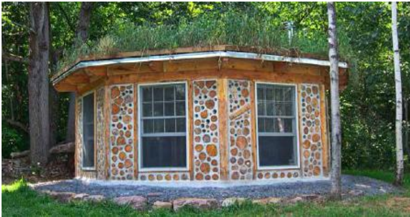
FIGURE 30.4. This octangular structural framework is infilled with cordwood and mortar. This sturdy structure also supports a living roof, which in the winter will sport an insulating cap of snow. [Credit: Rob Roy]
