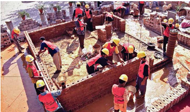
FIGURE 27.3. CEB house under construction in the Philippines. [Credit: CRAterre]
