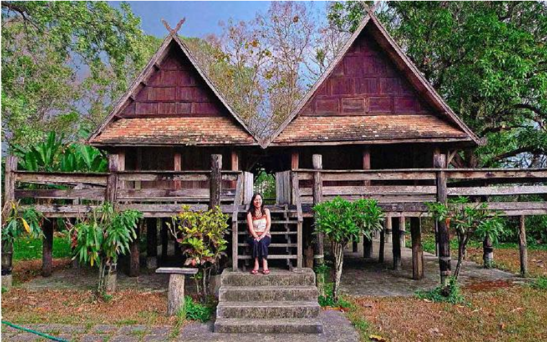
FIGURE 2.7. This vernacular home in coastal Thailand is designed and constructed to stay high, dry and comfortable even with monsoon rains and flooding waters. [Credit: Kyle Holzheur]
