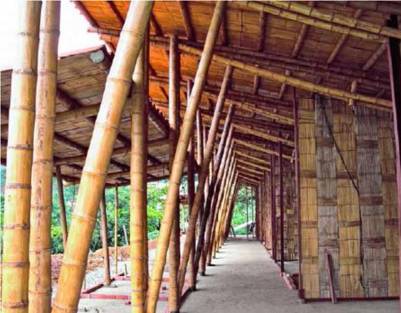
FIGURE 38.6. Curved bamboo poles used as bracing. [Credit: Darrel DeBoer]
