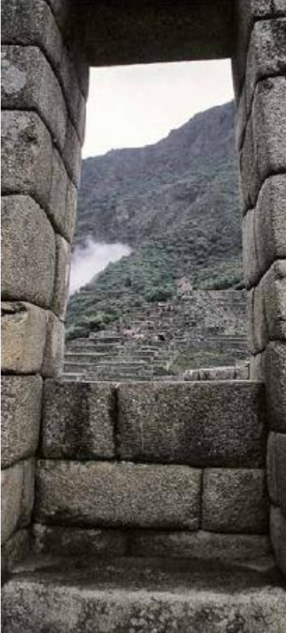
FIGURE 21.1. Using techniques we still do not entirely understand, the Inca civilization built walls and buildings using immense stones, so carefully fitted that one cannot slip a thin knife between them anywhere. [Credit: Michael G. Smith]
