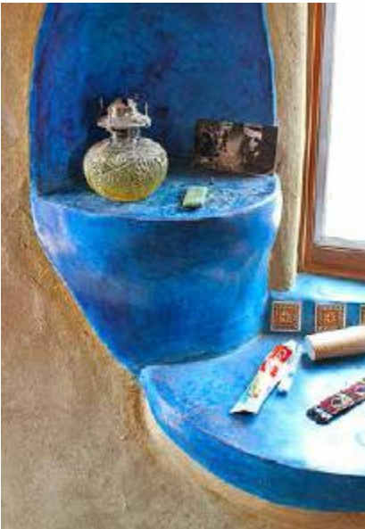
FIGURE 50.6. The Moroccan tadelakt natural finishing technique. Tadelakt is a polished and compressed lime-based finish that incorporates soap to create a glossy, water-repellant surface that can be used for bathrooms and other wet areas. [Credit: Joseph F. Kennedy]
