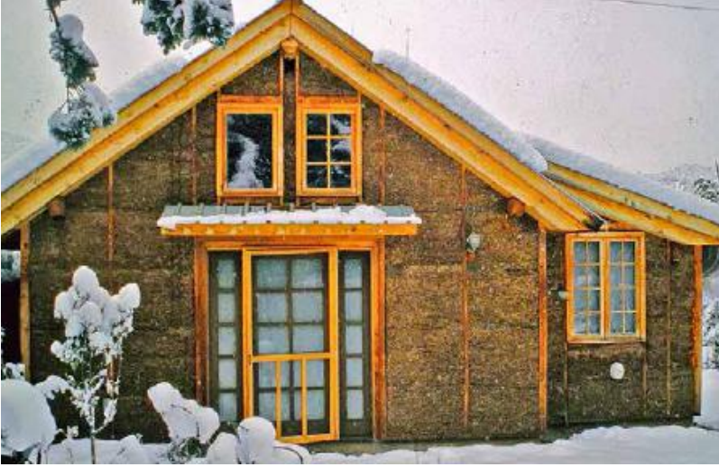
FIGURE 33.5. Straw light-clay provides good insulation, making it appropriate even in cold climates. This small house built by EcoNest Co. awaits its exterior plaster. [Credit: Michael G. Smith]
