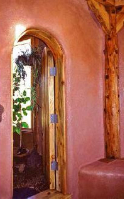
FIGURE 48.6. This adobe meditation room in Taos, New Mexico, features a micaceous clay plaster by Carole Crews. [Credit: Catherine Wanek]
