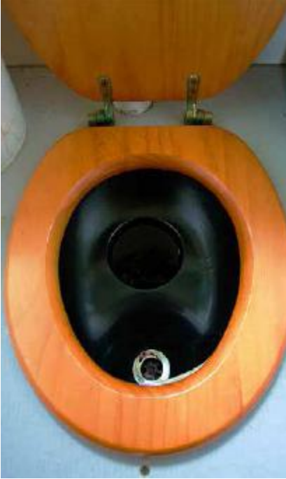
FIGURE 18.9. This composting toilet separates urine from feces so that the former can be diluted and used immediately as fertilizer while the latter is composted. Removing urine from the composting process helps to keep the temperature higher and reduces smells. [Credit: Catherine Wanek]
