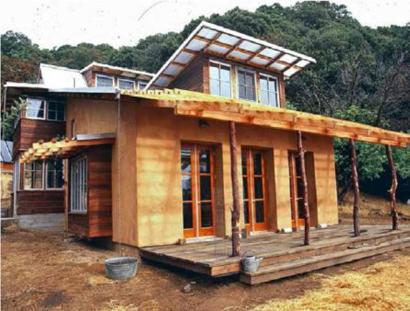
FIGURE 12.2. The clerestory windows of this off-the-grid straw bale home in Northern California are designed to maximize the entry of winter sun, while shade structures over windows facing south and west will help prevent overheating (Architects David Arkin and Anni Tilt; builder Tim Owen Kennedy, Vital Systems Natural Building & Design). [Credit: Catherine Wanek]
