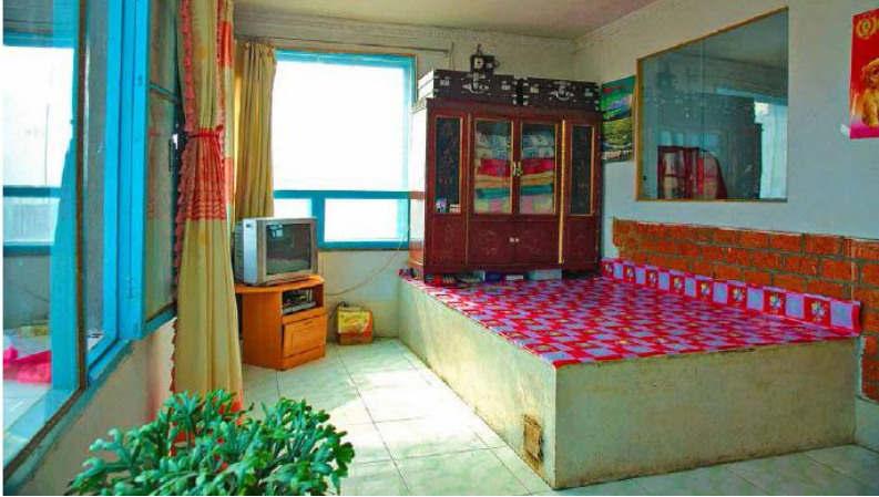
FIGURE 54.2. This typical Chinese living room features a kang , or raised sleeping platform, which is heated by the circuitous flue from the kitchen coal-burning cooking stove on the other side of the fired-brick wall. [Credit: Catherine Wanek]
