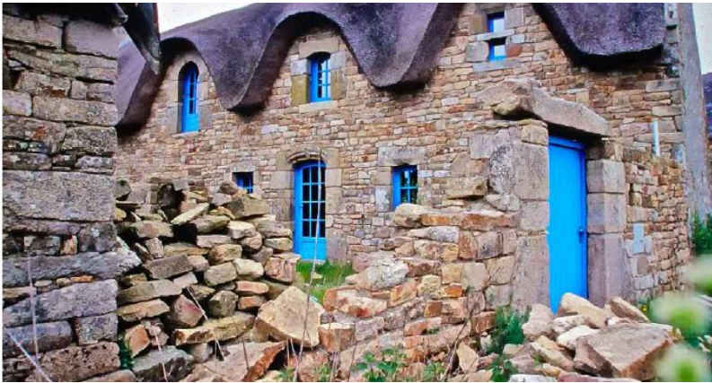
FIGURE 23.5. A historic chateau in France, being reconstructed to repair damage done by bombing during World War II. Some of the carved cornerstones and lintels bear dates from Roman times, and may have been reused in multiple buildings. [Credit: Catherine Wanek]
