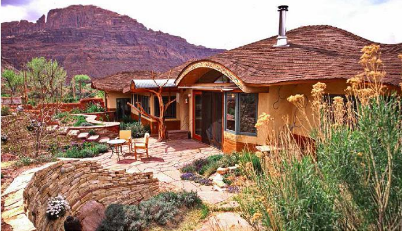
FIGURE 16.1. When designing her own home near Moab, Utah, architect Susie Harrington looked to the site for inspiration. By choosing local materials and a form that reflects the surrounding landscape, she ensured that the building would look and feel like a natural outgrowth of the site. The walls of this passive solar home are straw bale and the undulating roof is covered with recycled plastic “eco-shakes.” [Credit: Catherine Wanek]
