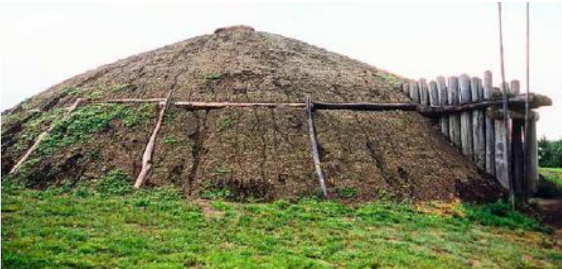
FIGURE 2.1. The Numatciki (referred as the Mander Indians) built their villages along the fertile floodplain of the Missouri River, in what is now North and South Dakota. The women of the tribes built sturdy pole
