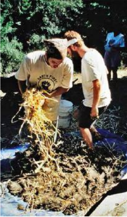
FIGURE 25.4. When mixing cob on a tarp, clay, sand and water are first combined and mixed to a doughlike consistency before straw is added. [Credit Michael G. Smith]
