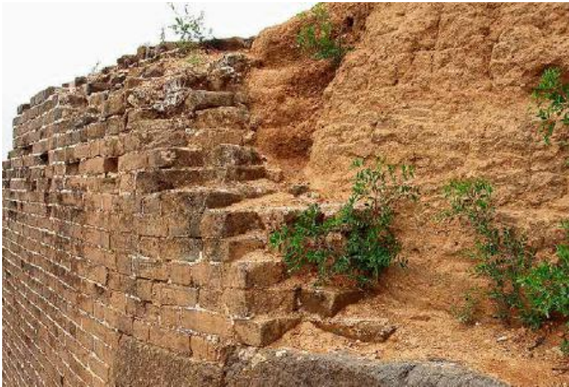
FIGURE 26.1. The majority of the 3,000-year-old, over 4,000-mile-long “Great Wall of China” was constructed of earth, hand-tamped by hundreds of thousands of workers. In later centuries, the rammed earth walls were faced with fired brick, for greater longevity. [Credit: Catherine Wanek]
