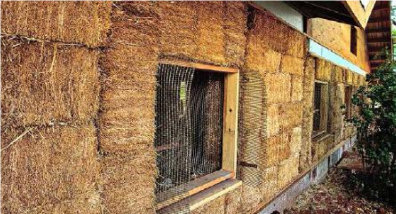
FIGURE 31.3. Plastered straw bales are strong enough to support the weight of a typical roof, along with the loads of wind and snow. In this load-bearing bale wall, the bale orientation varies, yet the bales, compressed by the bond beam, still support the roof loads. With a plaster finish, the bales will perform much like a stressed-skin wall system. [Credit: Catherine Wanek]
