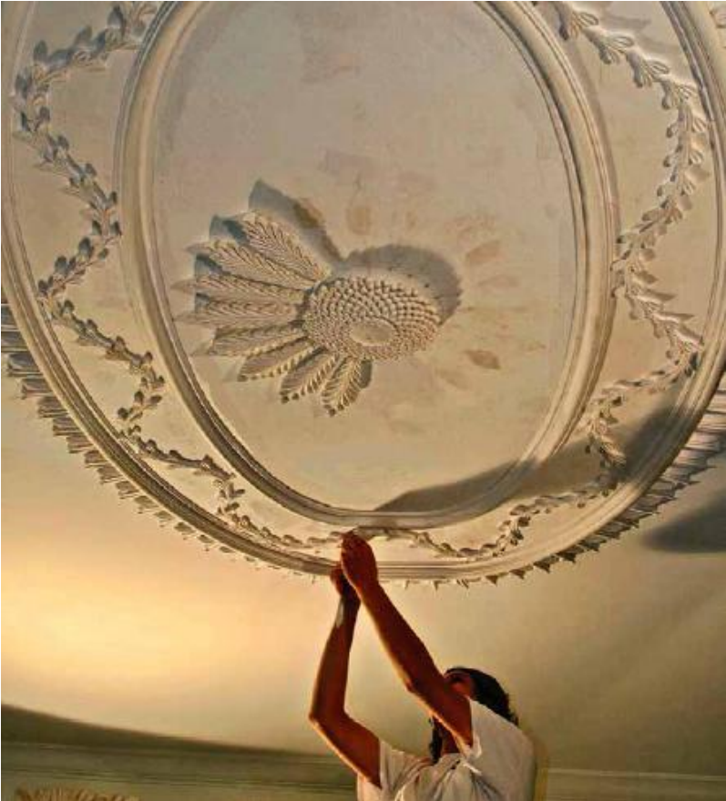
FIGURE 8.4. Hand-applying ornamental gypsum plaster details. [Credit: American College of the Building Arts]
