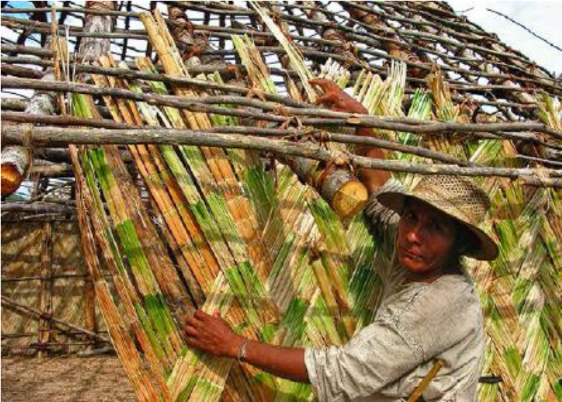
FIGURE 38.1. Using woven split bamboo as a wall covering for an indigenous dwelling in Colombia. [Credit: Shannyn Sollitt]
