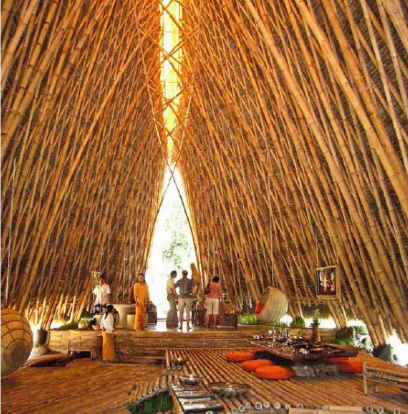
FIGURE 38.3. Jöerg Stamm’s design for this jewelry showroom in Bali gets added strength by triangulating the rafters across each other. [Credit: Darrel DeBoer]
