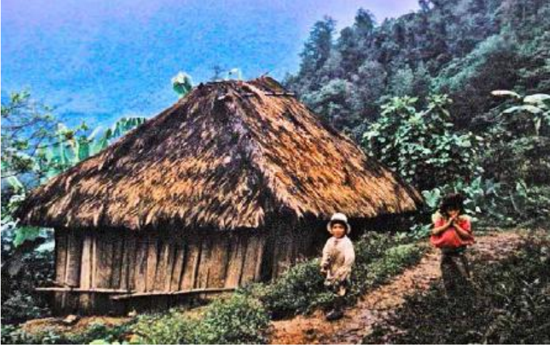
FIGURE 4.1. Throughout history, people with few economic resources have been able to build themselves adequate shelters, often both elegant and functional. This simple dwelling in highland Guatemala is made entirely from materials gathered from the forest nearby: a frame of saplings lashed together with vines, covered with split-palm trunk siding and palm frond thatch. People's capacity to house themselves according to these ancient traditions is rapidly being eroded by multiple forces, including the destruction of local ecosystems, loss of secure land tenure and economic and social forces that impel young people to seek work in the market economy, often leaving rural areas for cities. [Credit: Michael G. Smith]
