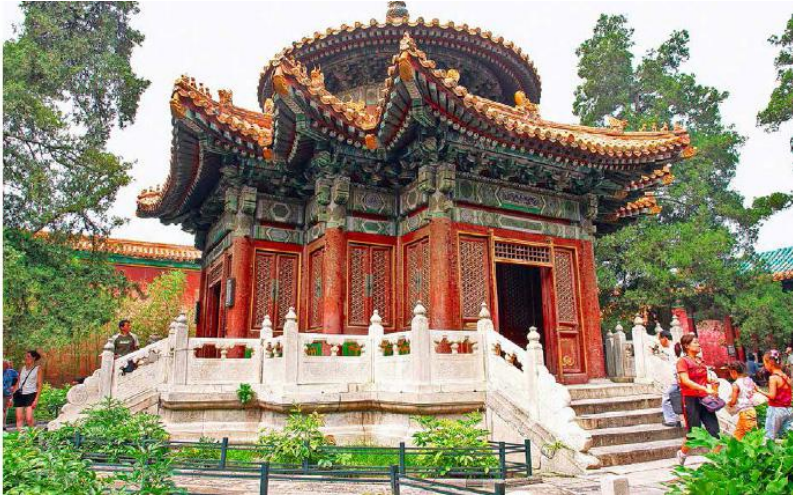
FIGURE 42.2. Roofs can be the dominant aesthetic feature of a building, as evidenced by this elaborate sculptural roof on a temple at the Palace Museum in Beijing, China. [Credit: Catherine Wanek]
