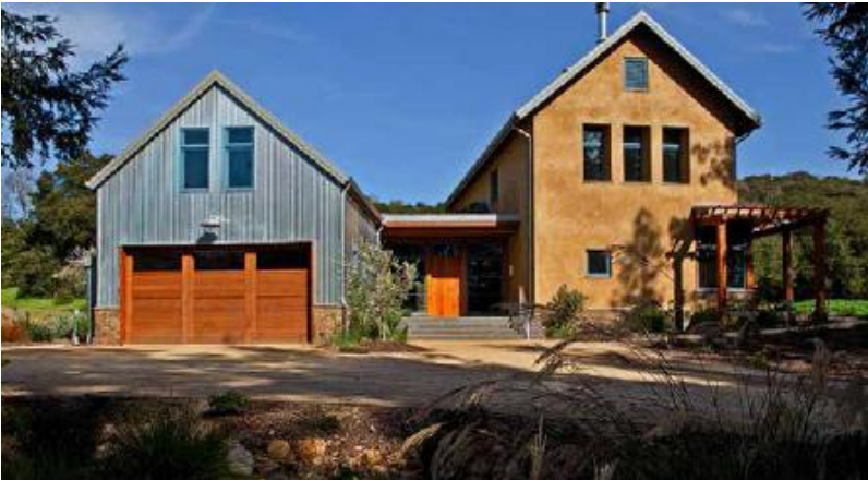
FIGURE 6.1. This Sonoma Valley homestead by Daniel Smith & Associates Architecture features straw bale walls supplemented with solar collectors, mass storage and a variety of energy- and water-efficient measures that are integral to the design, including a living roof, greywater and rainwater harvesting. This house achieved LEED for Homes Platinum certification. [Credit: Russell Abraham]
