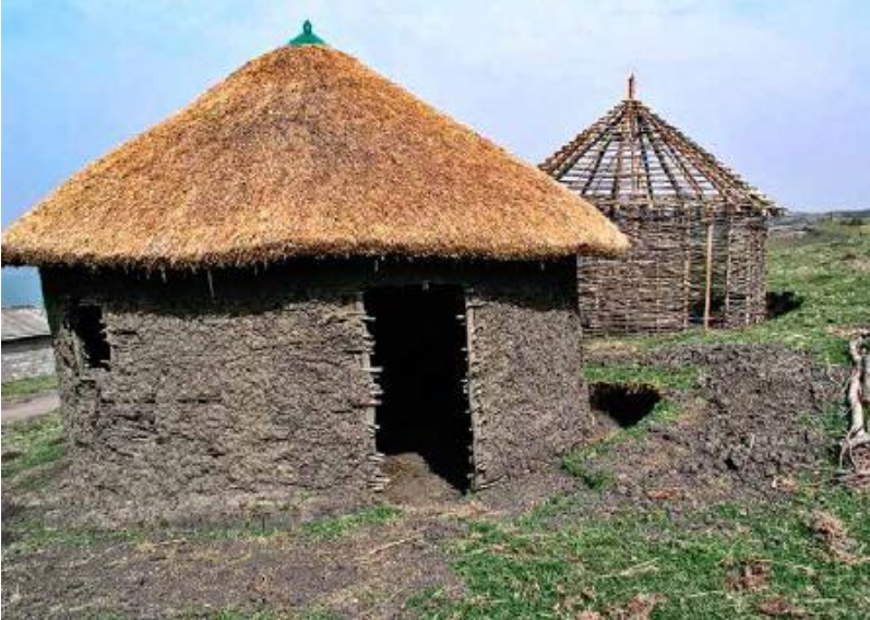
FIGURE 34.5. Thatched wattle-and-daub “rondavels” under construction in South Africa. [Credit: Mark Mazziotti]
