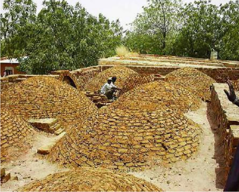
FIGURE 53.1. A roofscape of earthen domes and vaults in the Sahel. [Credit: John Norton]
