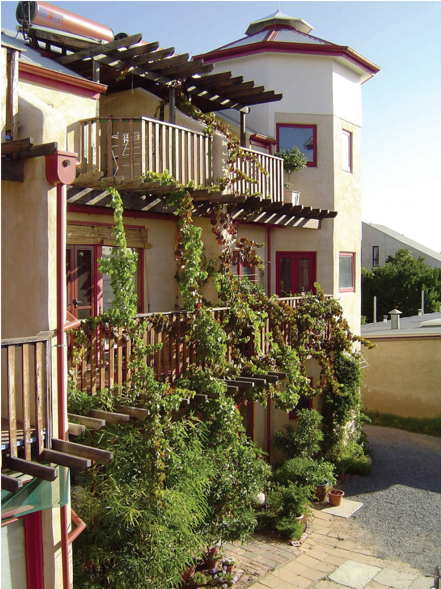
Plate 42: Christie Walk, Adelaide, South Australia Seasonal shade for solar houses from vegetation and balconies
