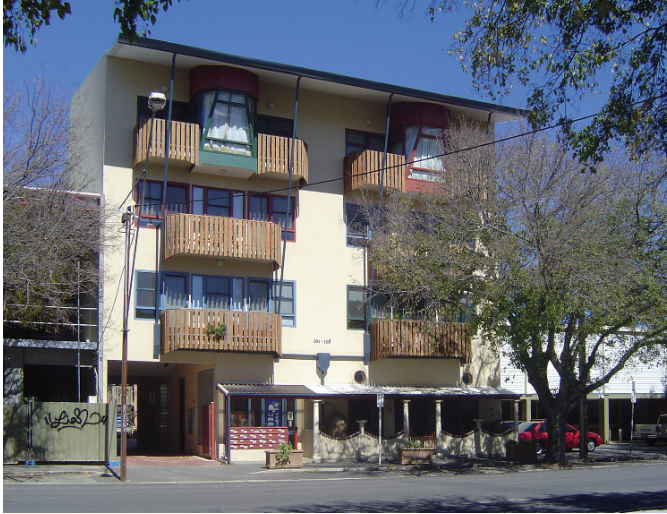
Plate 39: Christie Walk, Adelaide, South Australia The 'stage 3' building on Sturt Street contains 13 apartments plus community facilities on a 16 m × 16 m footprint and carries 5.3 kW of photovoltaics. (© Ecopolis Architects )
