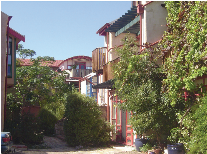
Plate 40: Christie Walk, Adelaide, South Australia Designed for high density with substantial vegetation and a car-free environment. (© Ecopolis Architects )
