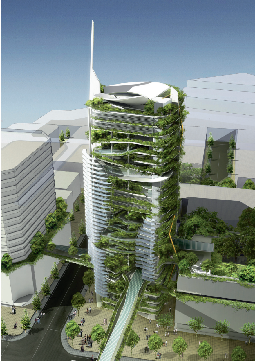
Plate 10: EDITT Tower, Singapore Proposed for an ecologically degraded ‘Zeroculture’ (see Chapter 4) city centre site where the goals according to Yeang’s Ecosystems Hierarchy and Design Strategy have to be to increase biodiversity and organic mass and rehabilitate the ecosystem. The design provides for a surface area of biomass equal to about half the tower’s gross area and uses plant species compatible with the original site’s biodiversity. (© Llewelyn Davies Yeang )
