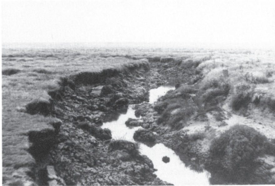
PLATE 3.1 Large borrow pit fronting a sea bank (Gedney Drove End, Wash, UK)
