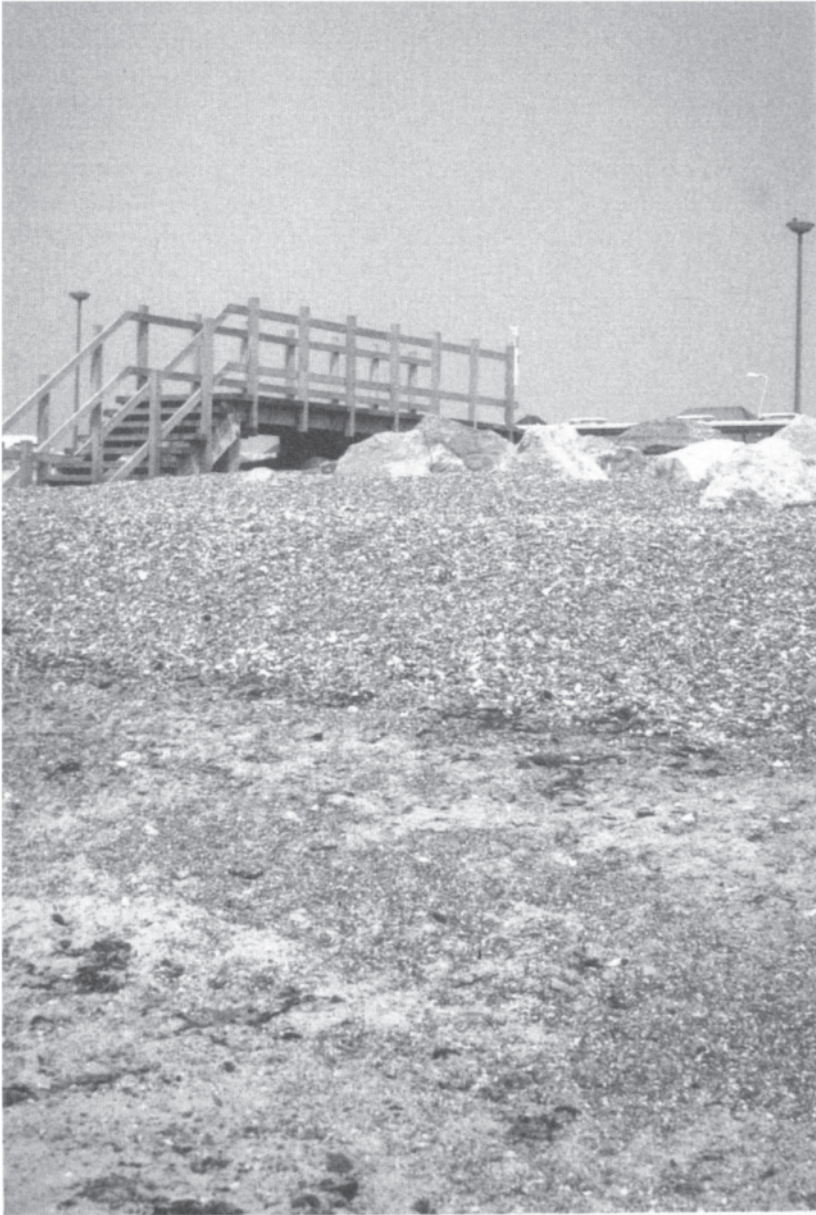
PLATE 5.2 Wooden bridge allowing beach access across large sea defence blocks (Worthing, Sussex, UK)
