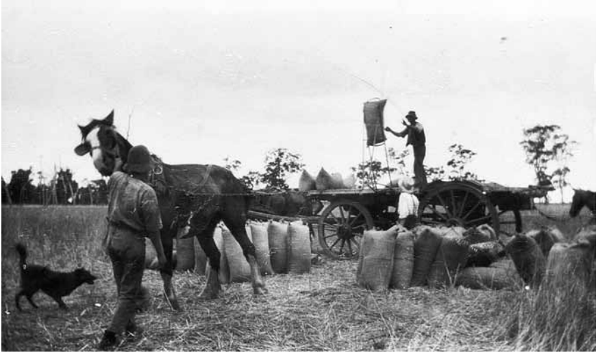
Figure 6.7 Loading wheat at Sunshine farm. Horse on left is pulling base of loader to raise bags – Temora, NSW, c1925
