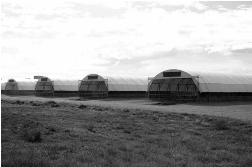
Figure 8.4 Pig shelters at Vertical Pigs
