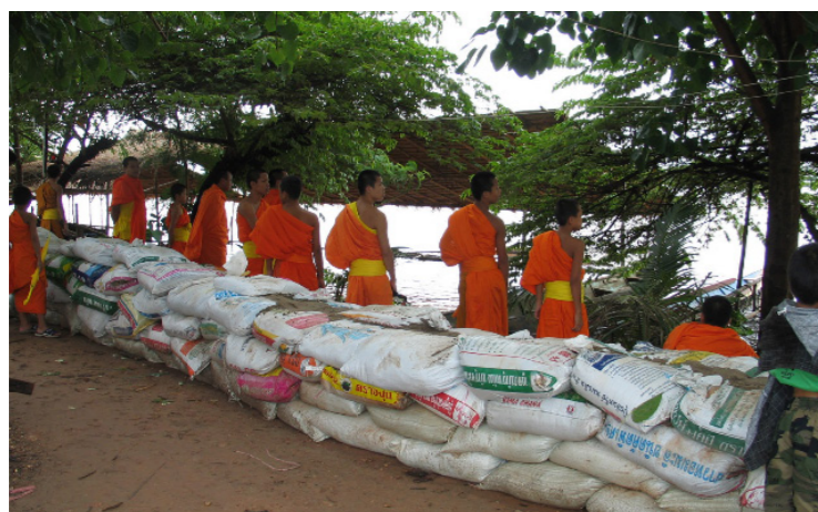
Building sandbanks to avert rising floodwaters in Vientiane, 2008.
