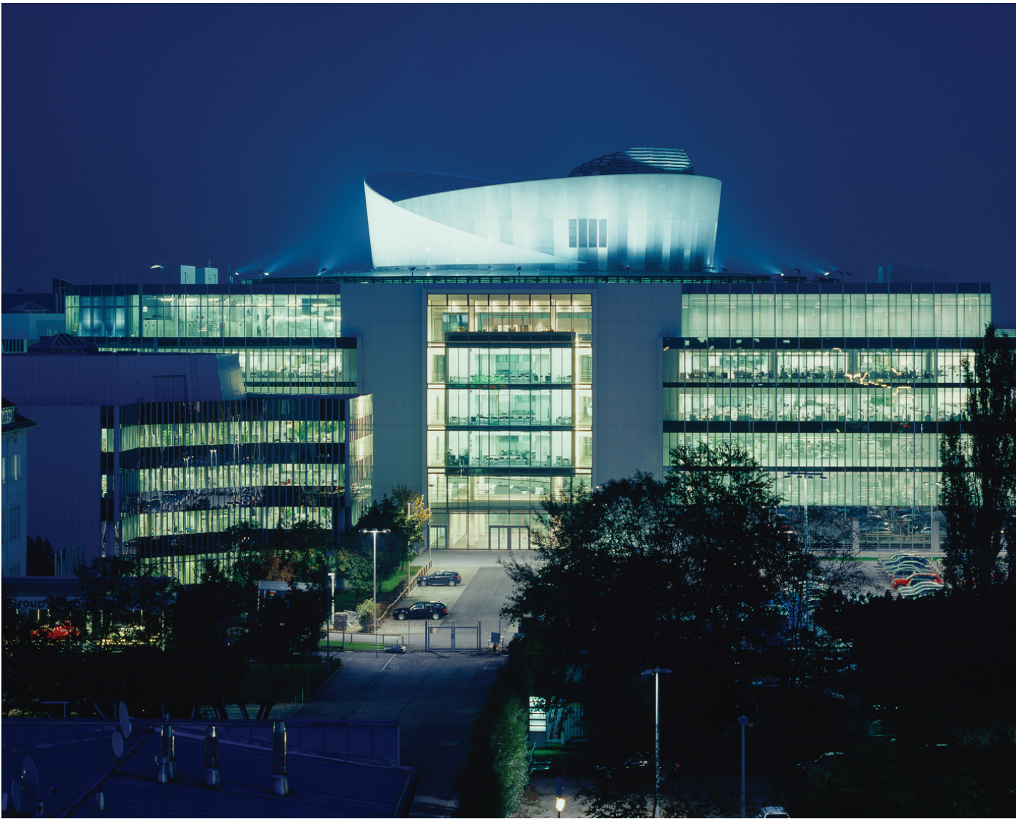
Figure 5-3 In the BMW Projektthaus, departments are located around a center core where most direct project work is done.
