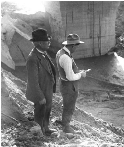
FIGURE 17.2 Mulholland and H. Van Norman, inspecting wreckage at the St. Francis Dam, March 15, 1928. (Photograph courtesy of Santa Clarita Valley Historical Society.)
