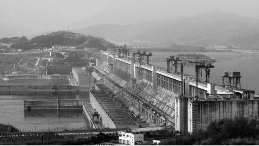
FIGURE 19.3 Completed Three Gorges Dam. (© istock.com/Prill Mediendesign & Fotografie. With permission.)
