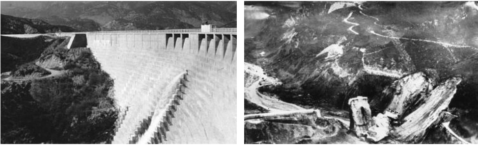
FIGURE 17.1 St. Francis Dam before and after the collapse. (Photographs courtesy of Santa Clarita Valley Historical Society.)
