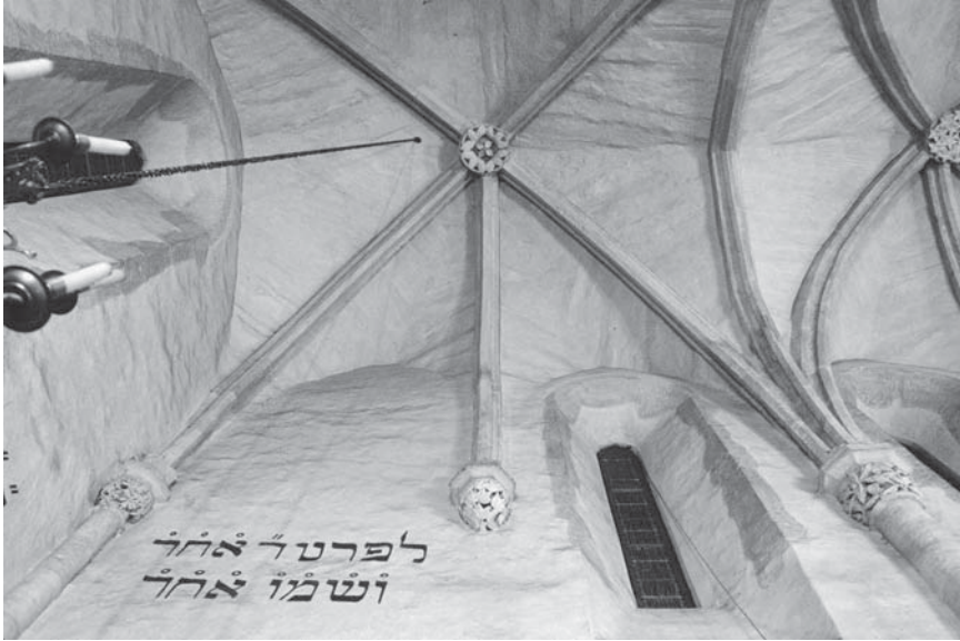
Figure 9.5 Altneschul Synagogue, interior, Prague, Czech Republic, mid-13th century. Erich Lessing / Art Resource, NY.
